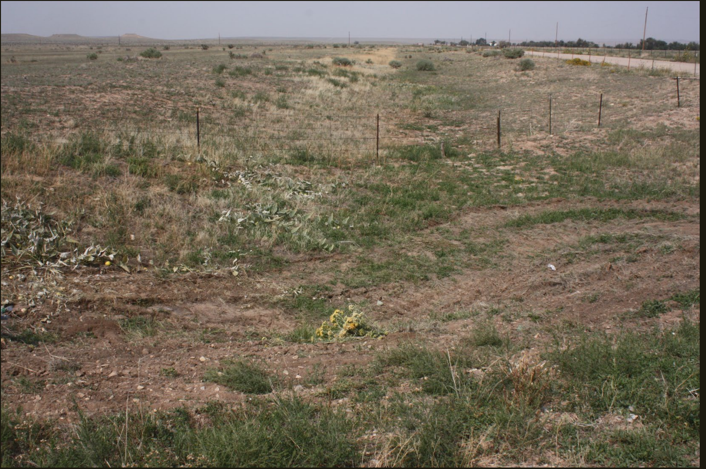
Northward view of the D&RG (1876n) 1,000 feet south of the previous location. Here the grade is in a shallow cut to lower the tracks for a crossing of the Cucharas River, which is a quarter mile south of here (behind the viewer).
