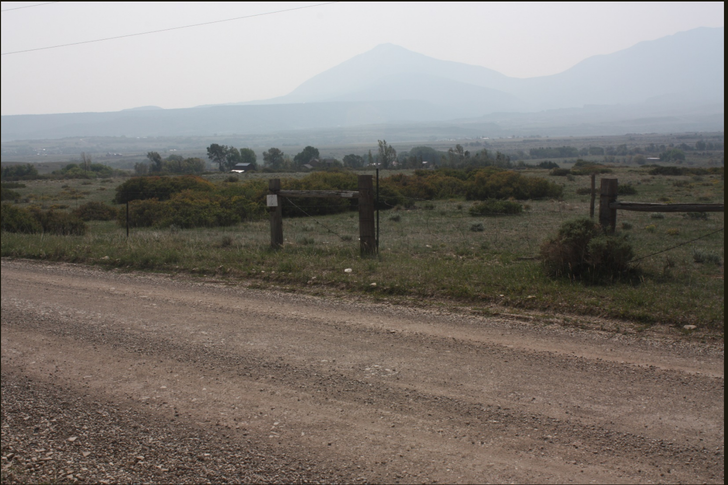
Southeastward view of the D&RG San Juan Extension (1878n), 2 miles west-northwest of the previous location and 1 mile northwest of the point where the original narrow gauge route over the Sangre de Cristo Range (La Veta Pass route) diverges from the alignment of the 1899 standard gauge route (Veta Pass route). The San Juan Extension (1878n), which was abandoned in 1900, ran through this location, but I could find no evidence of the narrow gauge grade in this view or anywhere between here and the standard gauge route (which is 1,500 feet south of this location but is not visible in this view).
