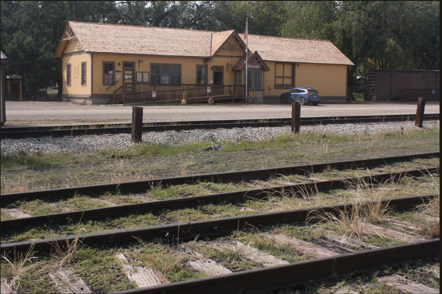
Now we are back at the depot looking south. The farthest track is the D&RG San Juan Extension (1878n) mainline, which at this location was converted to standard gauge in 1894. The next closer track is a siding, the same one with the SL&RG passenger train, which is parked 200 feet to the left (east) of this photo. The closest track is the east branch of a turning wye, which was used to turn helper engines for the climb up to La Veta Pass (for narrow gauge trains) and since 1899 has been used to turn helper engines for the climb up to Veta Pass (for standard gauge trains).
