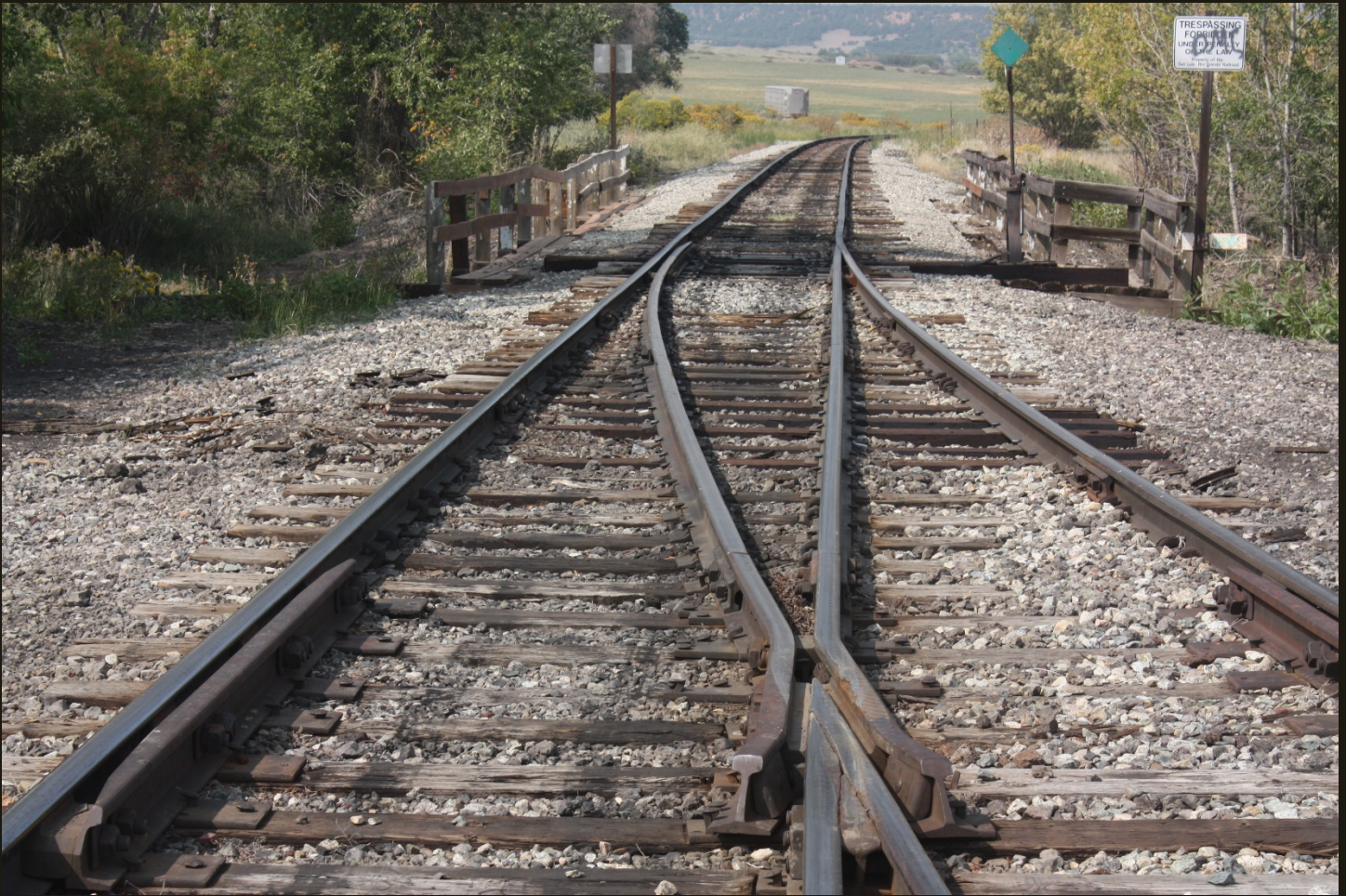
Westward view at the same location as previous, showing the connection of the west branch of the wye (on the right) with the D&RG San Juan Extension (1878n) mainline, which heads out of town after crossing the small bridge over the Cucharas River.
