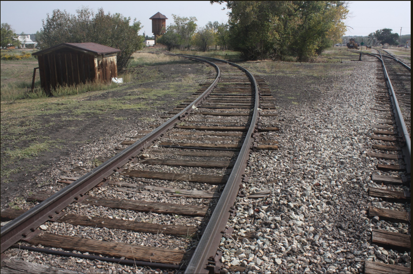
Eastward view a few steps south of the previous location. The track to the left is the west branch of the wye, the track on the right is the D&RG San Juan Extension (1878n) mainline, switch in the upper right connects the mainline to the siding, and the depot is just out of sight to the right of the photo. Note that the west branch of the wye connects directly to the mainline at a switch behind the viewer whereas the east branch connects to the siding (as seen in earlier photos).
