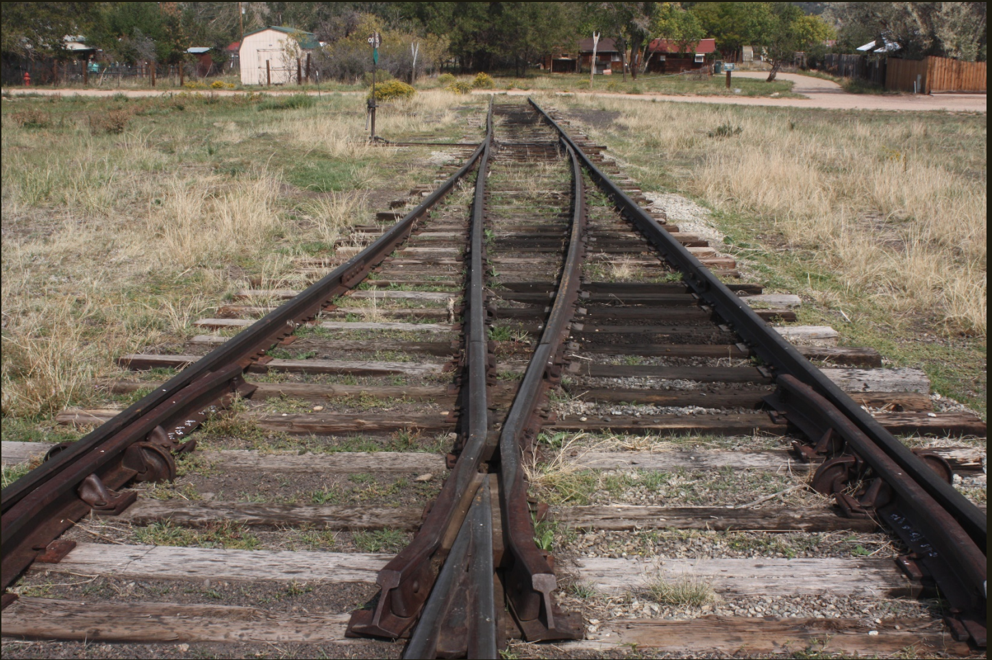
Northward view a few steps north of the previous location at the tip of the wye. There is just enough track beyond the switch to turn a steam engine with and its tender or a diesel engine.
