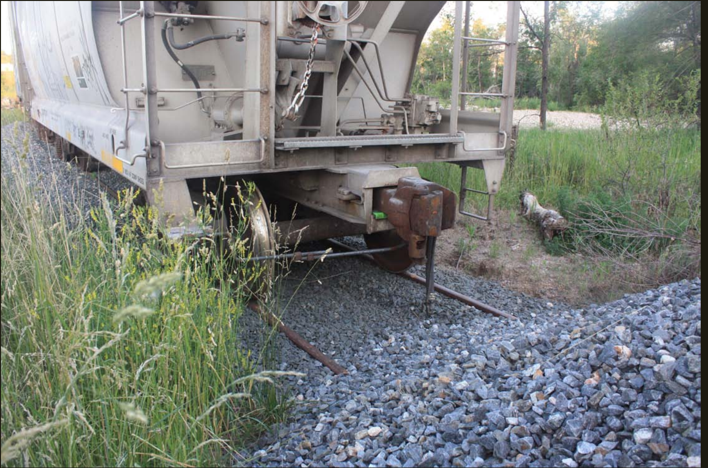
The DU&P (now BNSF) end-of-track at Lyons.
