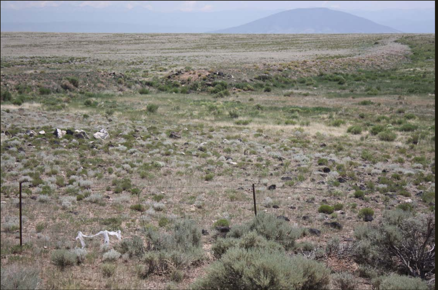
Southeastward view of a breached fill grade on the D&RG Chili Line/Santa Fe Branch just south of the previous location.
