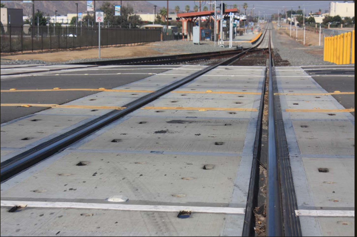
Northward view of the CS/AT&SF, same location as previous and 1.5 miles south of Highgrove. The line on the foreground is the CS (1885). The track on the left is a 1 mile spur, a re-use of a part a former SP branch (which, along with hundreds of miles of connectors, local railroads, and commuter railroads in the LA basin, are not shown on the map). The orange overhang just beyond and to the left of the switch is the Riverside-Hunter Park Metrolink Station.
