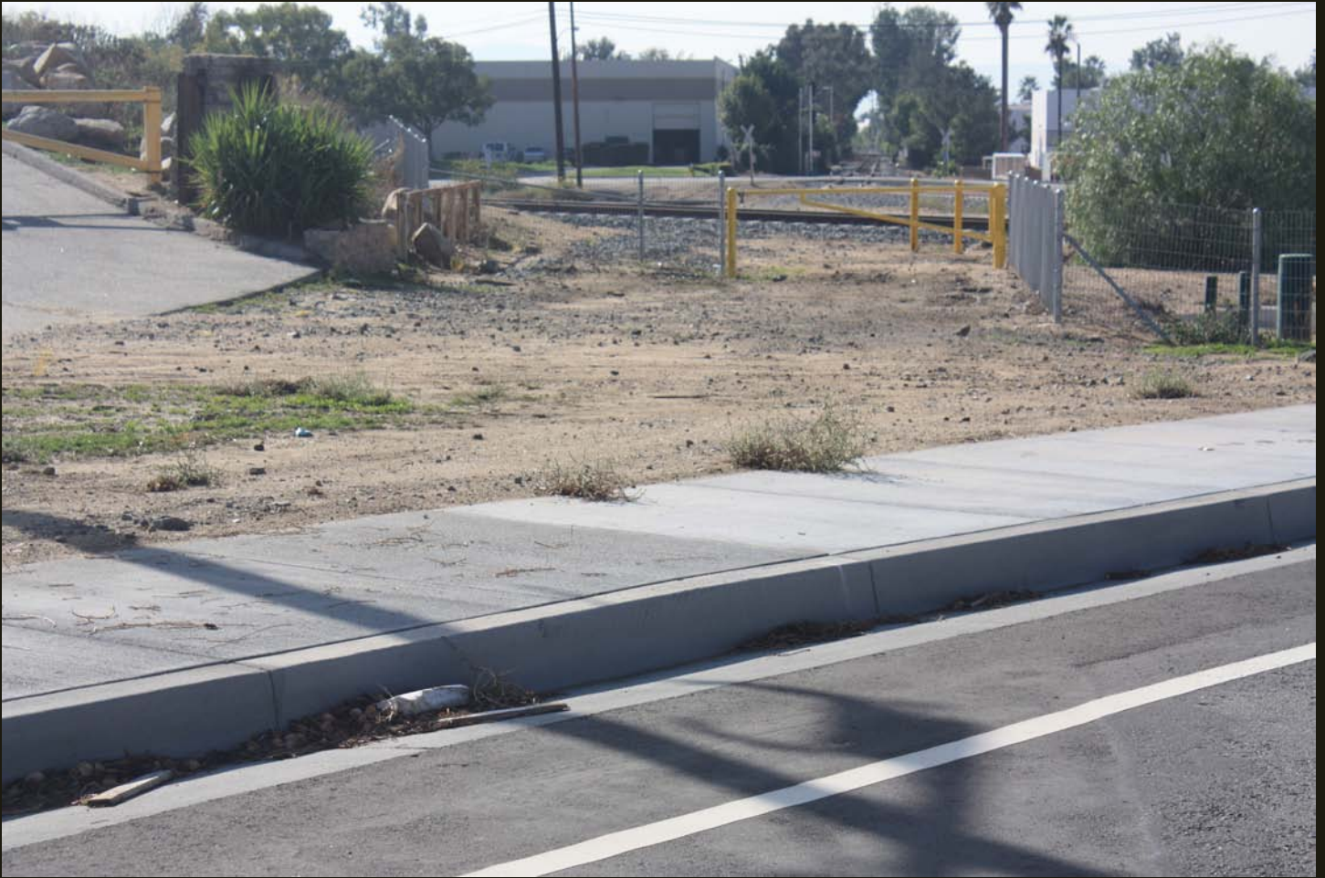
Southwestward view of the CS (1885) line, a few steps east of the previous location. The line just beyond the yellow gate is the CS (1885), with Metrolink concrete ties and welded rail. The SP/PE tracks once extended from the immediate foreground, through the yellow gate, across the then-AT&SF (former CS) tracks, and onto the track alignment visible in the distance just right of center (now an industrial spur). So the straight track in the distance once continued straight toward the viewer, and the curved track that now connects it to the CS alignment (previous photo) was built when the rest of the SP/PE line was abandoned.
