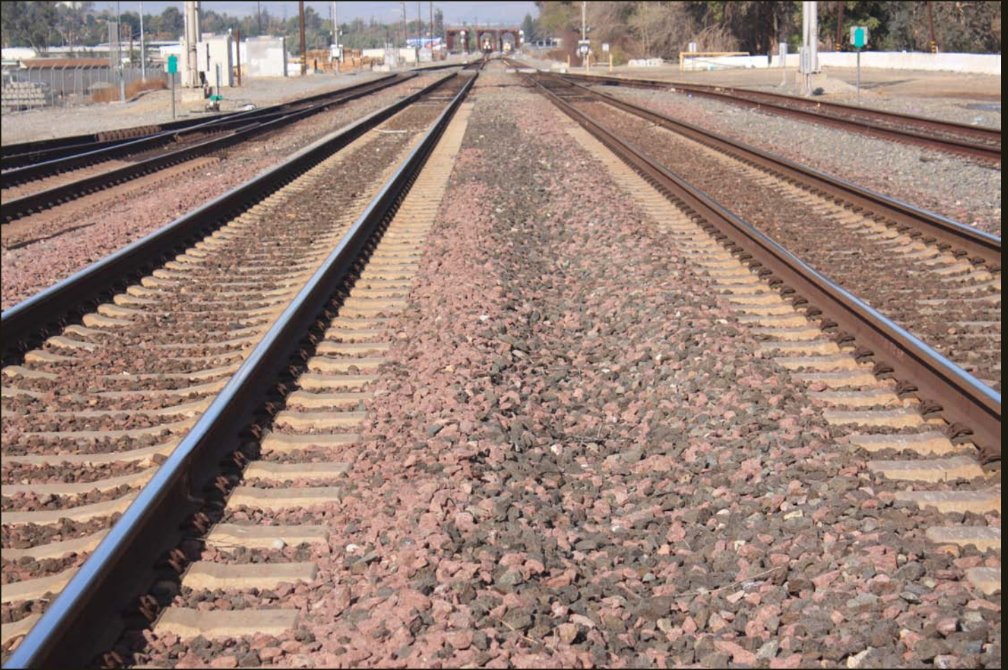
Northward view a few steps west of the previous location. The multiple tracks with concrete ties are on the CS (1885) alignment and the siding on the right connects to the southern continuation of the CS (1885) alignment. The three massive bridges in the distance carry the BNSF Southern Transcon over the I-215 Freeway.
