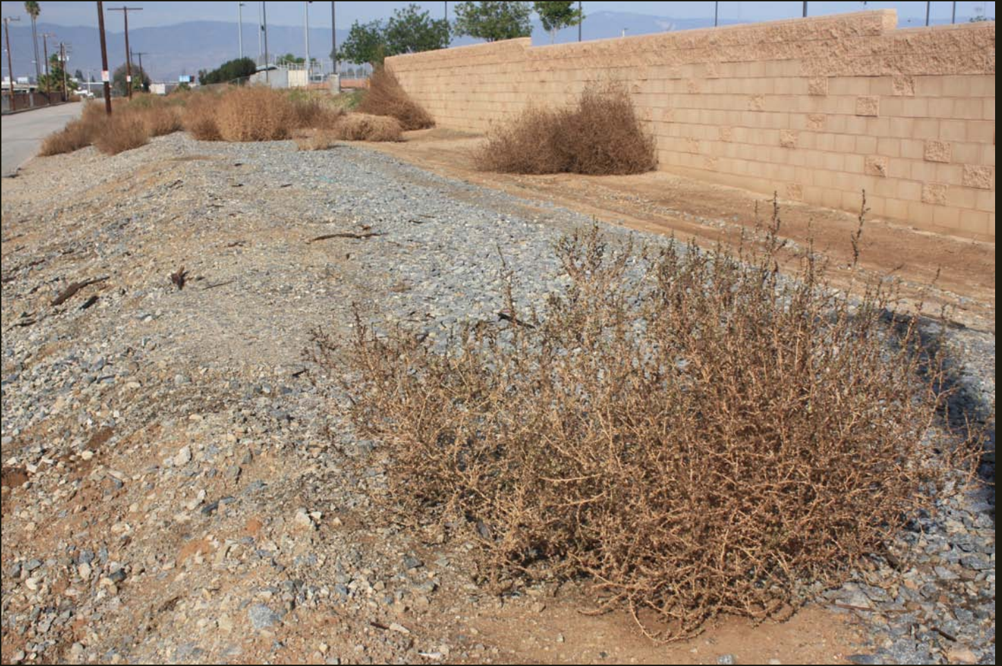
Northward view of the abandoned SP (circa 1900; not shown on map) branch line, in Highgrove 800 feet east of the CS/RSA&LA junction at the previous location.
