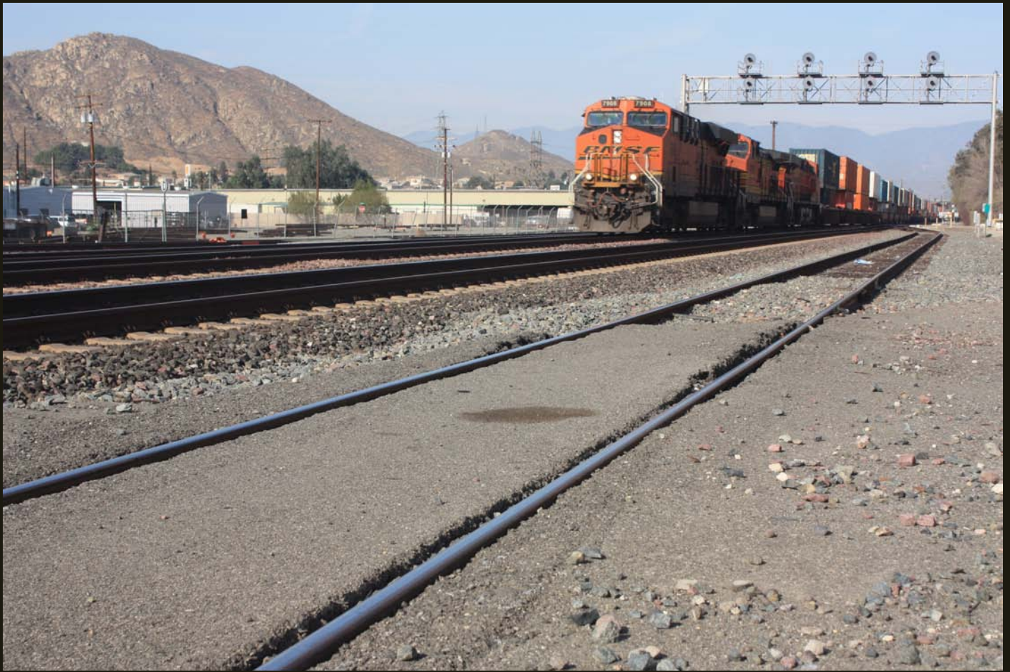
Northward view at the same location as previous in Highgrove. The multiple tracks with concrete ties are on the CS (1885) alignment; the southbound train is approaching the junction with the RSA&LA (1888) to continue on BNSF's Southern Transcon. The siding connects to the southern continuation of the CS (1885) alignment (previous photos).
