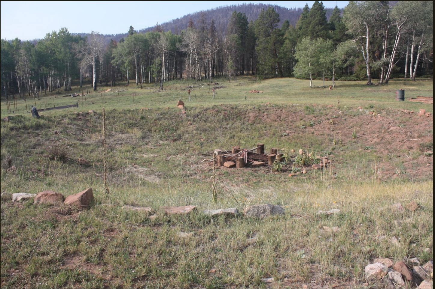
The remains of a turntable used to turn helper engines at the top of the grade. The turntable hardware was moved to the D&RG Crestone Branch (1900n).
