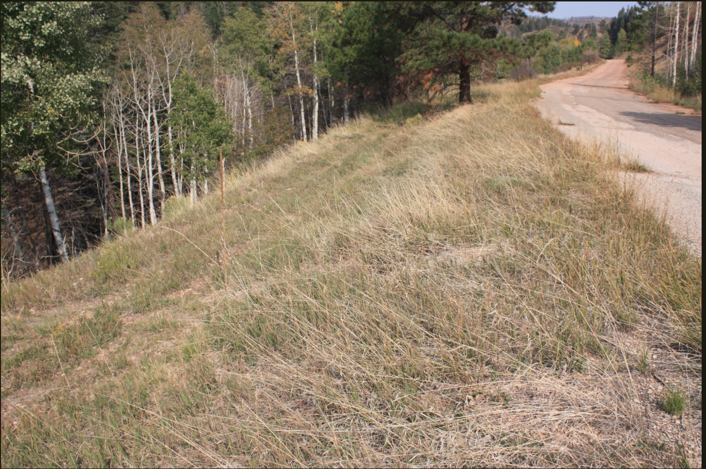
Northwestward view at the same location as previous. The partly overgrown cut grade that runs from the lower left edge of the photo to the Ponderosa Pine in the top center of the photo is the D&RG San Juan Extension (1878n). At the pine tree, the railroad grade merges with the unpaved road from U.S. Highway 160. From that point northwestward, the unpaved road (Forest Road 443) follows the D&RG San Juan Extension (1878n) all the way to La Veta Pass.
