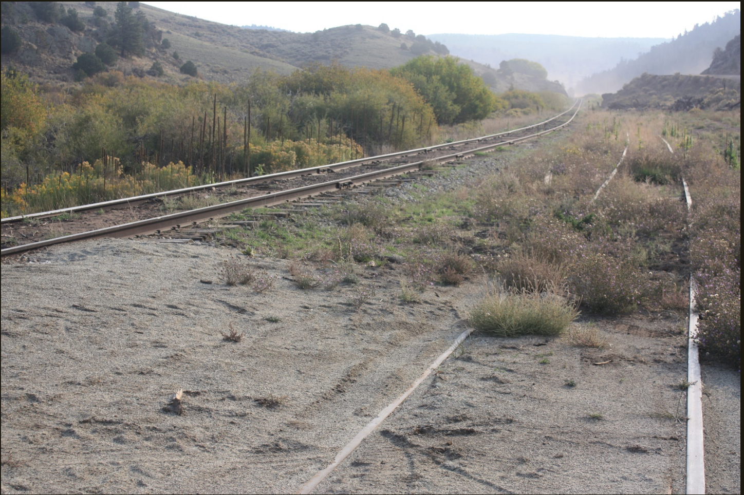
Eastward view of the D&RG San Juan Extension (1899), 2,000 feet east of the previous location and 2.3 miles east of the divergence point with the abandoned narrow gauge route. The bolted mainline is on the left and the partially overgrown siding (the same siding as in the previous photo) is on the right. Access east of here is blocked at a gate for a residential development.
