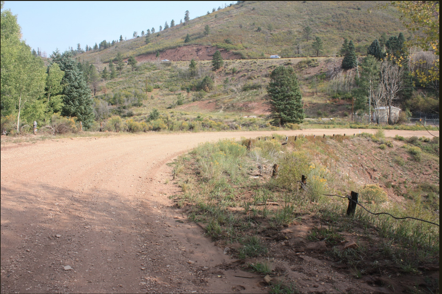
Eastward view of the D&RG San Juan Extension (1878n), now Forest Road 443, 1,300 feet northwest of the previous location. This is the first of two horseshoe bends needed for the climb up to La Veta Pass. This 180-degree curve involved a significant fill grade and a culvert (not visible here) to allow South Abeyta Creek to flow beneath it. The road with cars is U.S. Highway 160.
