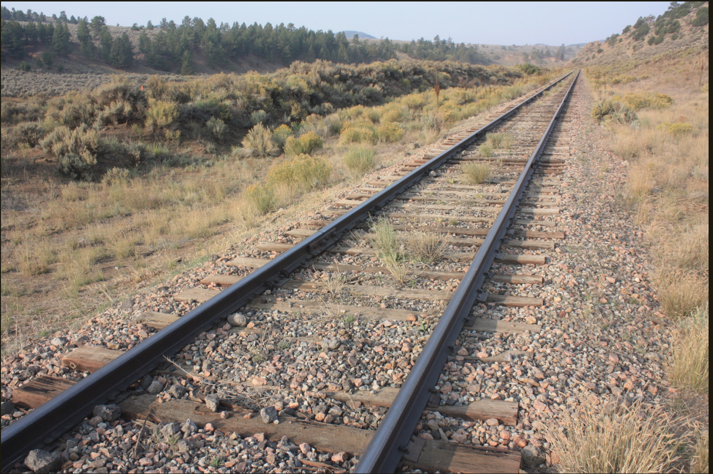
Westward view of the D&RG San Juan Extension (1899) one mile east of the previous location. The abandoned D&RG San Juan Extension (1878n), now U.S. Highway 160, is 3 miles north (to the right) of this location.
