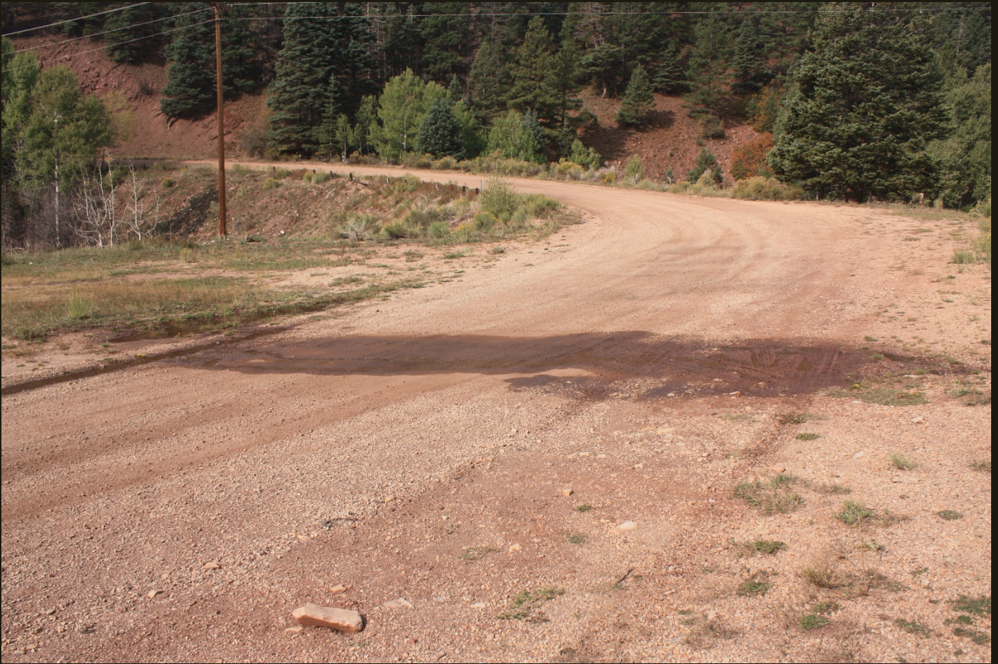
Westward view of the D&RG San Juan Extension (1878n) at the same location as previous. This horseshoe bend changes the alignment from northwestward along South Abeyta Creek to southeastward to climb the slope on the west flank of the creek valley. In this view the grade changes from a fill grade over the creek to a cut grade to negotiate the slope (note the cut exposing red rock in the upper left).
