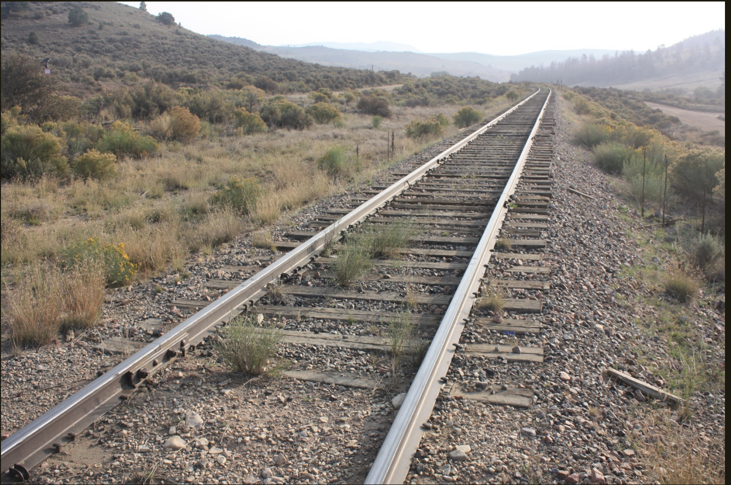
Eastward view of the D&RG San Juan Extension (1899) at the same location as previous. Wagon Creek is out of view to the right (south).
