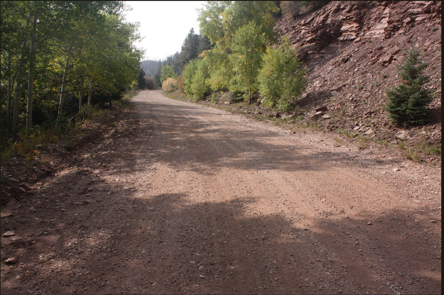
Southward view of the D&RG San Juan Extension (1878n) a few steps west of the previous location, just coming out of the horseshoe bend. Note the cut grade that carries the alignment south-southeastward to climb the slope on the west flank of the valley of South Abeyta Creek. The creek and the lower-elevation portion of the railroad grade (before the horseshoe bend) are parallel to and downslope to the left (east) of this view.
