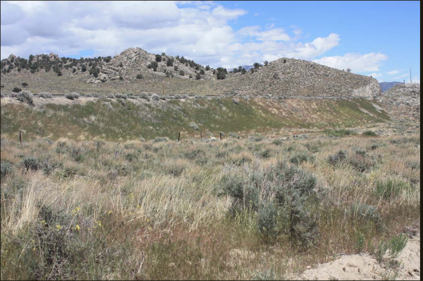
Northward view of the same stretch of the WP (1909) as in the previous photo. Note the high fill grade followed immediately by a cut grade; a lot of earth moving.
