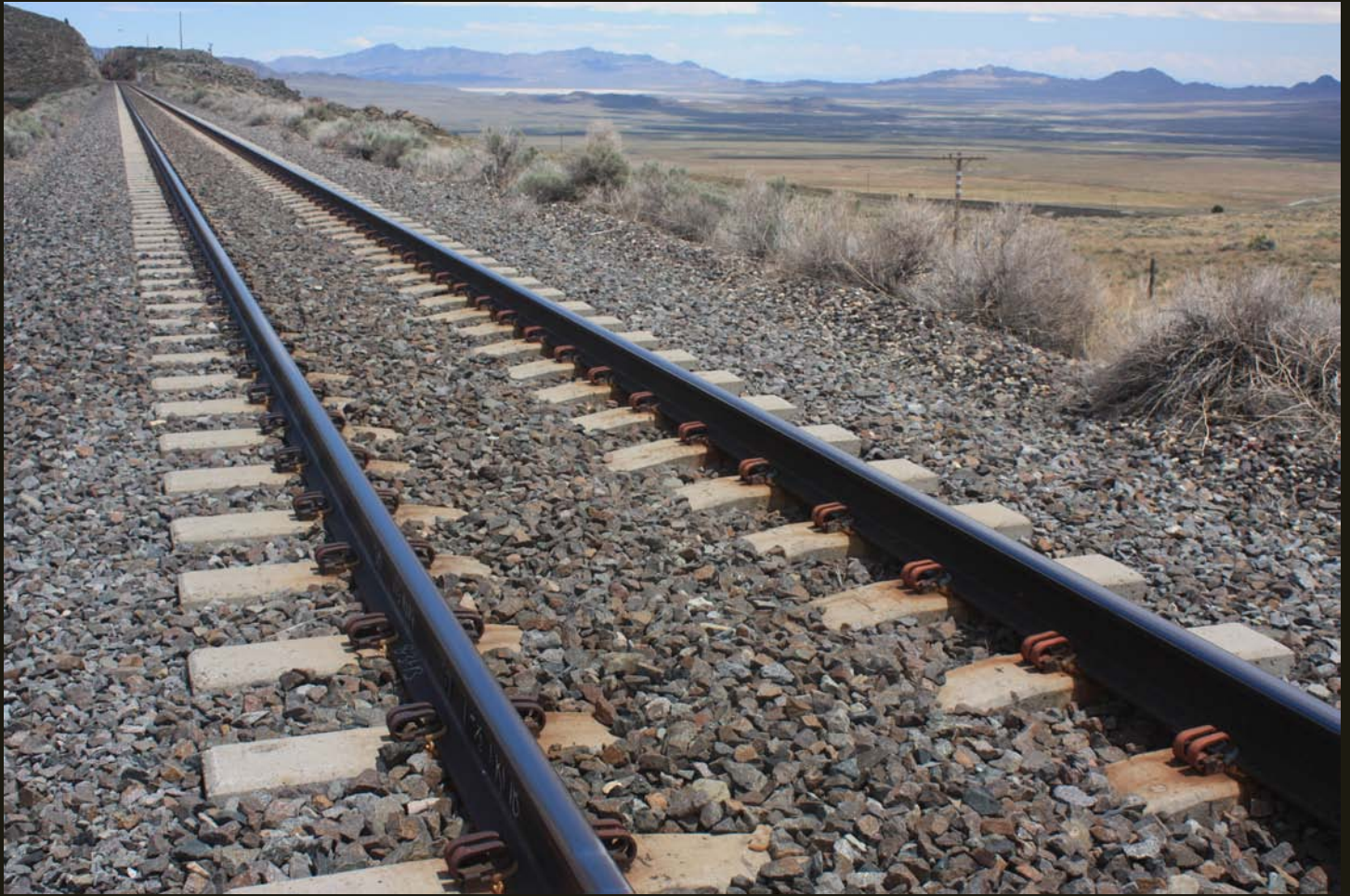
Eastward view of the WP (1909), same location as previous. The drop-off in elevation to Pilot Creek Valley is evident in this view. The dark alignment behind the utility pole is the shadow of the fill grade for the lower arm of the loop.
