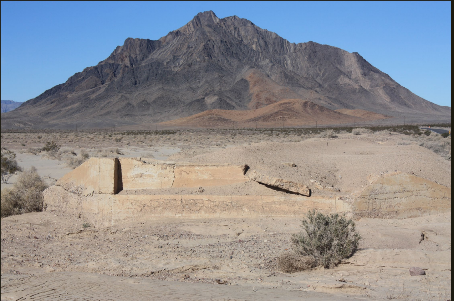
Northward view of a concrete bridge buttress that once carried the T&T over the Amargosa River near a site called Evelyn, 14 miles north of Shoshone. Note the ripple marks in the lower left, formed when the river flowed during a wet winter or a summer monsoon. In the background, 3,800-foot Eagle Mountain is uplifted along a Basin and Range normal fault and consists of Cambrian (half billion years old) limestone and quartzite deposited along what was then the continental shelf of North America.
