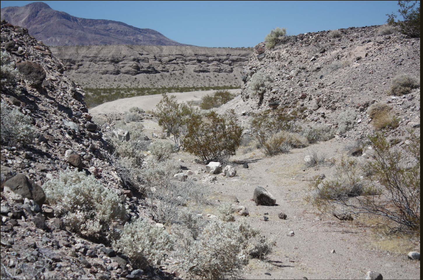
The T&T runs north-south through several fault-bounded valleys of the Basin and Range Geologic Province and across several dry playas. The grade crosses a few low passes, which required some minor cut-and-fill work such as this cut (foreground) and curved fill grade (beyond the cut), located 5 miles north of Shoshone.
