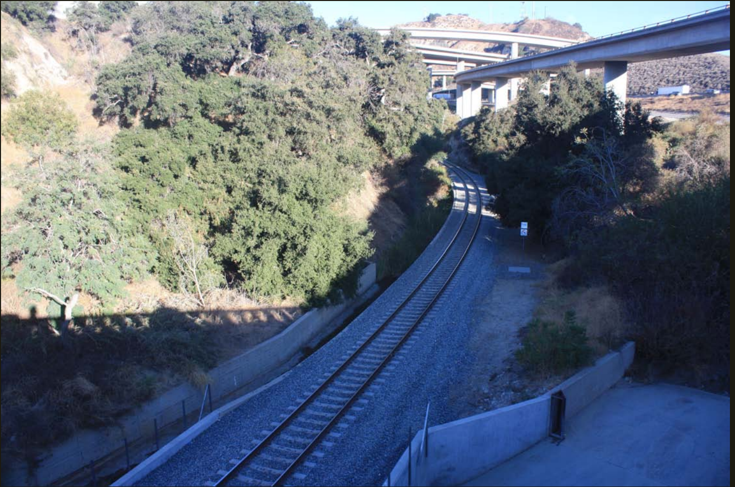
Southern approach to the south end of the 1876 San Fernando Tunnel and the Interstate 5 - State Route 14 Interchange.
