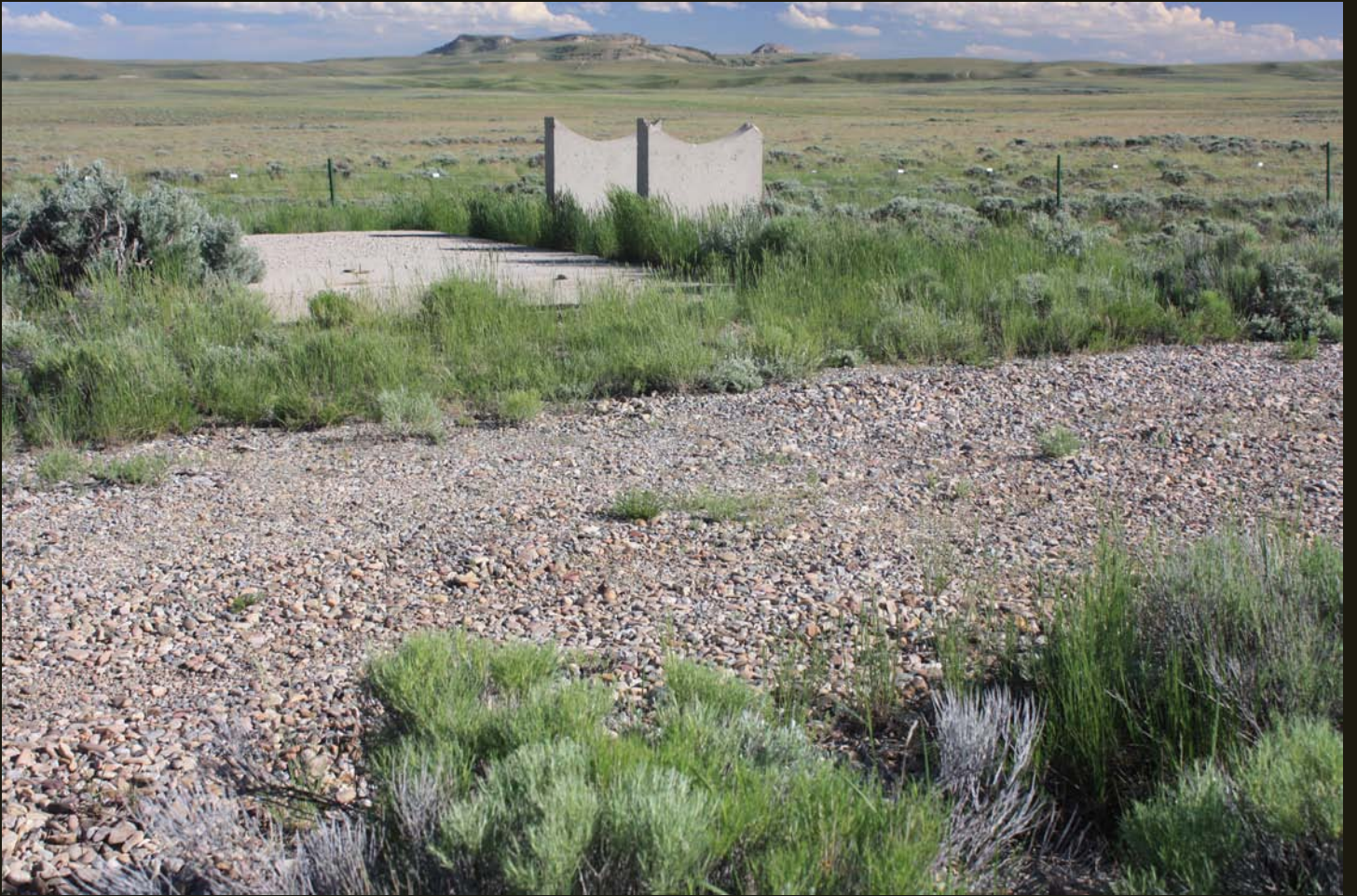
A concrete support structure for some sort of a tank along the grade of the US Steel Atlantic City Railroad at South Pass.
