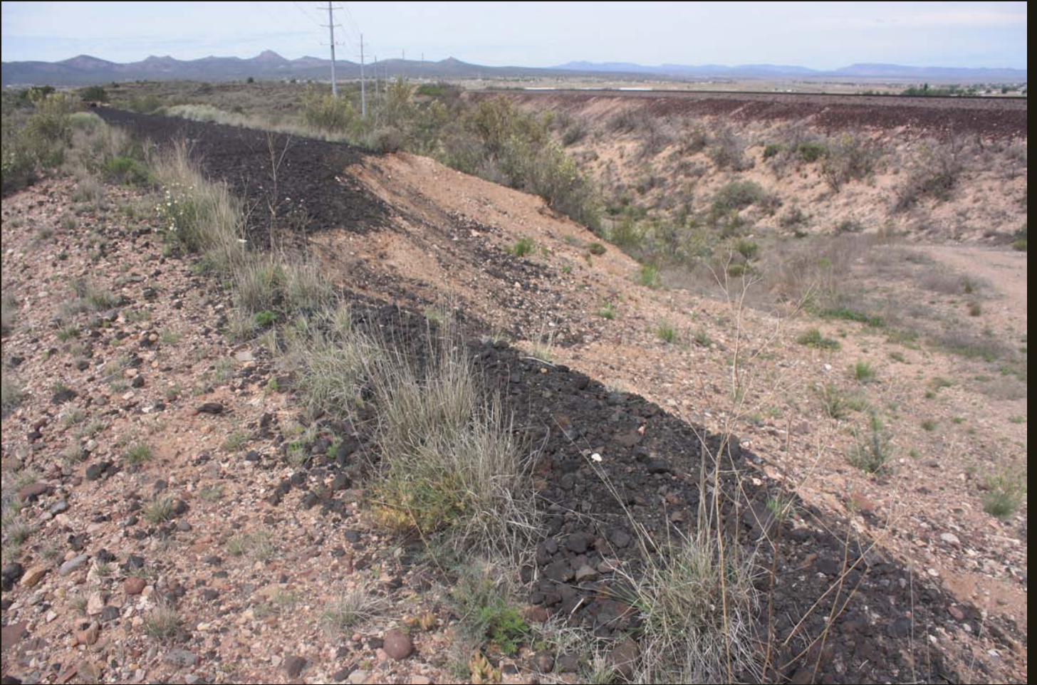
Same location as previous; the black basalt ballast is all that remains of the original SFP&P route that was circumvented in 1962. The welded track to the right is the 1962 grade.
