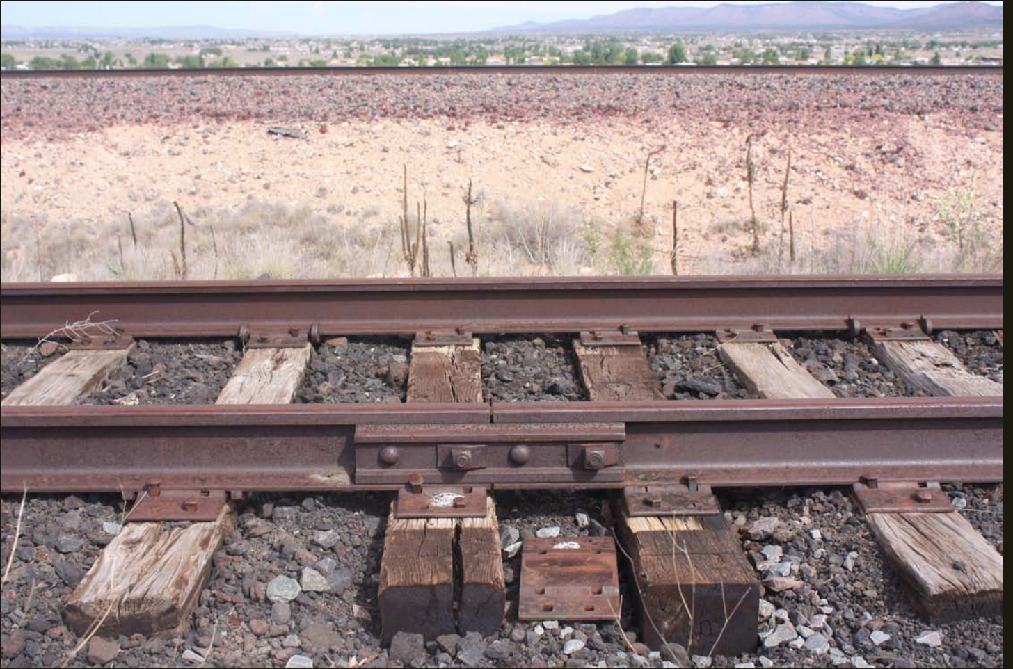
Northward view a few hundred feet west of the previous location. The welded track in the distance is the 1962 grade. The near bolted track is the part of the SFP&P route that was circumvented in 1962.
