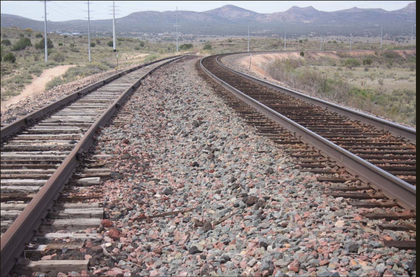
Southwestward view at same location as previous. The welded track that curves to the right (west) is the 1962 grade. The bolted track to the left is the northern end of the SFP&P route that was circumvented in 1962.
