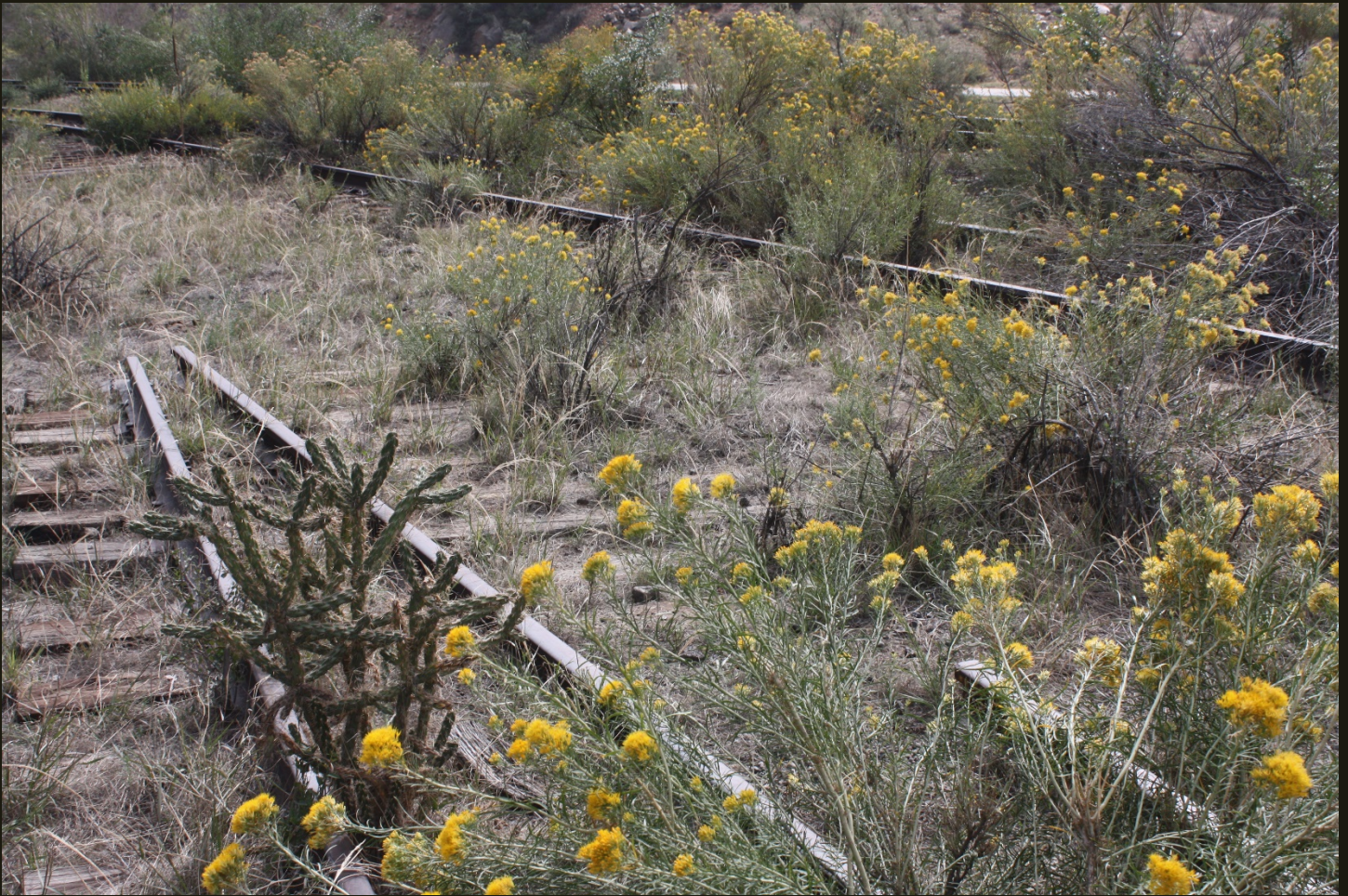
Eastward view a few steps west of the previous location. The D&RG Leadville Branch (1880n) mainline and siding of the previous photo are overgrown with sagebrush. The tracks in the foreground are former sidings that once connected to the main siding at the former switch noted in the previous photo; the long ties for that switch are barely visible in the upper left.
