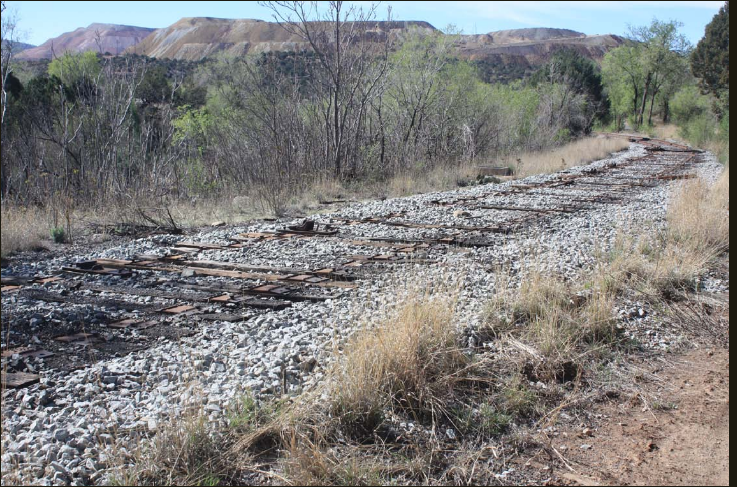
Missing rails just south of Hanover.
