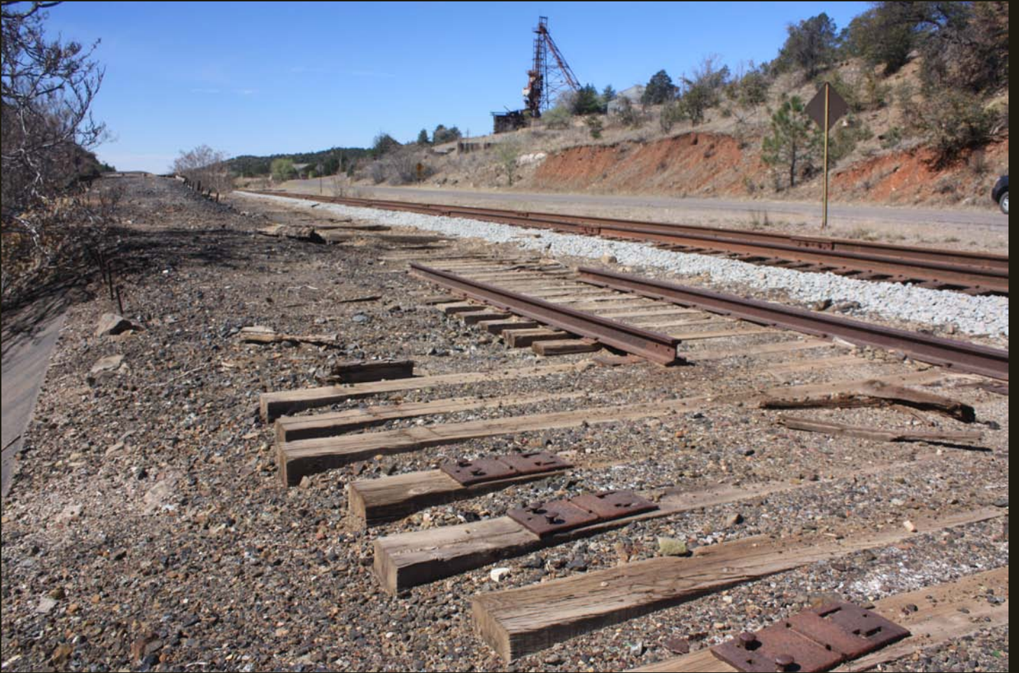
Abandoned loading facility on the SC&N at Hanover, with abandoned mine headworks in the distance.
