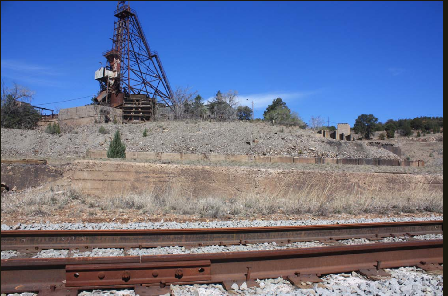
The SC&N line and Hanover abandoned mine headworks.
