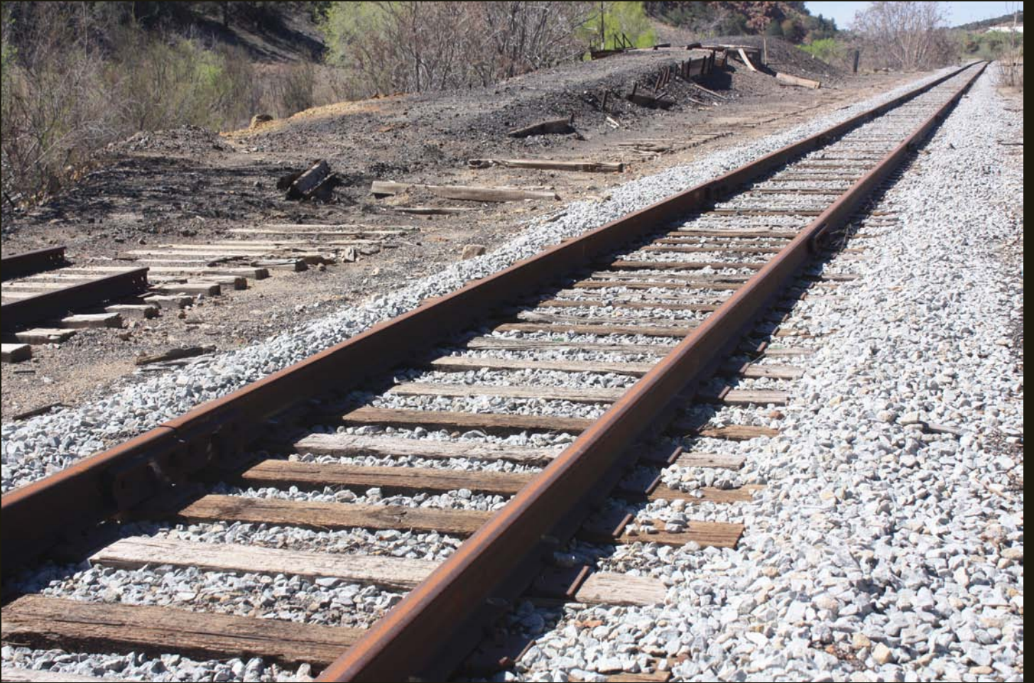
An abandoned loading facility on the SC&N at Hanover.
