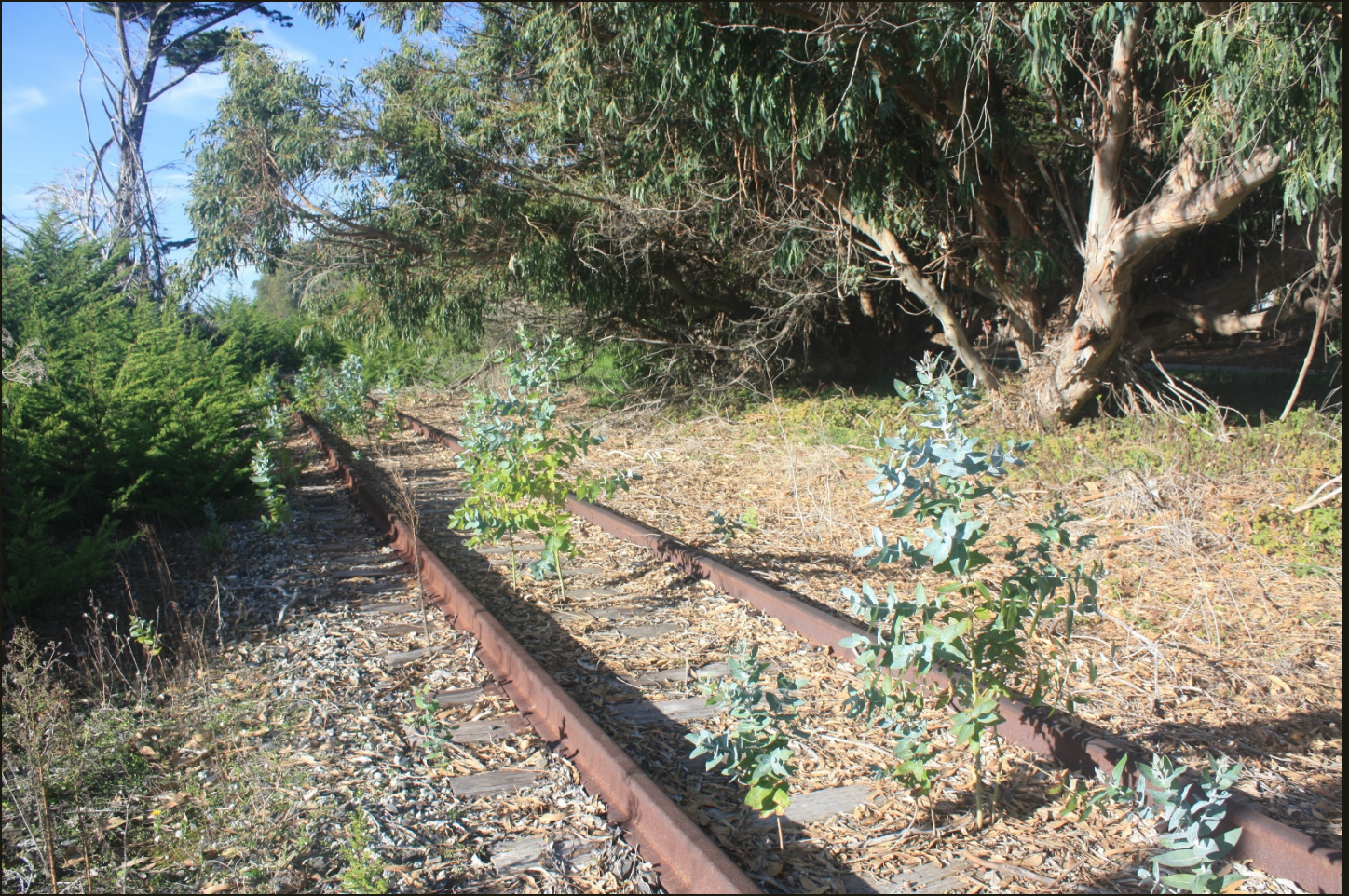
Northward view, same location as previous. The track ends under the brush; the track was removed north from here 4 miles to the original end-of-track at Swanton.
