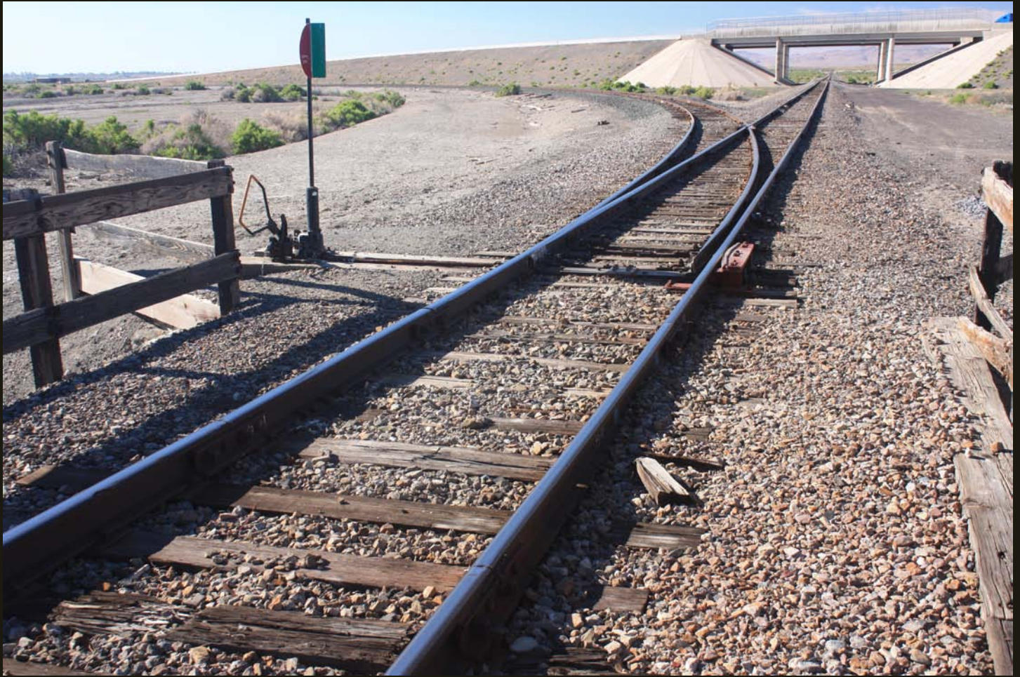
Southeastward view of the same small bridge and switch as in the previous photo. The N&C Hazen Cutoff (1905) is in the foreground and continues straight under the U.S. Highway Alt 50 overpass and the N&C Fallon Branch (1907) goes off to the left (southeast). The small bridge is for Hazen Drain, which drains agricultural fields west of this location.
