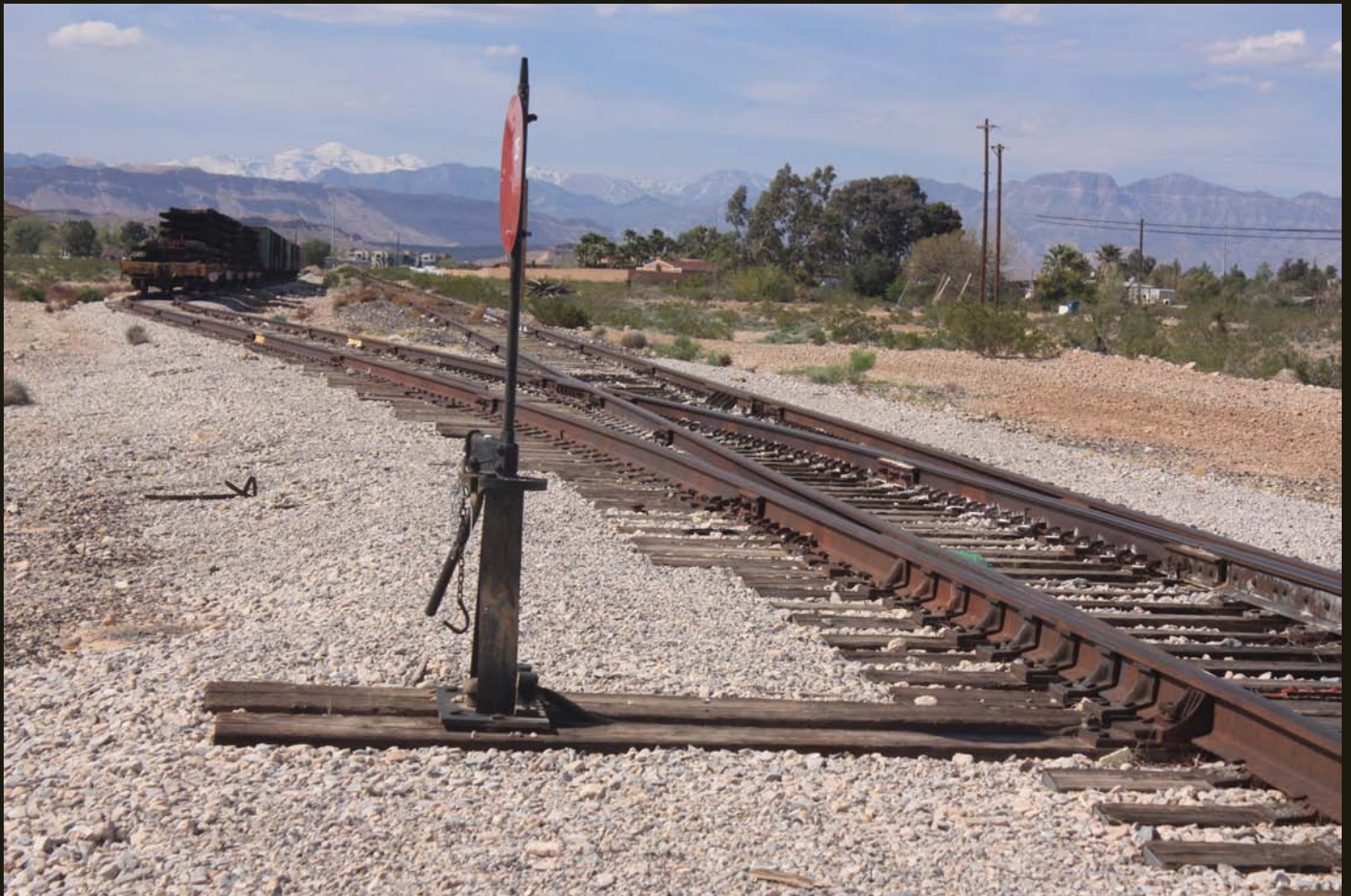
Westward view of the LA&SL Blue Diamond Branch (1923), same location as previous. A siding splits off the line and is used for car storage. The 11,000-foot Spring Mountains are visible in the distance; Blue Diamond and the gypsum deposits are in the foothills.
