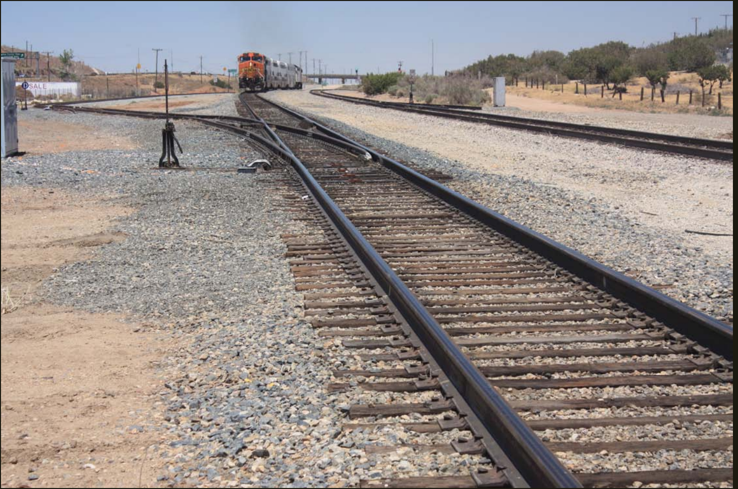
Sidings at Soledad Pass, adjacent to Vincent Hill Station. Note overpass in the distance, which is the grade summit.
