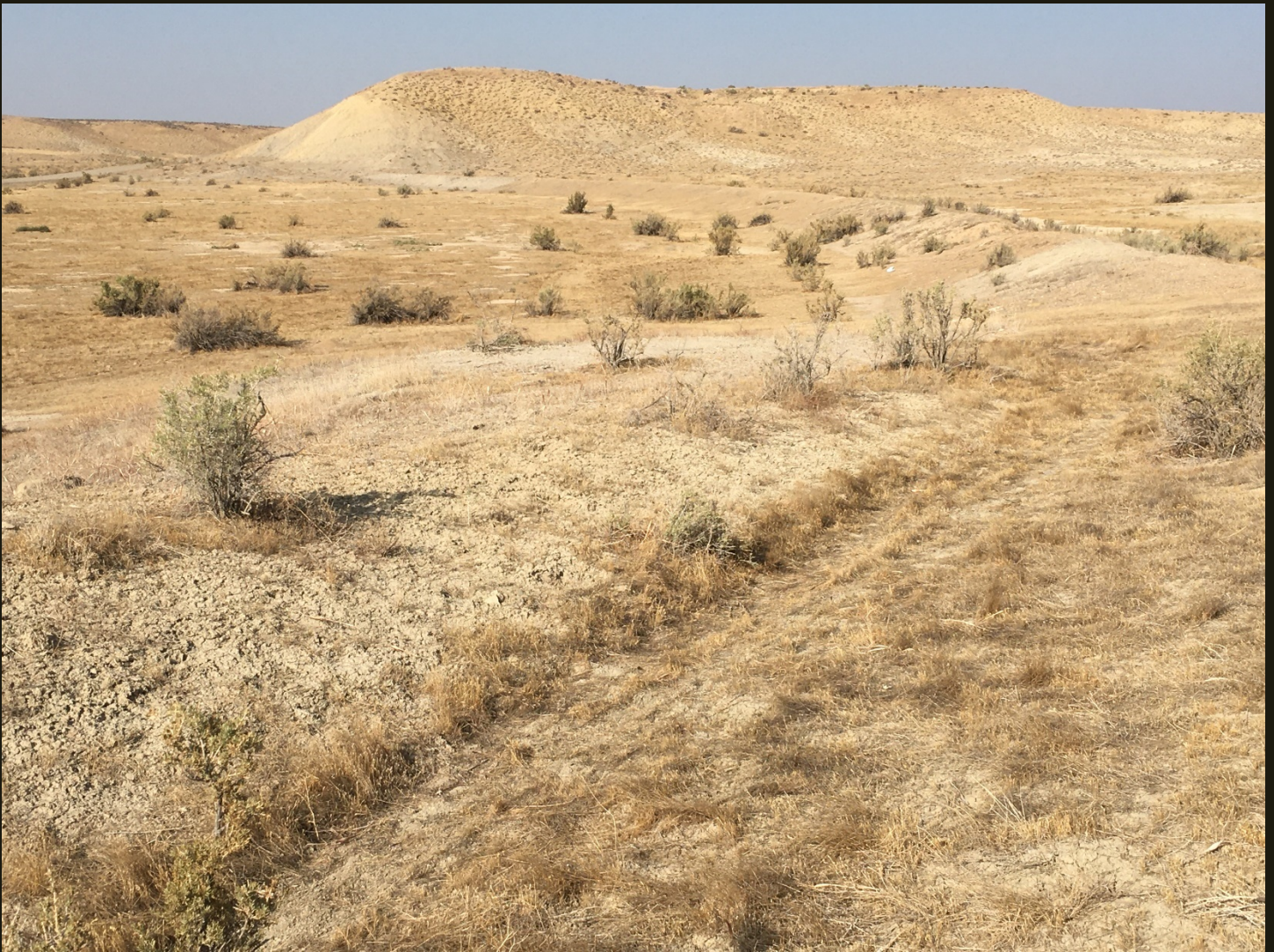
Westward view of the D&RGW (1883n) in Utah, 2.5 miles west of the previous location (which is in Colorado). The significant fill grade here is well preserved. Old U.S. Highway 6/50 is visible in the upper left where it crossed the railroad alignment.
