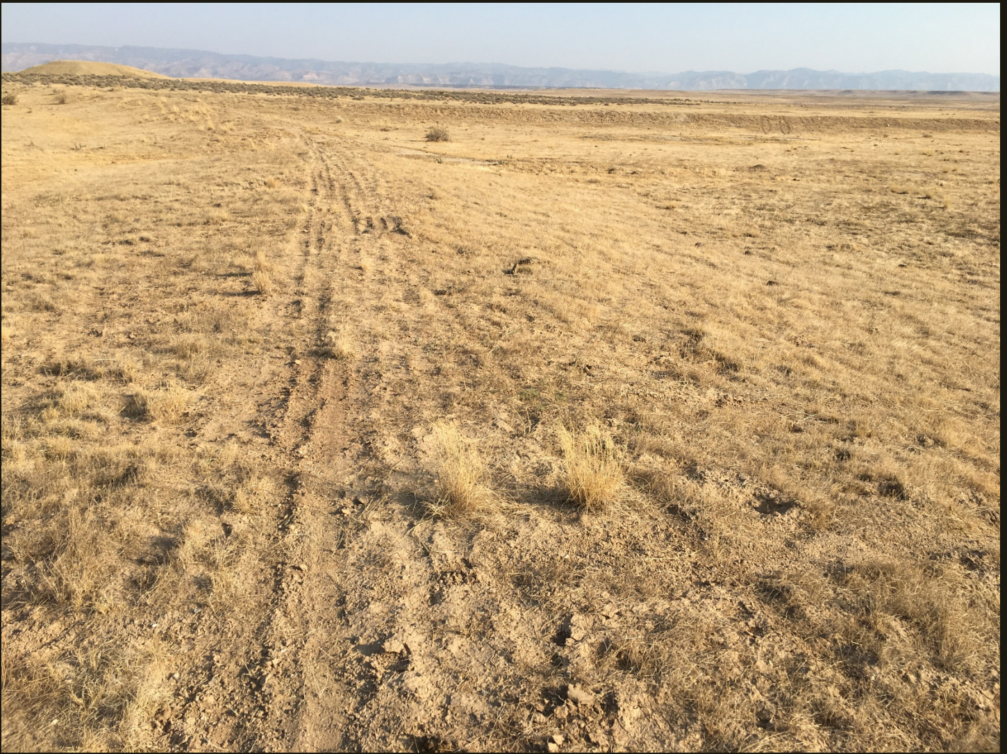
Northward view of the southwest branch of the wye, 200 feet south of the previous location. The tip of the wye is in the far left corner and the northeast branch of the wye runs across the width of the photo in the distance.
