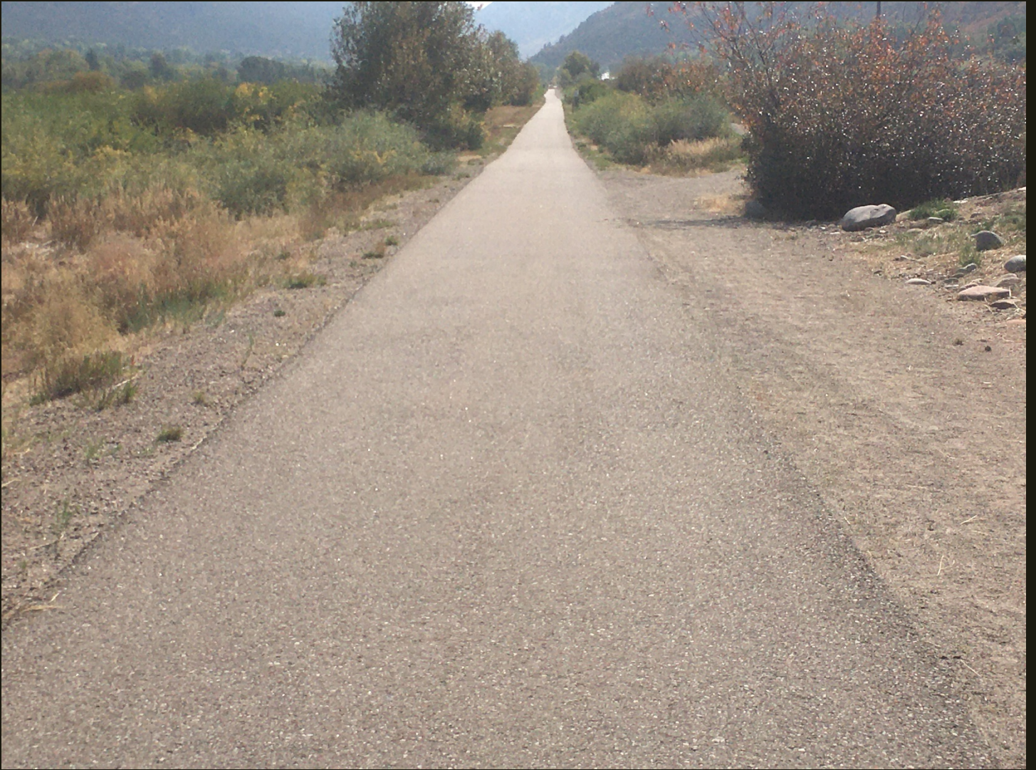
Southeastward view of the D&RG Aspen Branch (1887n) at the same location as previous.
