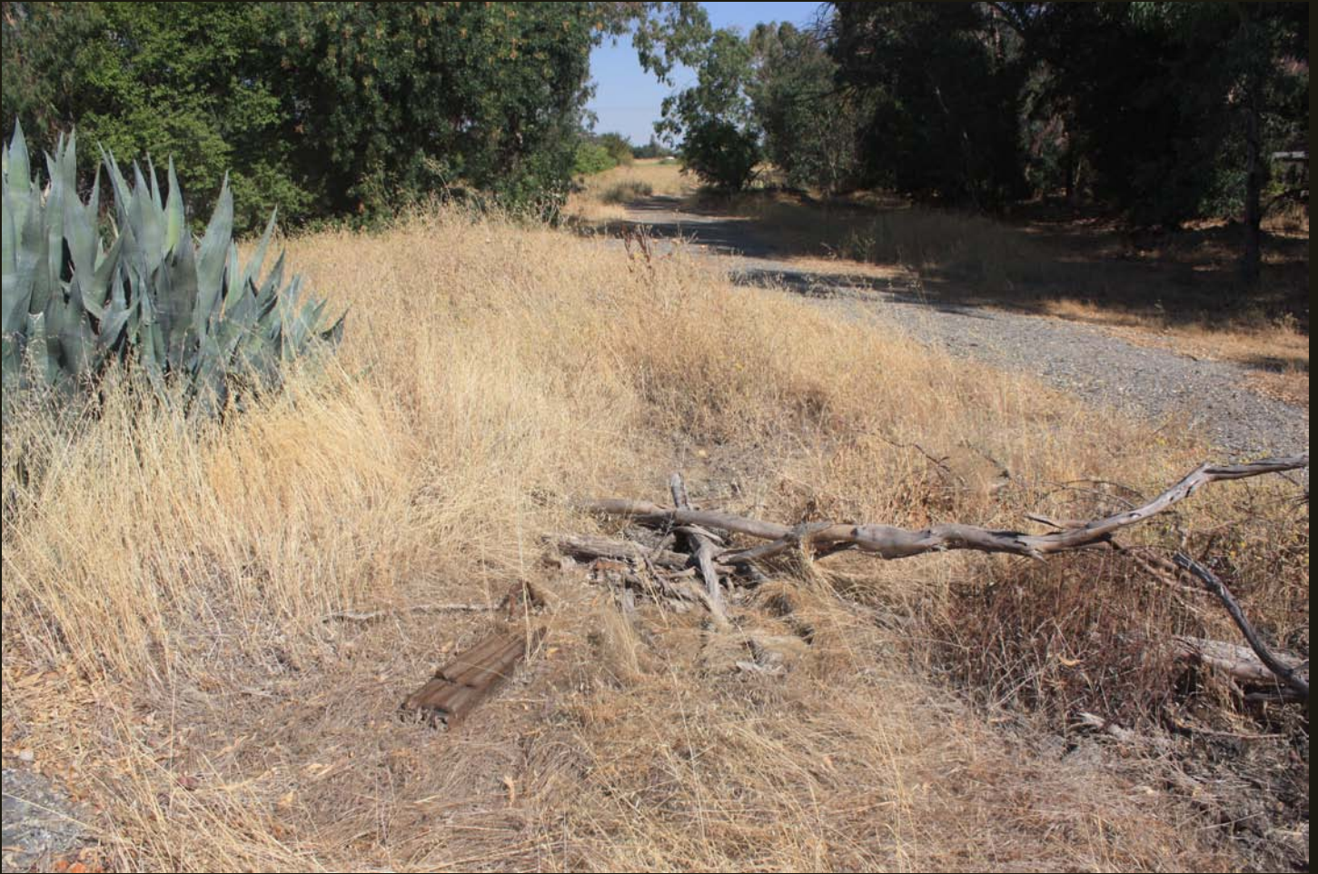
The gravel grade in partial shadow in the upper right of the photo is the abandoned northern leg of the former wye for the Hamilton Branch at Wyo. Note the curve to the right in this northward view, which once carried the east-west Hamilton Branch into alignment with the north-south Northern Railway.
