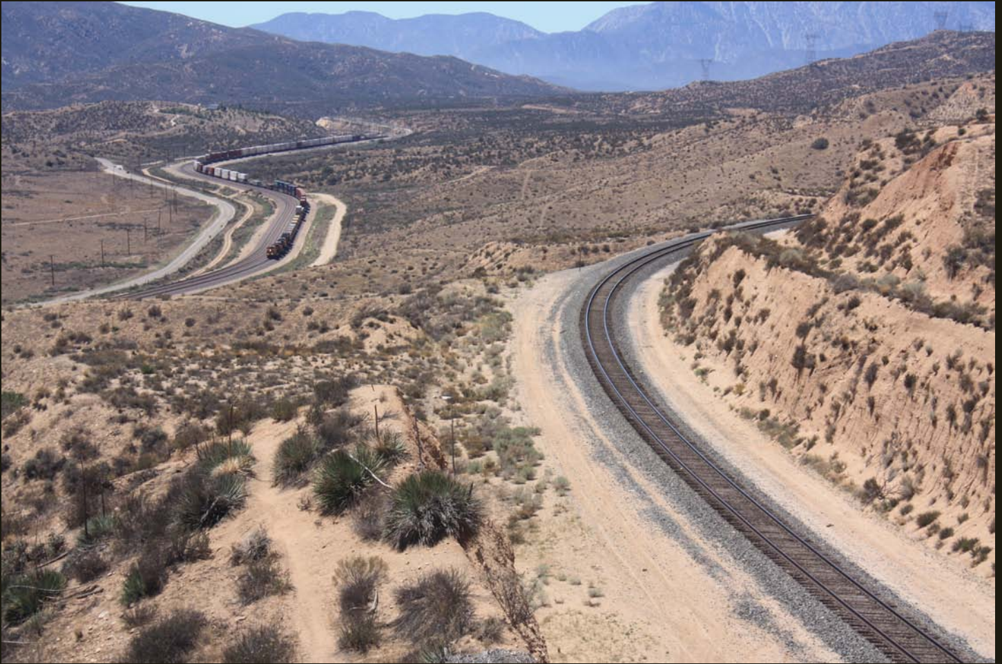
Southwestward view of same area as the previous few photos, with the BNSF triple train in Summit Valley and, in the right (northwest) foreground, the 1967 SP Palmdale Cutoff comes in at a higher elevation than Cajon Pass, located at the rear of the train. Note that the 1967 SP cut is in soft alluvium.
