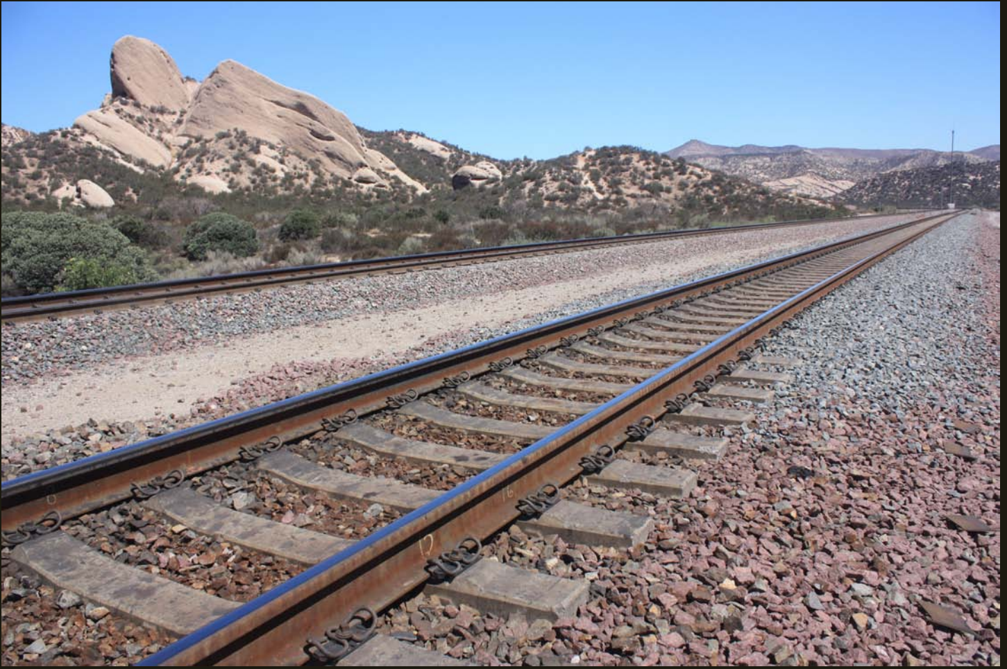
The 1913 AT&SF route passes through the Mormon Rocks, which are Miocene-aged (18-20 million years) gravelly sandstone that has been folded and tilted during movement of the nearby San Andreas fault. The second track was added in 2008.
