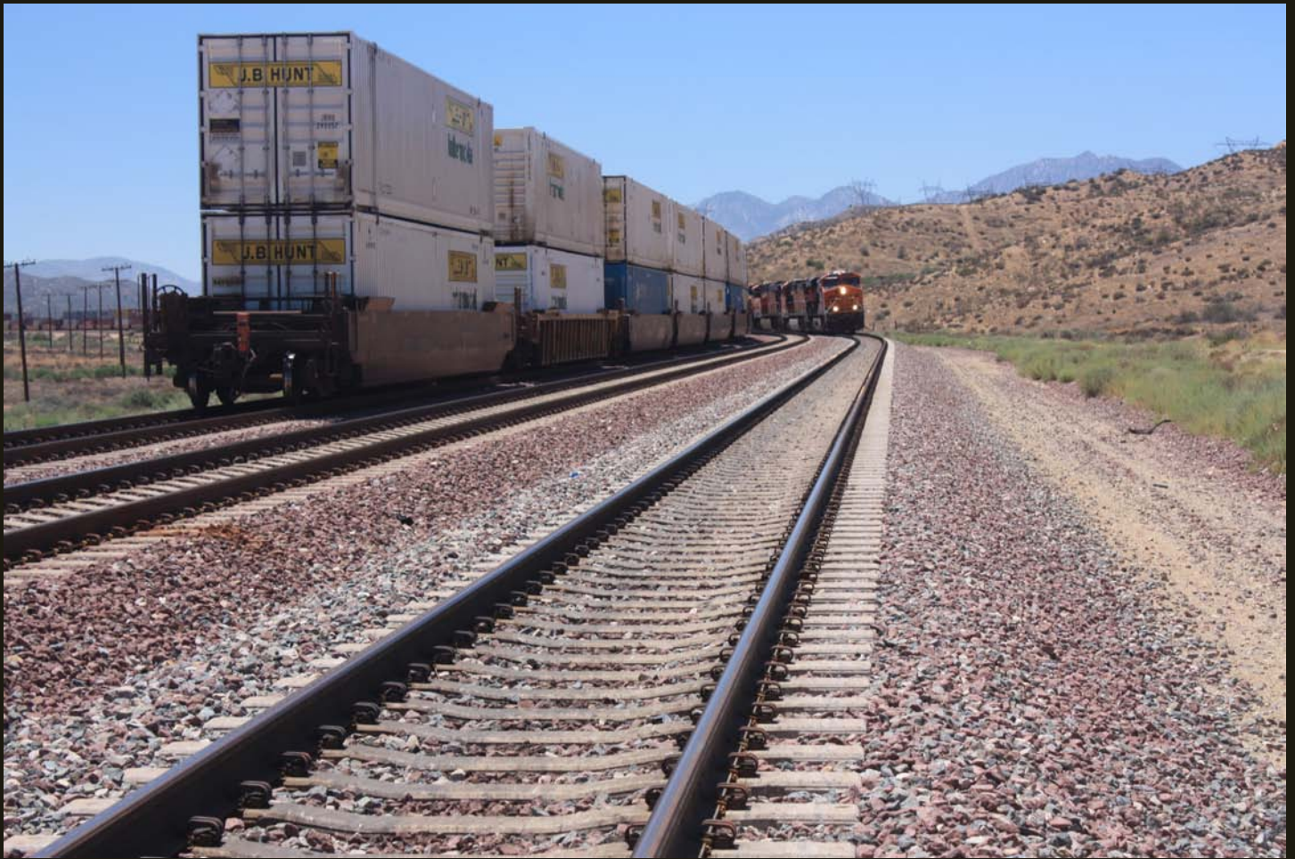
Closer view of the BNSF triple track, at about the same location as the previous photo. The CS first built through here in 1885, the AT&SF added a second track in 1913, and BNSF added a third track in 2008. The SP Palmdale Cutoff is upslope and out of view on the right (north) in this southwestward view in Summit Valley.
