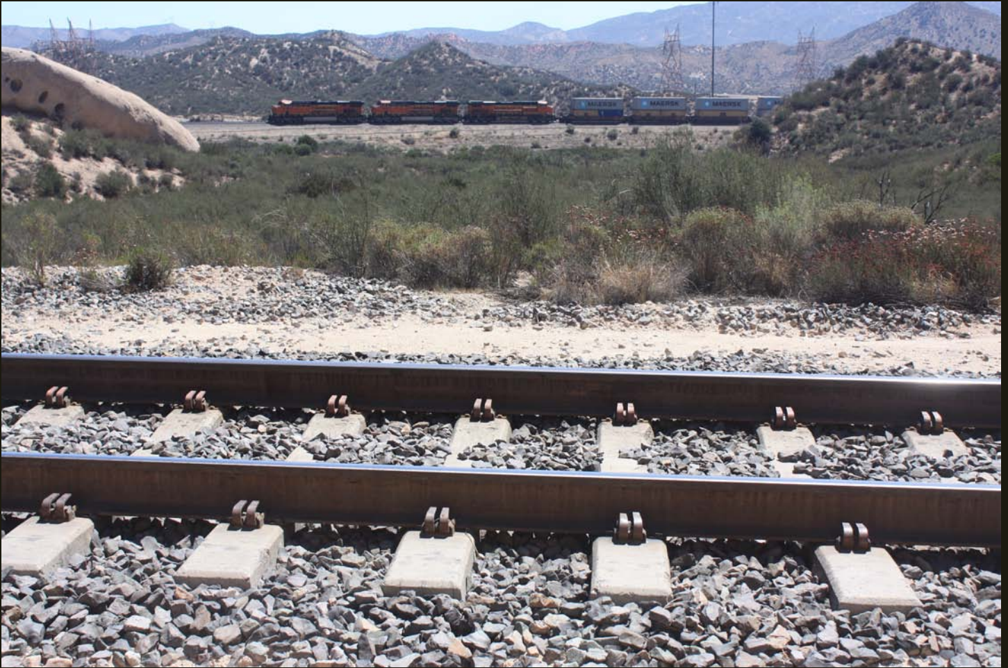
In this eastward view 8 miles southwest of the Cajon Pass at Mormon Rocks, the 1967 SP Palmdale Cutoff is in the foreground and the AT&SF mainline (1913 grade) is plied by a BNSF container train. The 1885 CS grade is out of site a half mile farther east and lower on the slope.
