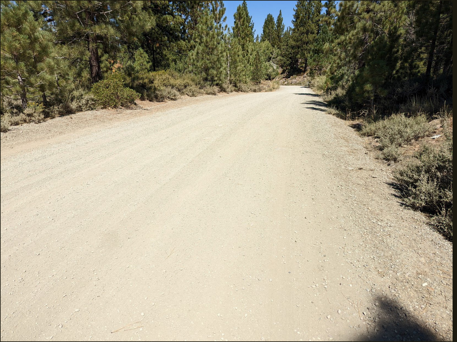
Northward view (toward Loyaltan) of the B&L (1901), now Smithneck Road, at the same location as previous.
