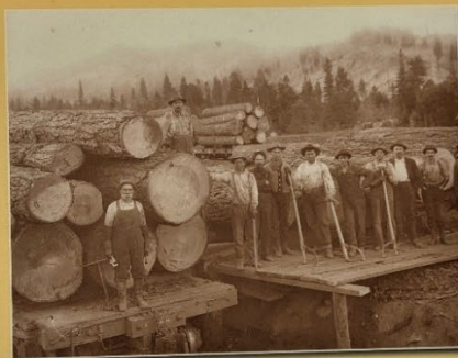
Crew with peavy hooks used for transferring logs to rail cars.
