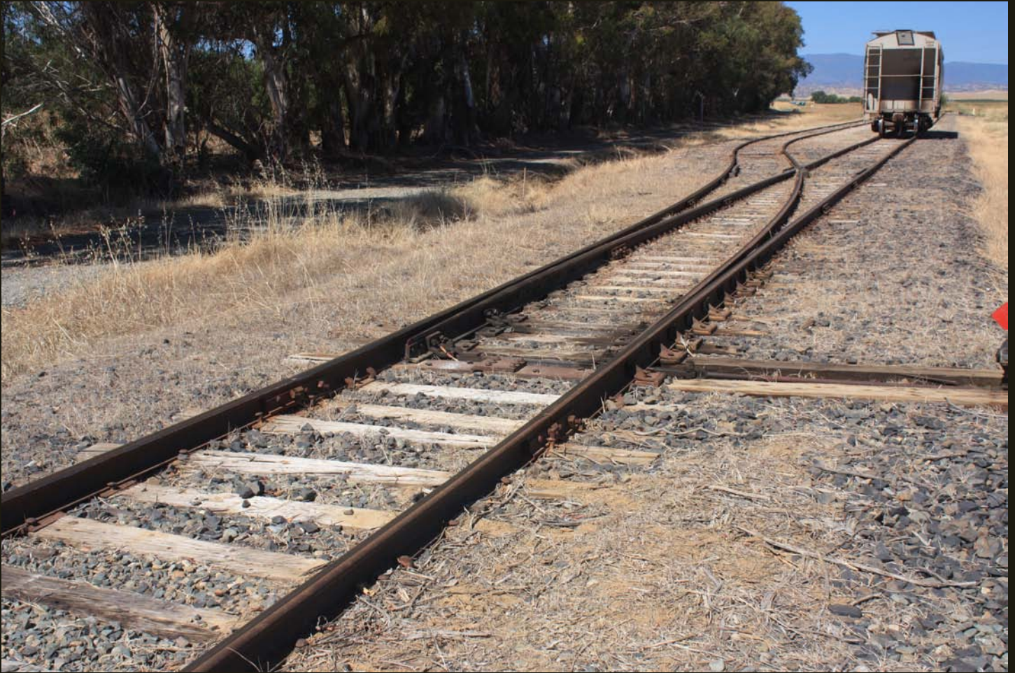
Westward view of the WS&M 2 miles west of Willows near the end-of-track. The gravel road to the left (south) of the track is the original WS&M grade. The existing tracks leave this grade just behind the viewer, and the tracks shown here to access the Johns-Manville Fiberglass Plant were likely laid in 1951, when the line west of here was abandoned. Note the curve to the right just beyond the siding; the end-of-track and plant access are 100 yards north (to the right) of that curve.
