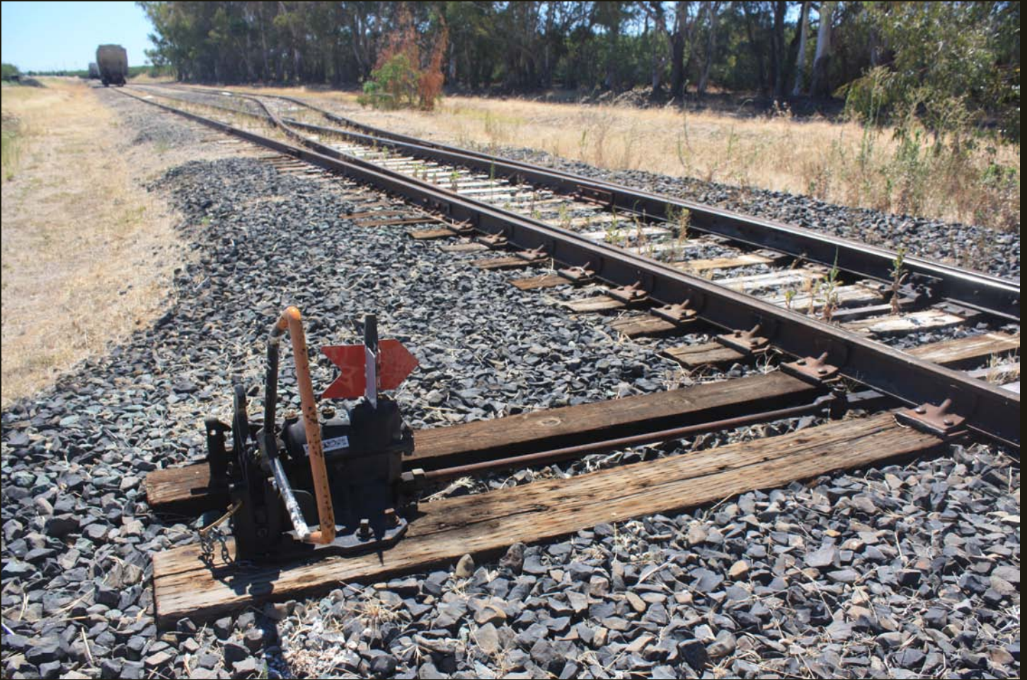
Eastward view of the WS&M re-alignment 2 miles west of Willows near the end of track, same siding and stored car as the photo before last. The end-of-track curve to the north is just behind the viewer.
