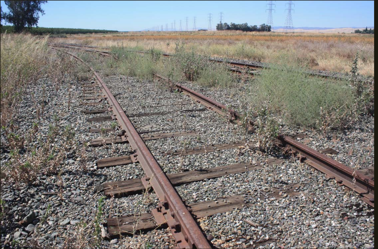
Slightly different southward view of the same curve and siding as previous. Now we are 100 yards north of the WS&M grade, which runs along the edge of the orchard in the left distance.
