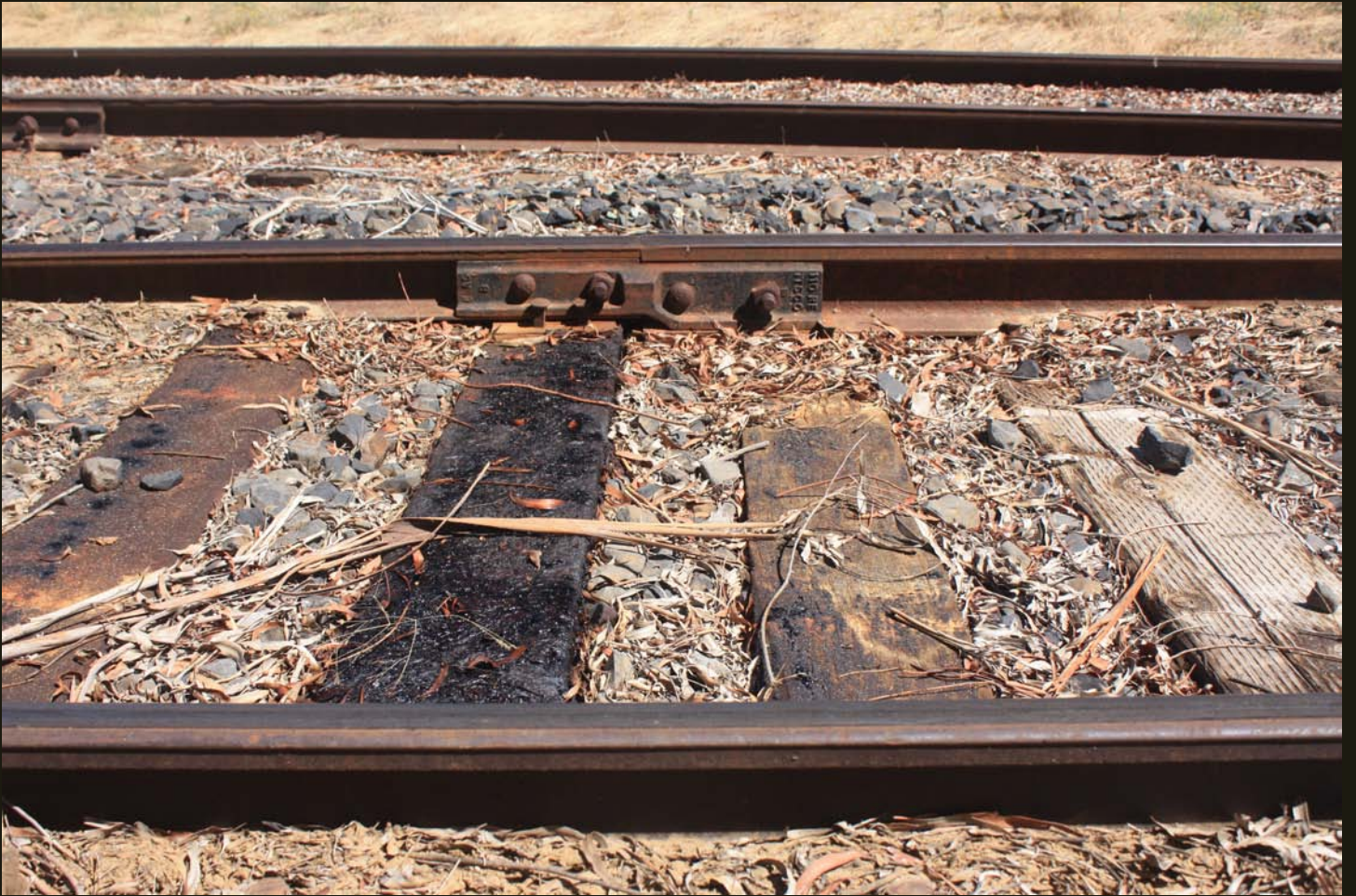
This change in track weight likely occurred in 1951, when the end-of-track was realigned to access the Johns-Manville Plant.
