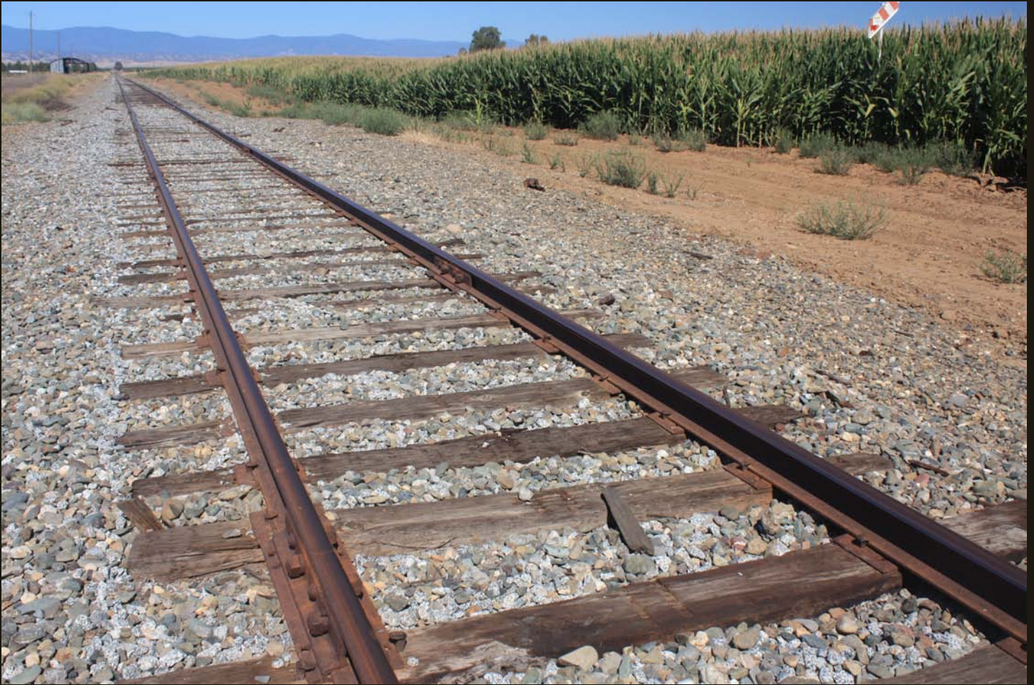
Westward view of the WS&M in corn fields one mile west of Willows. Note the foothills of the California Coast Range in the distance.
