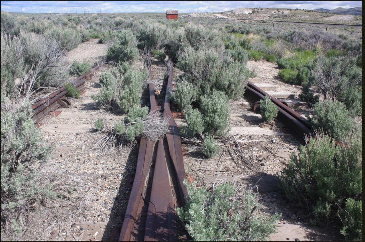
Northwestward view of the NN mainline; the engine house is out of sight to the left. The right (northeast) track at this switch is a siding for the north branch of the Cobre turning wye (the siding rejoins the mainline between the two branches of the wye). The CP (1869), now UP, is in the right distance.
