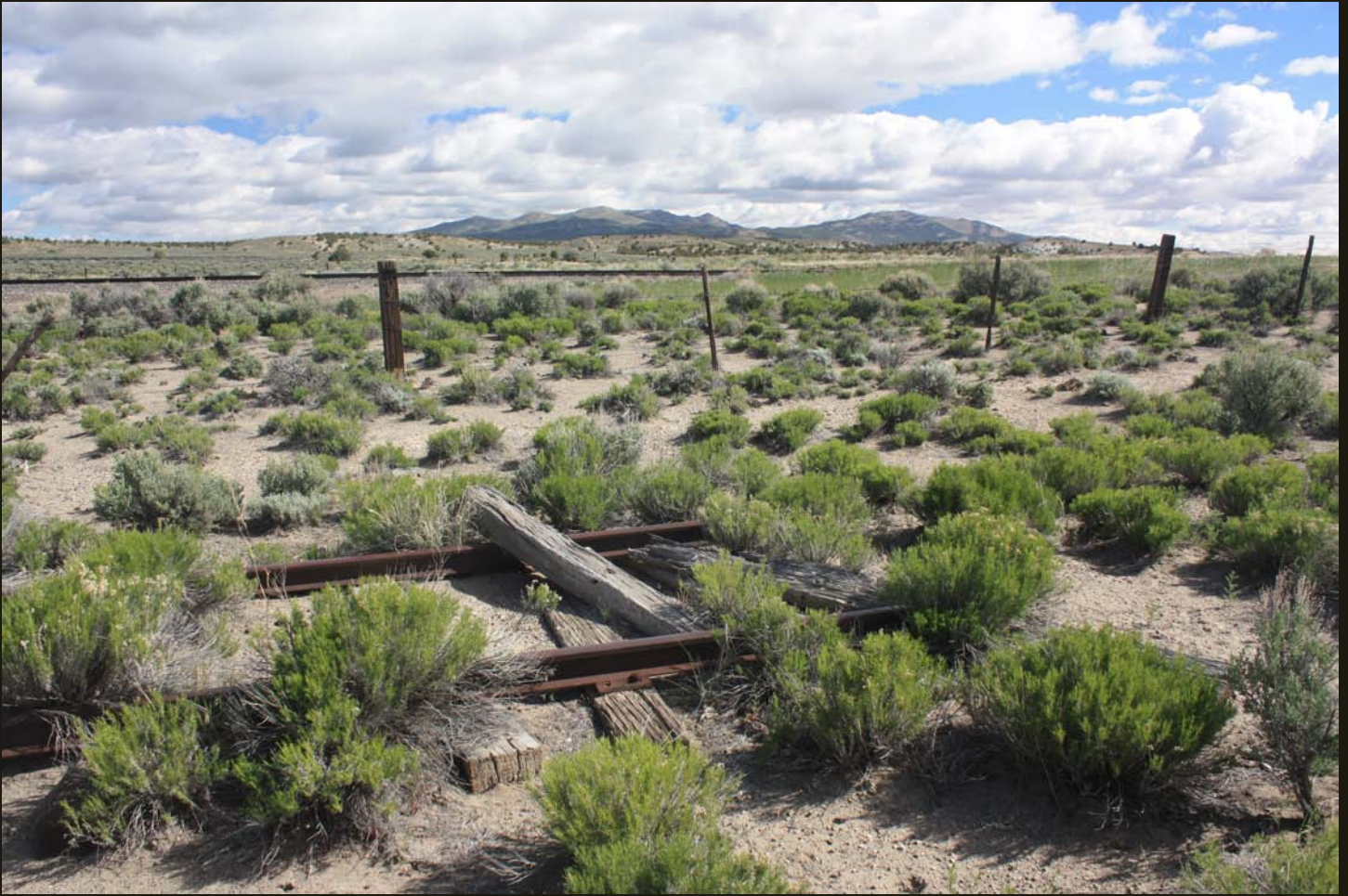
Northward view of the end-of-track at the east end of the Cobre turning wye (foreground), 1,200 feet east of the NN (1906) mainline. The CP/SP/UP is in the distance.
