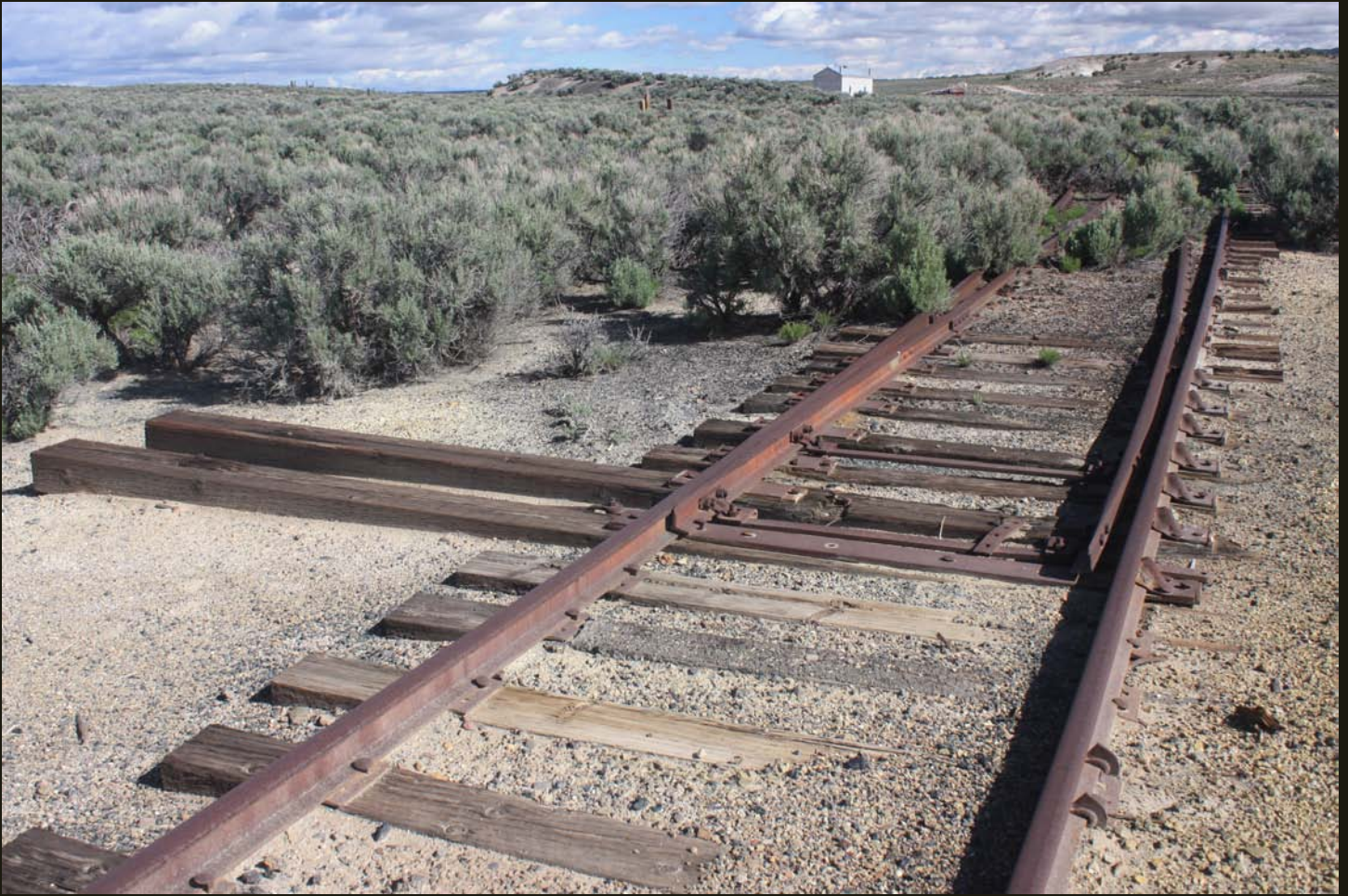
Northwestward new of the NN (1906), a few steps south of the previous location, where the track that leads back to the engine house (visible in the distance) joins the NN mainline, now a single track.
