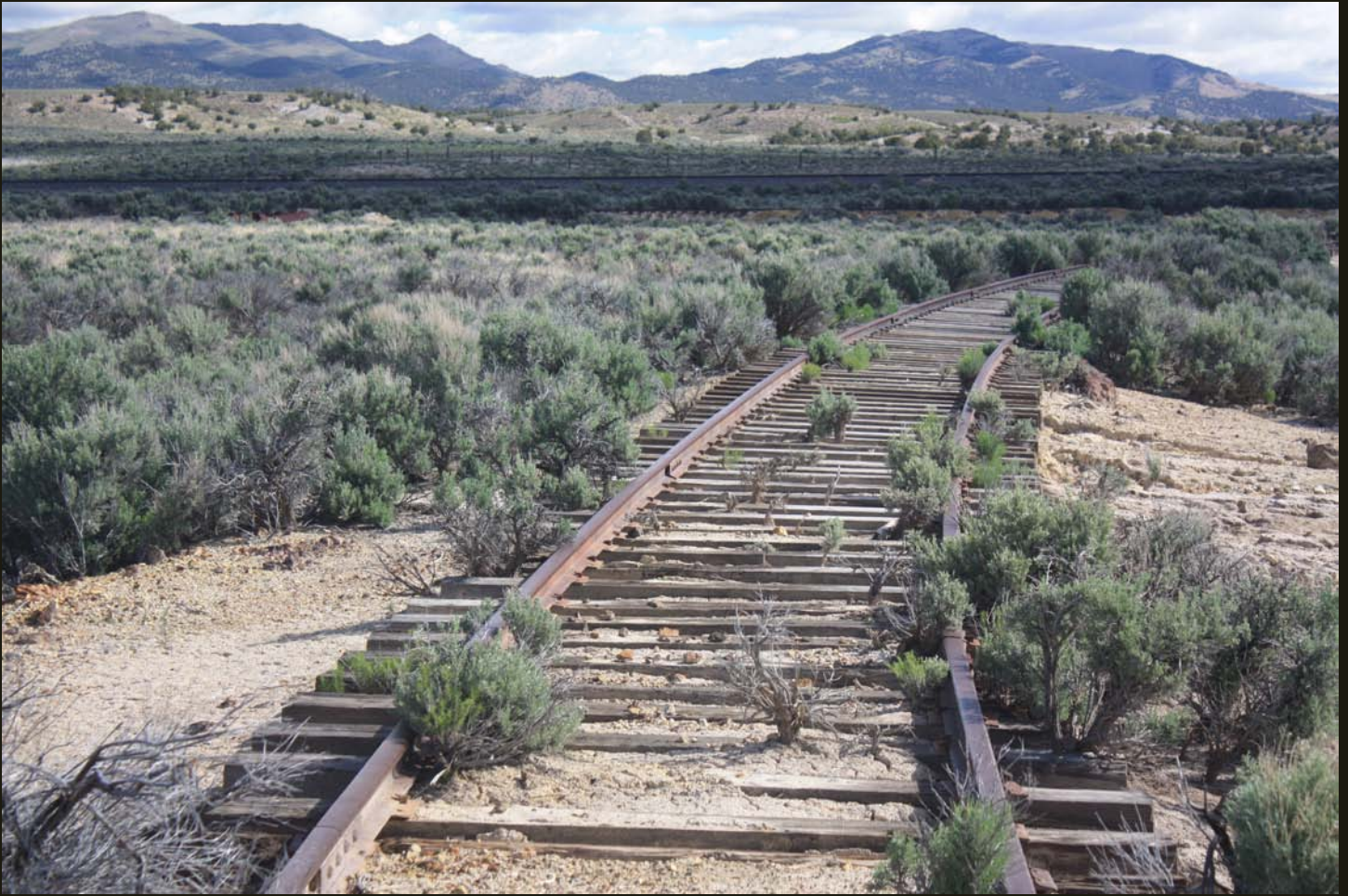
Northward view of the south branch of the Cobre turning wye (foreground), a few steps southwest of the previous location. The CP/SP/UP mainline is in the distance and the north branch of the wye is barely visible on this side of the mainline.
