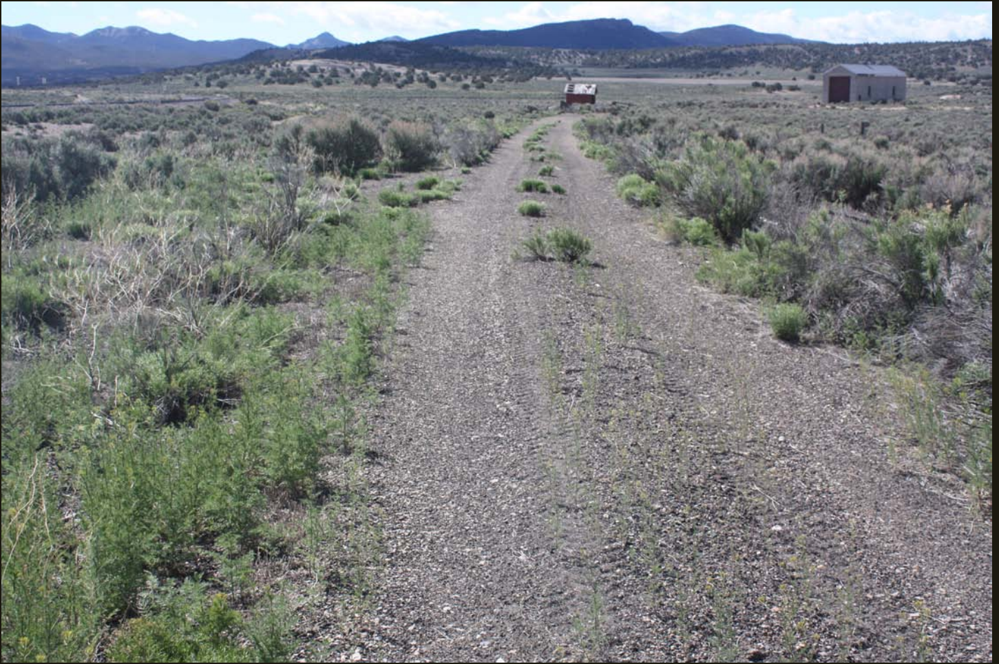
Southeastward view of the abandoned NN (1906) grade, 300 feet southeast of the previous location. The CP/SP/UP is in the upper left, where it turns 90 degrees, from northwest-southeast west of Cobre (e.g. as in first photo) to northeast-southwest east of Cobre.
