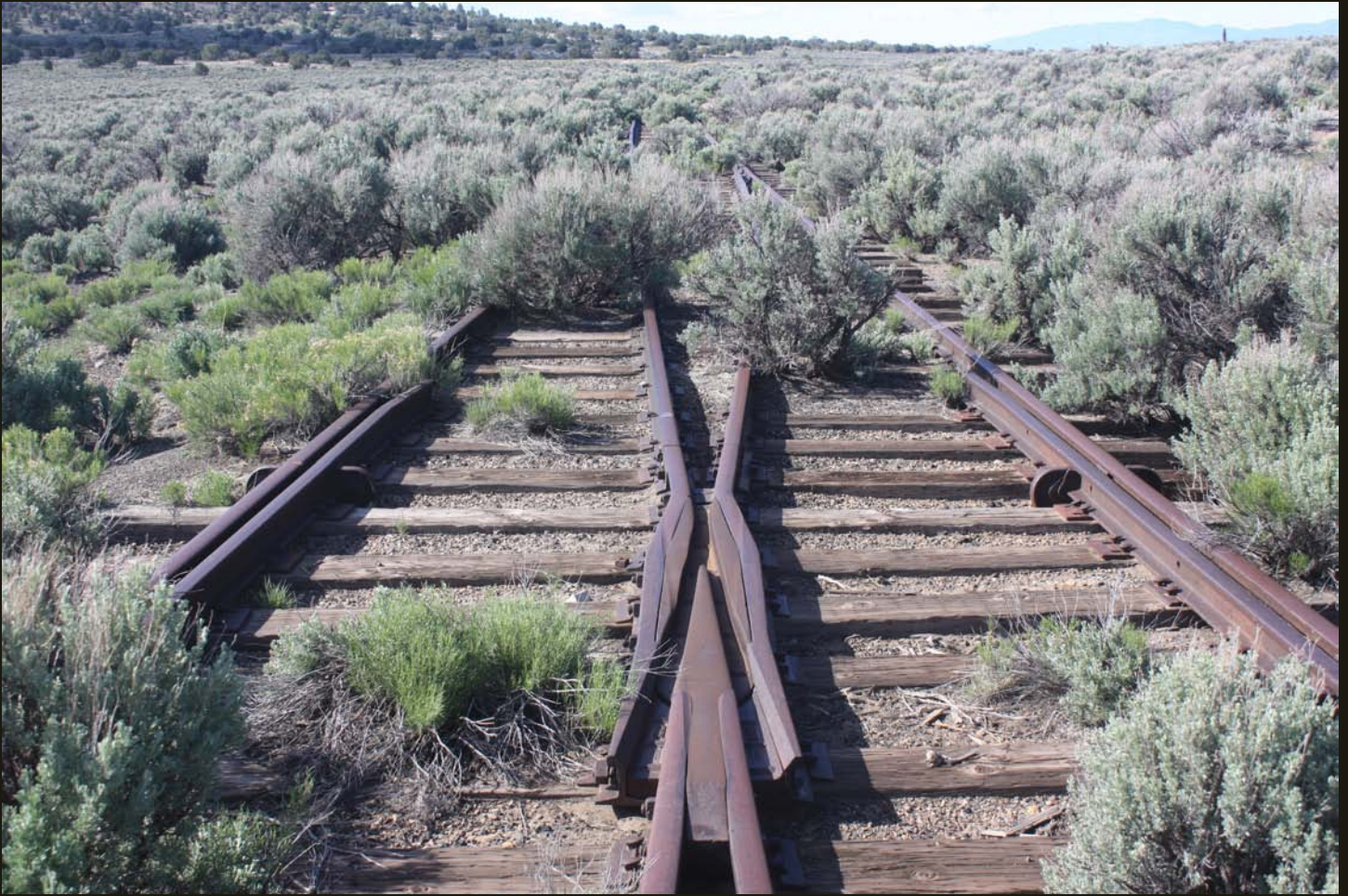
Southward view of the connection between the NN (1906) mainline on the right and the south branch of the Cobre turning wye on the left. The two tracks converge to a single track that leads southward out of Cobre. This location is 1,700 feet south of the end-of-track at the north end of Cobre.
