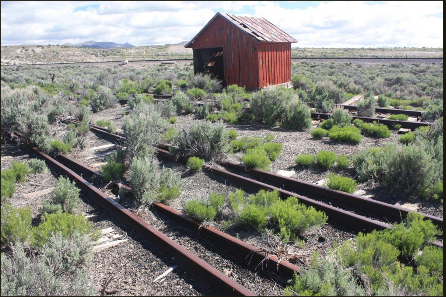
Another northeastward view of the handcar shed at Cobre. There are two NN tracks; the track in front of the shack is the NN (1906) mainline; the track in the foreground is veering away from the mainline and is splitting via a switch to form another track, both of which lead to the engine house.
