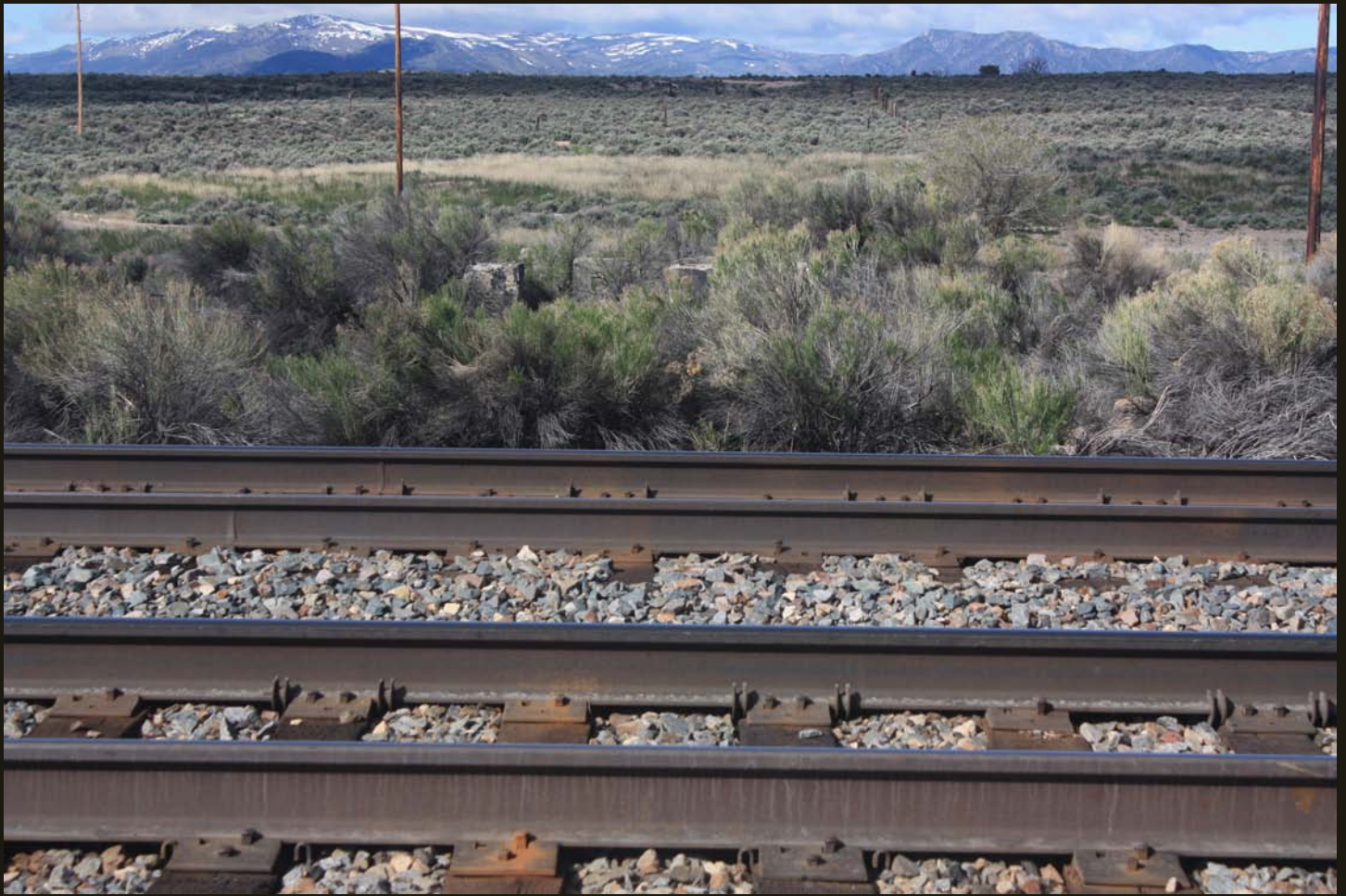
Southwestward view of the CP (1869), now UP, and the Pequop Range, same location as previous. The NN (1906) siding is lower than and behind the mainline tracks. Note the old foundations just left of center.
