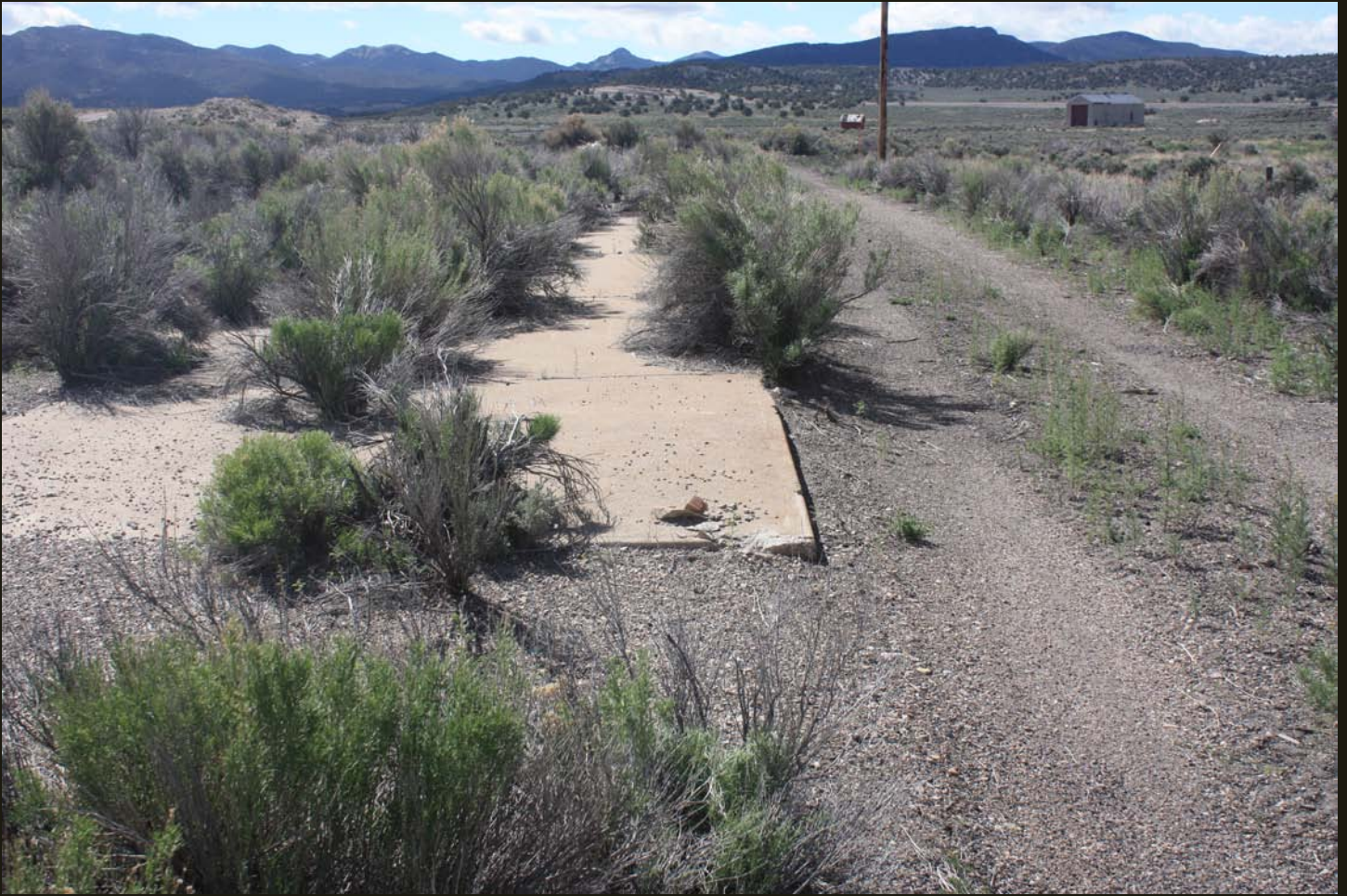
Southeastward view of the abandoned NN (1906) grade and an old foundation, same location as previous. Note the same engine house as in the first photo and another building, a handcar shed, just left of the pole – that's Cobre.
