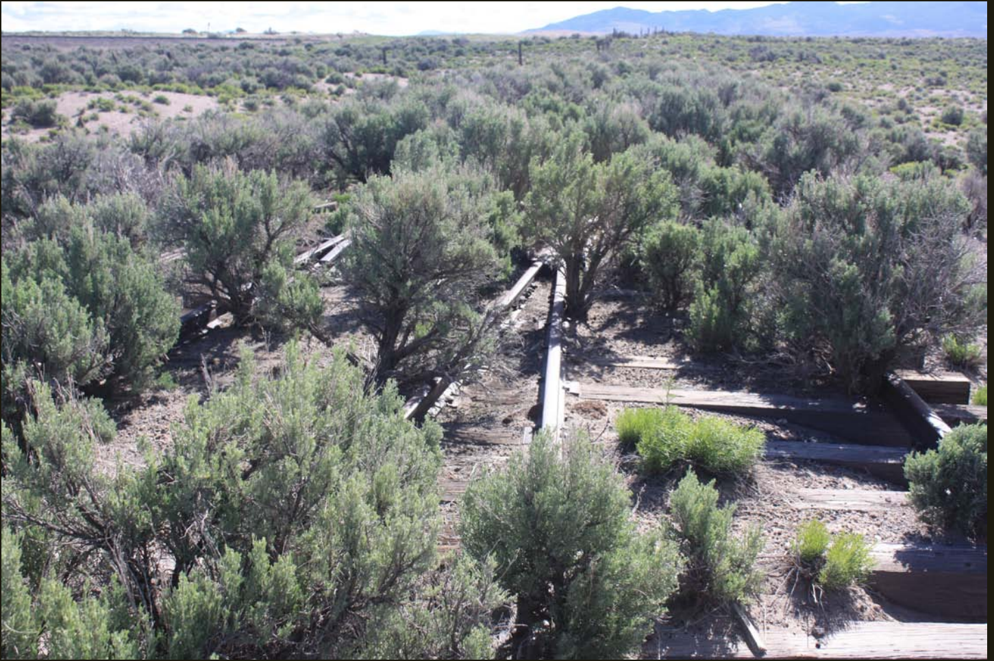
Northeastward view of the tip of the Cobre turning wye, where the two branches meet. There is another 350 feet of track beyond the tip and another 200 feet of track-less grade beyond that, much more than needed to turn an engine and tender; the wye turned trains. The CP/SP/UP is in the upper left distance, where it turns 90 degrees, from northwest-southeast west of Cobre (e.g. as in first photo) to northeast-southwest east of Cobre.
