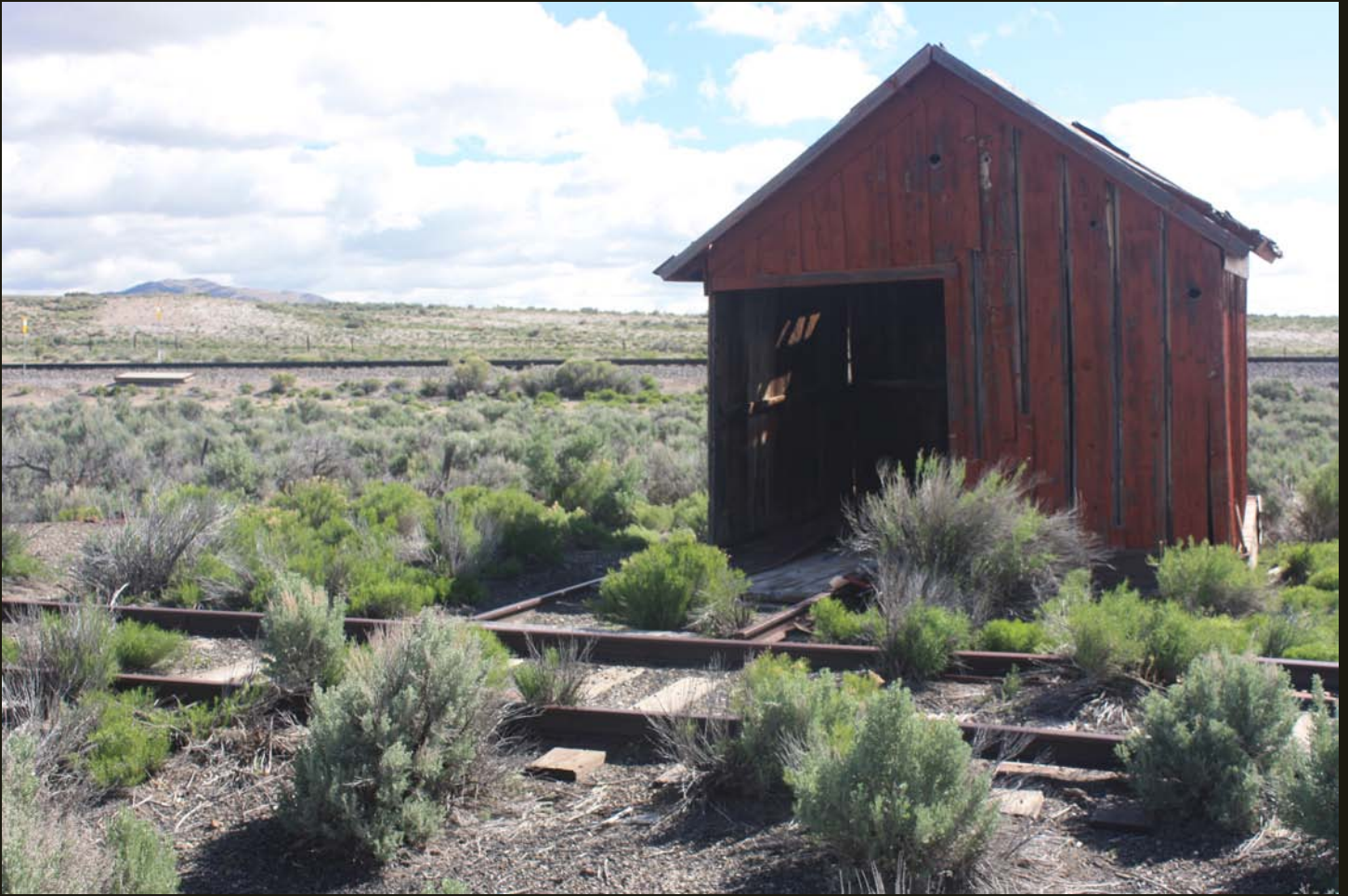
Northeastward view of the NN's handcar shed at Cobre. The CP/SP/UP mainline is behind the shed. The track in the foreground is one of two tracks after the split in the previous photo; the second track is just behind viewer. Note the rails in front of the shed and perpendicular to the track; I've seen this before but I don't know what it's for.
