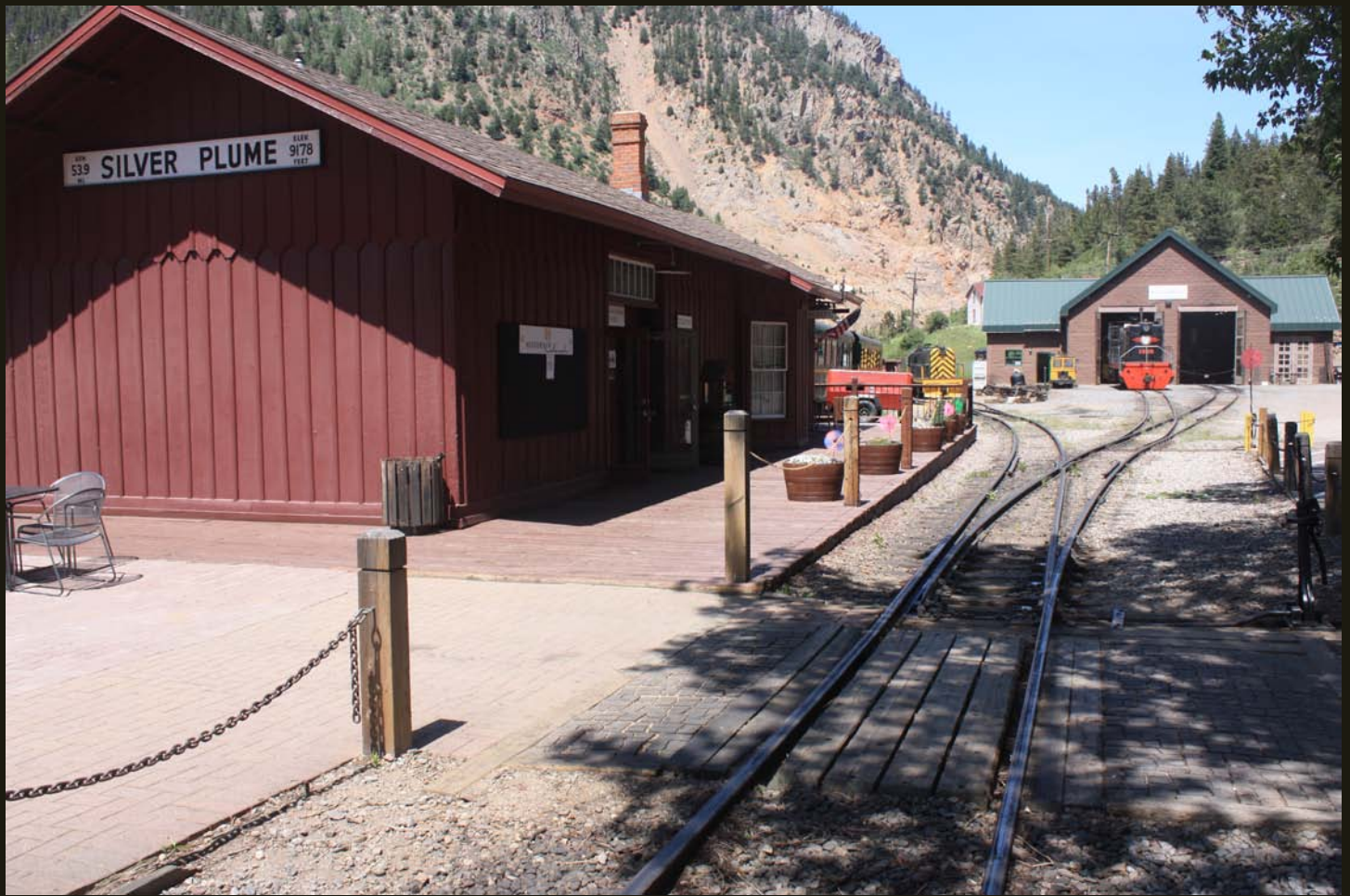
Eastward (downstream) view of the Georgetown Loop Railroad at Silver Plume. The left track is the mainline down to Georgetown, the right track goes to an engine house. The end-of-track is behind (west) of the viewer.
