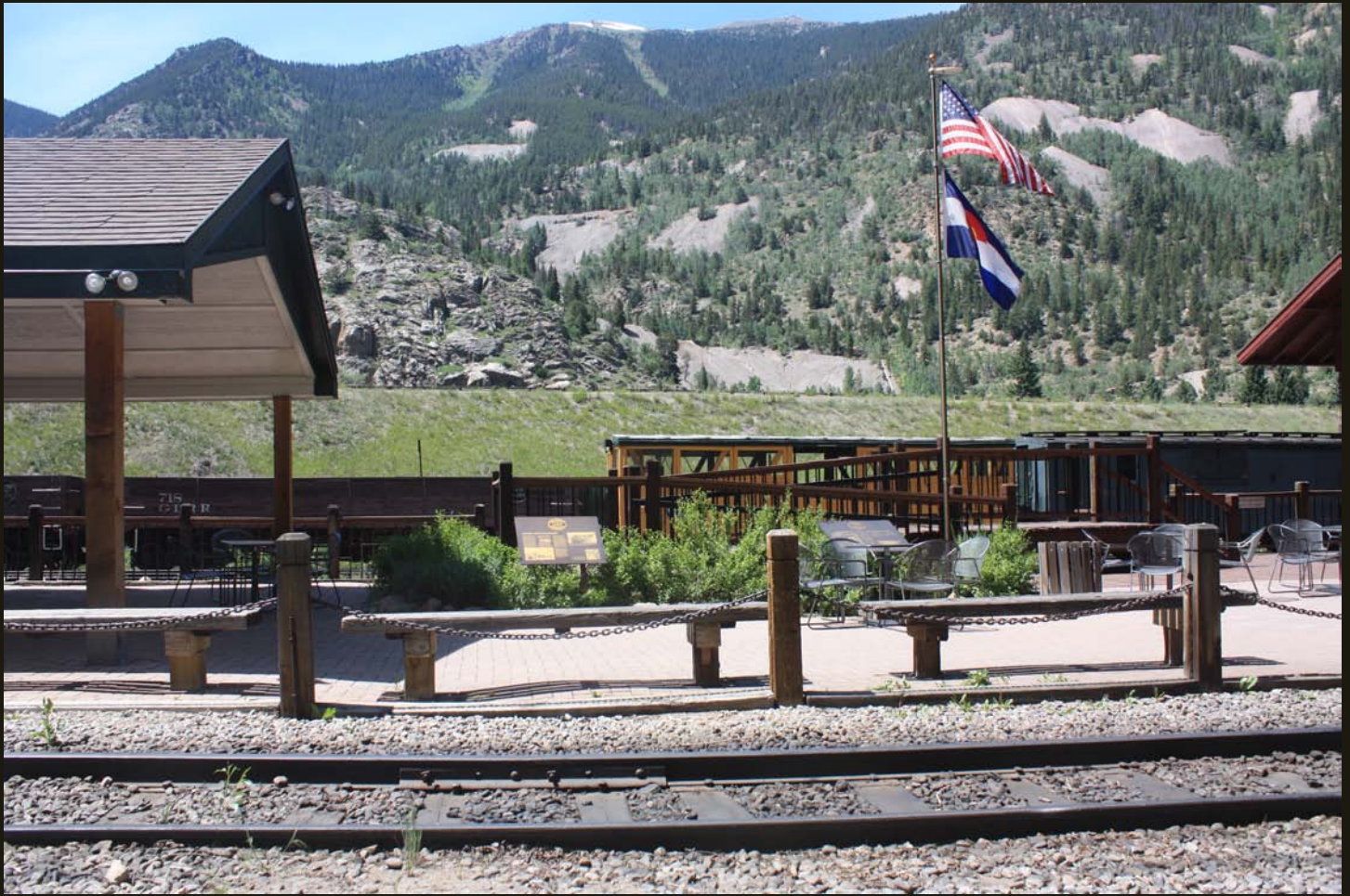
From foreground to background in this northward view at Silver Plume: the Georgetown Loop Railroad tracks, the Georgetown Loop Railroad passenger loading area, stored rail cars at the Georgetown Loop Railroad Silver Plume Yard, U.S. Highway 6, tailings from silver mines, and snowcapped peaks above 12,000 feet elevation.
