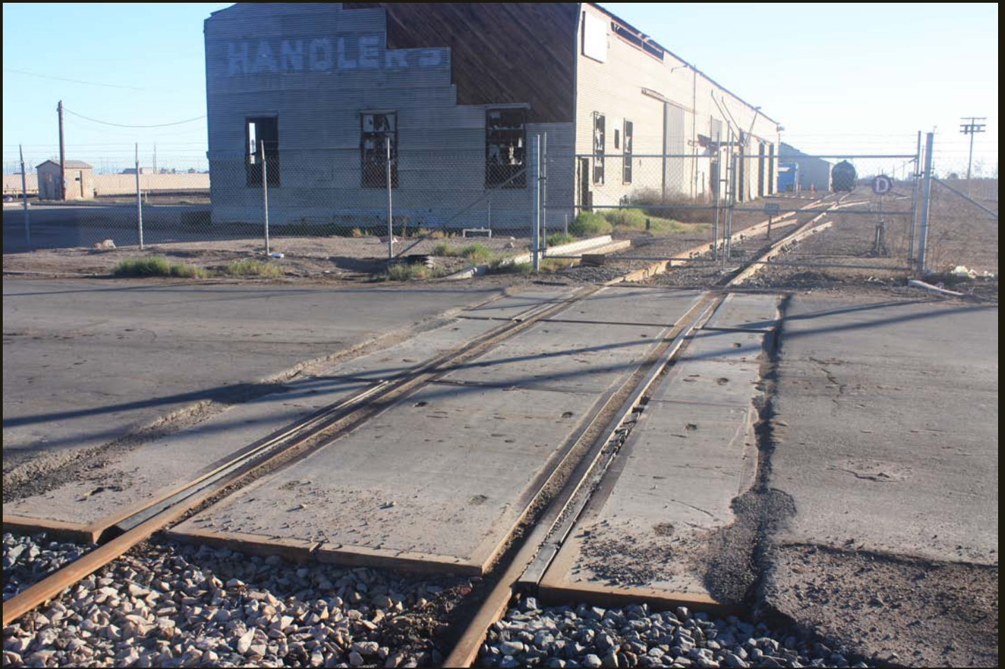
The spur in the previous photo leads to this abandoned warehouse.
