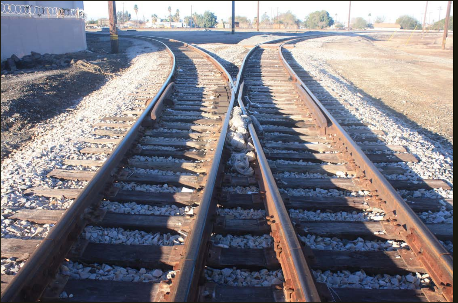
Westward view of the east tip of the HI (1904) wye.
