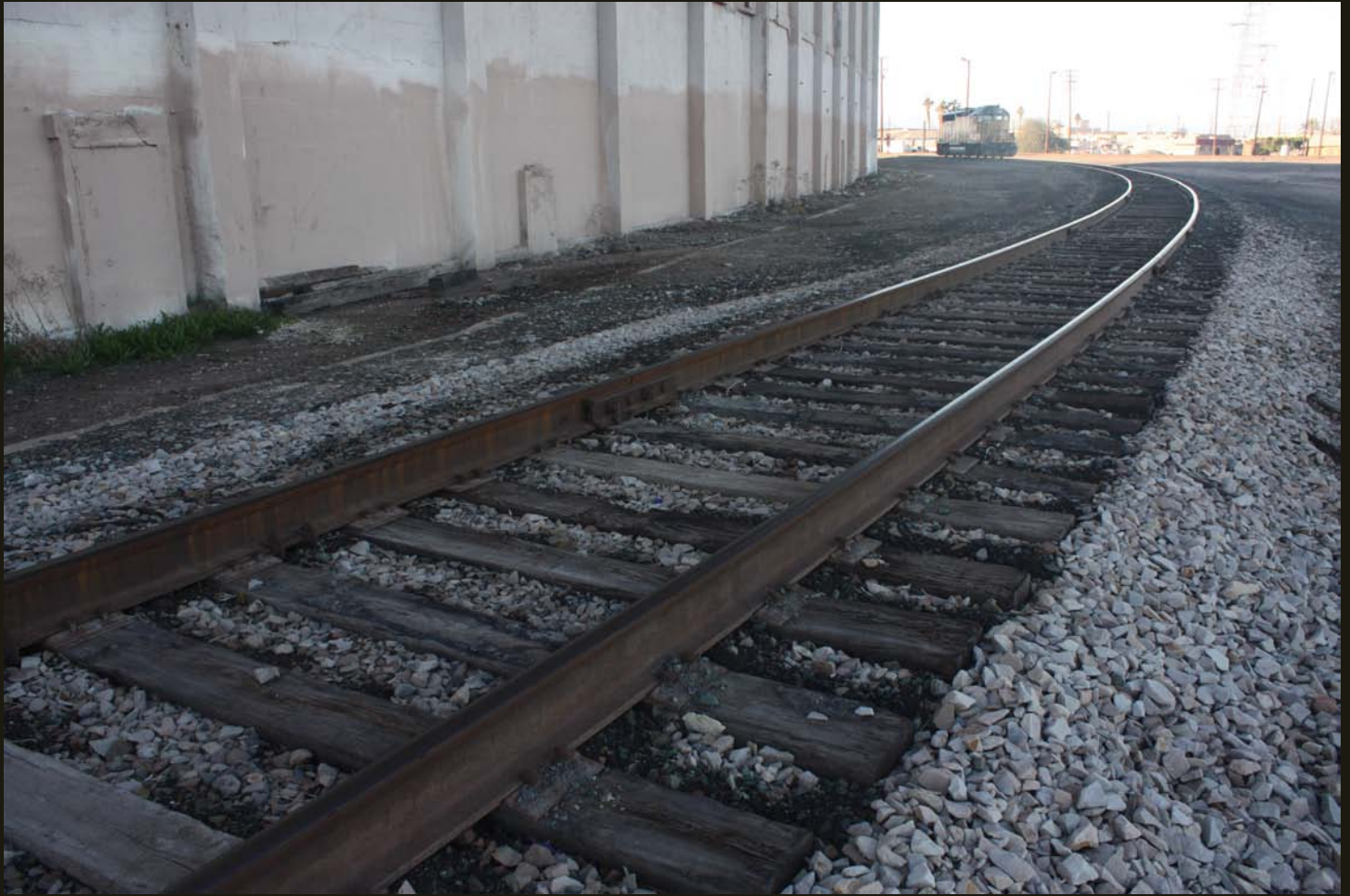
Westward view; the engine in the distance is on the south branch of the HI (1904) wye. Note the building wall curved parallel to the south branch of the wye.
