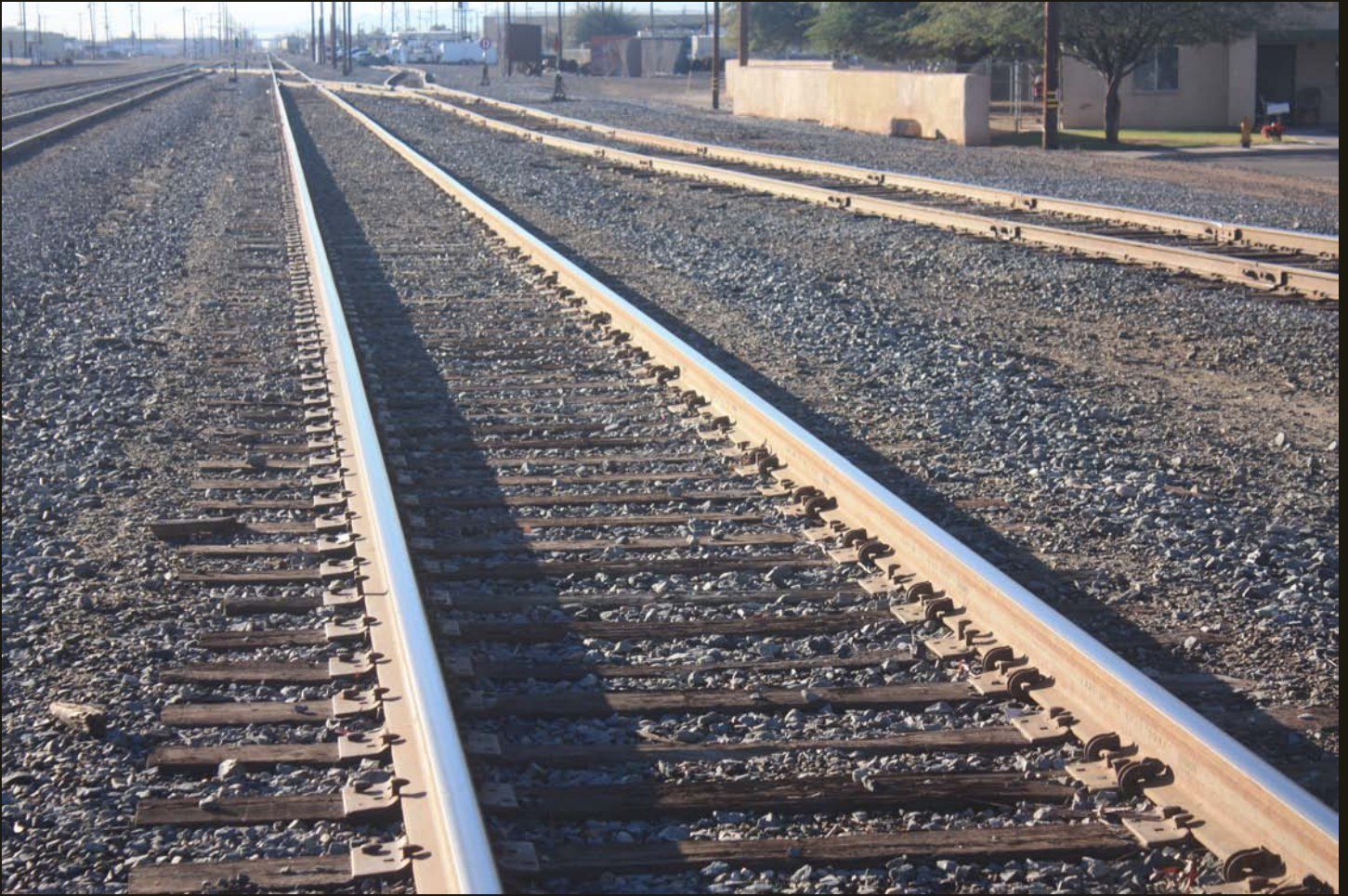
Southward view at the same location as previous. The south branch of the SD&A (1919) wye is on the far right.
