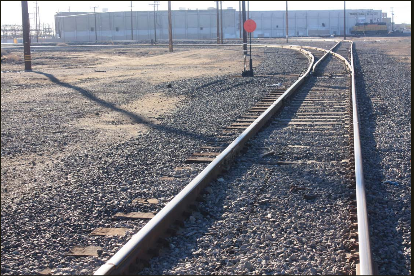
Southward view from the same location as the previous photo. The track in the foreground is the north branch of the wye for the HI (1904), with a switch to a spur. The engine in the right distance is on the south branch of the wye for the HI, and the wall of the huge building behind the engine is curved parallel to the south branch of the HI wye.
