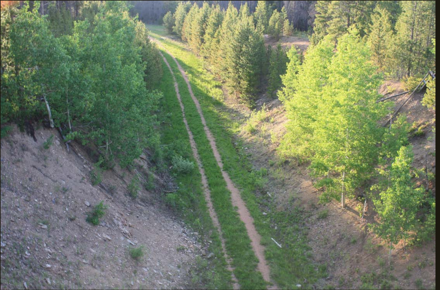
The LHP&P grade at Wyocolo, the same location as above. Note the deep cut in the foreground.
