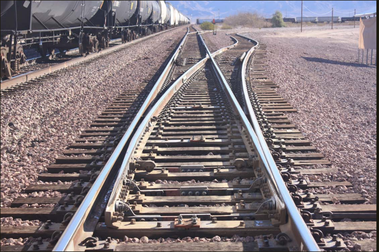
Eastward view of the double-tracked west branch of the A&C (1910) wye. The cars beyond to the right are on the east branch of the wye. The stored oil tank cars and other cars on the left are on a AT&SF/BNSF siding.
