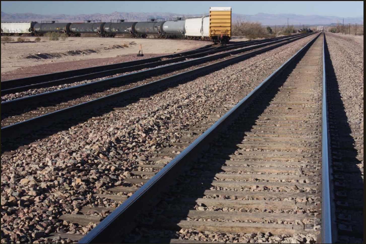
Westward view of the east branch of the A&C (1910) wye, used for car storage, where it merges with the siding; the center and right-hand tracks are the double-tracked BNSF Southern Transcon (SP (1883) Needles Branch).
