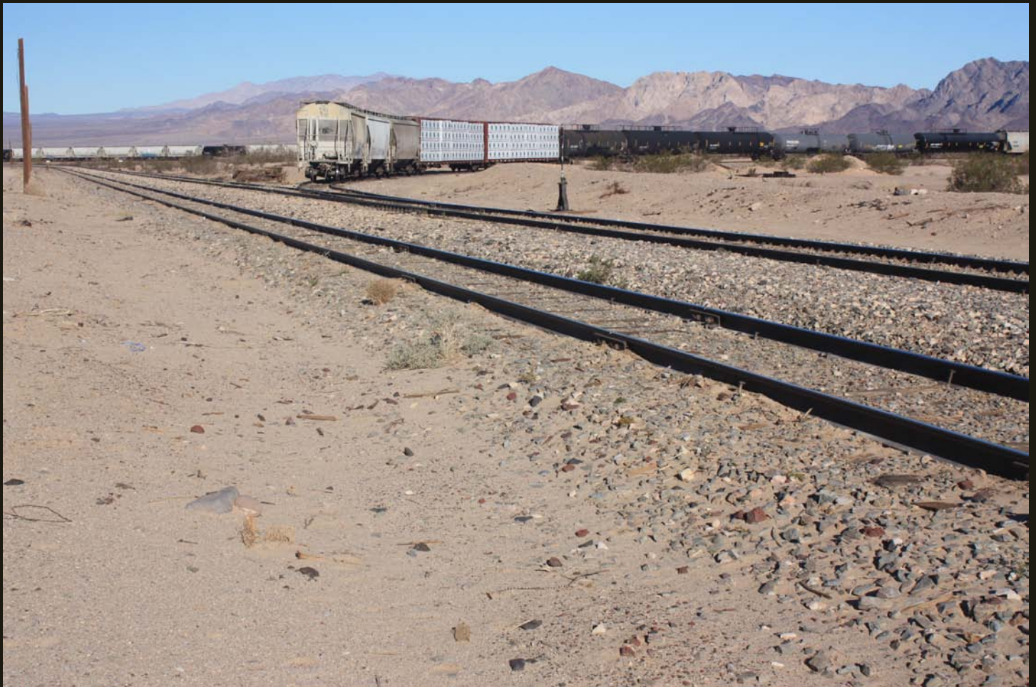
Northward view of the southern tip of the A&C wye. The double-tracked west branch of the A&C (1910) wye merges with the single-tracked east branch, used for car storage.
