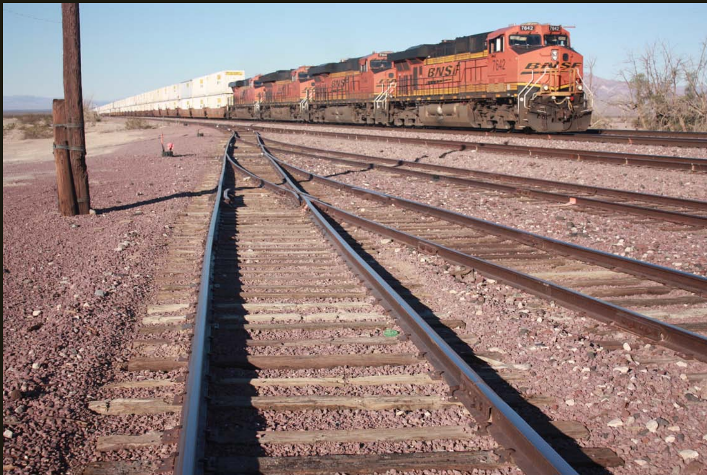
Northwestward view a few steps east of the previous location, with the first switch for the Cadiz yard left of center and several switches for the yard in the foreground.
