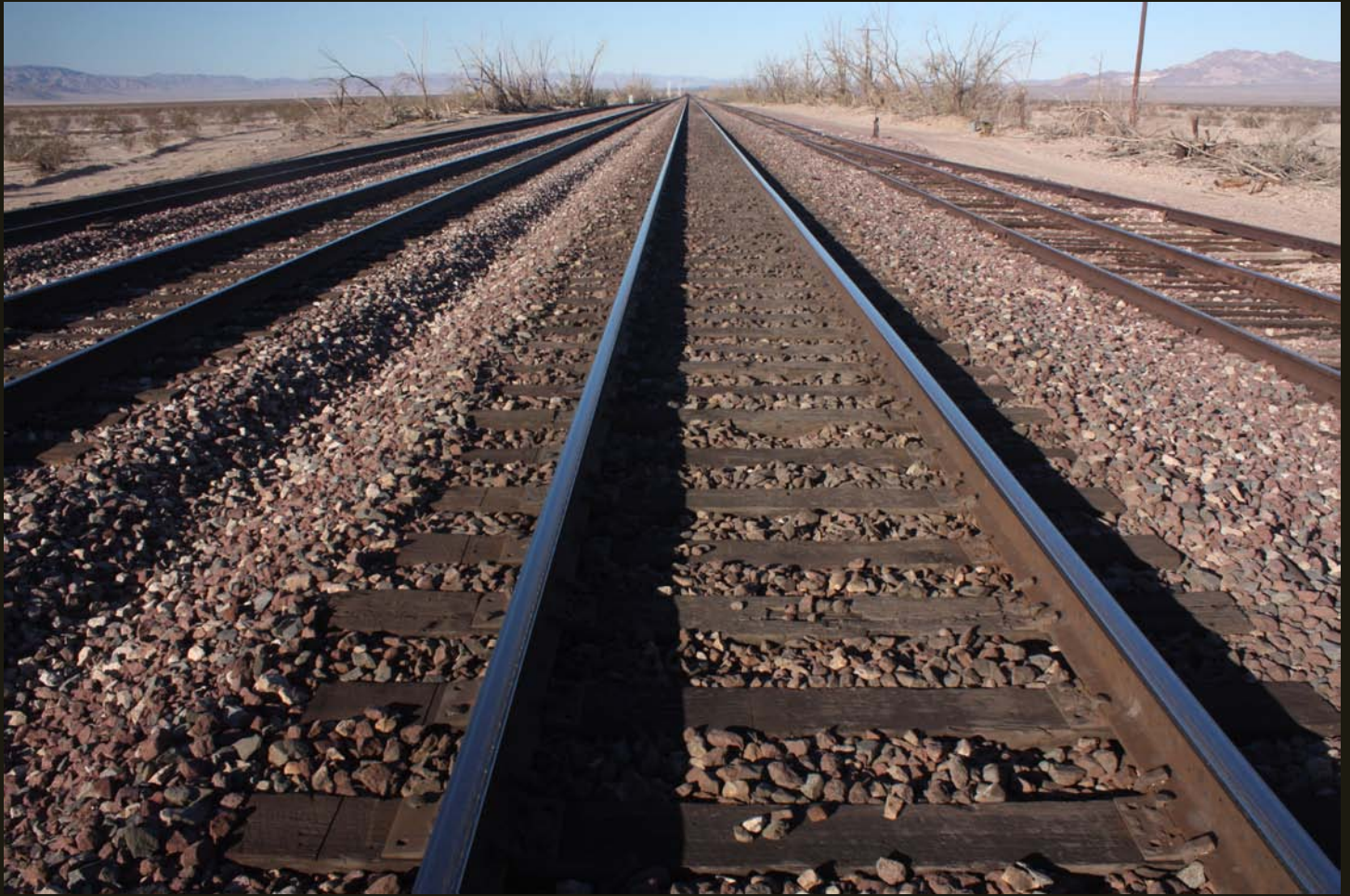
Westward view just west of the satellite image, from left (south) to right (north): the same siding seen in the previous photo; the two tracks of the BNSF main line; and the old siding that extends a mile west with a switch to a second "old" siding.
