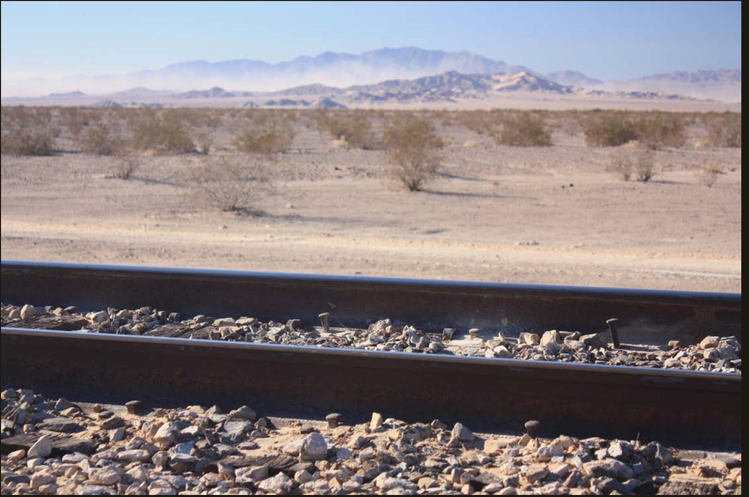
Westward view of the A&C (1910), same location as previous, with a dust storm brewing in the distance.
