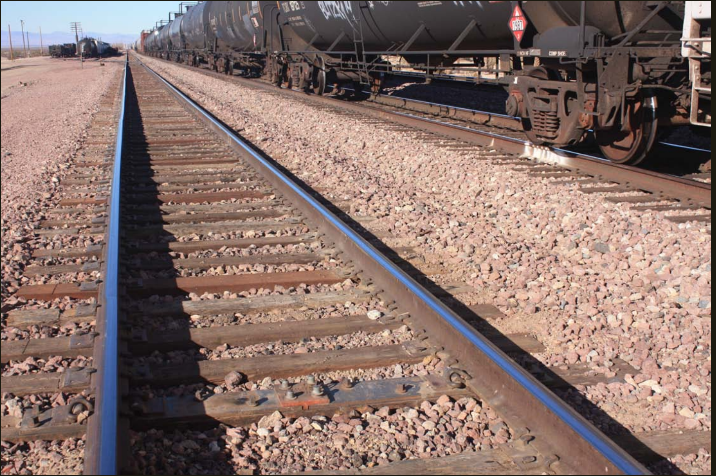
Westward view of the east end of the Cadiz yard (left distance); the switch for the west branch of the A&C (1910) wye is just behind the viewer.
