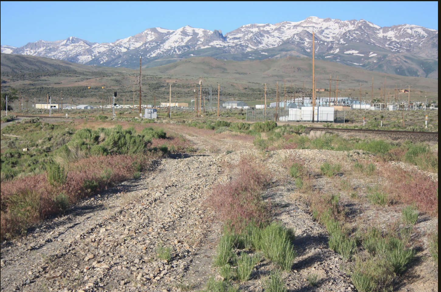
Southward view 2,200 feet southwest of the CP (1869)-OSL Wells Branch grade crossing (previous photo). The trackage that runs across the photo is the WP (1909) and the curved grade in the foreground is the abandoned OSL Wells Branch (1926) connection built in 1928. Note that signals for this connection are still in place at the far left, where a single switch once connected the lines (no wye). The 11,000+ foot East Humboldt Range in the background was capped by glaciers during the Pleistocene epoch, as indicated by U-shaped valleys evident in this view. Glacial melt waters drained westward to Pleistocene Lake Lahontan and eastward to Pleistocene Lake Bonneville.
