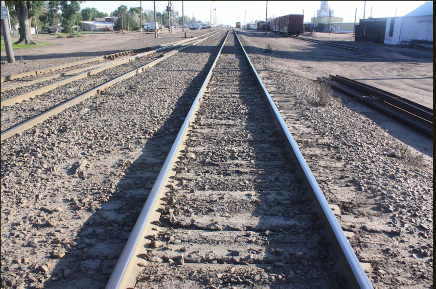
Southward view at same location as above; the DP mainline is the un-rusted track in the foreground, with a siding to the left for the UP Julesburg Branch, and the switch and track to the far left is the south branch of the La Salle wye for the Julesburg Branch.
