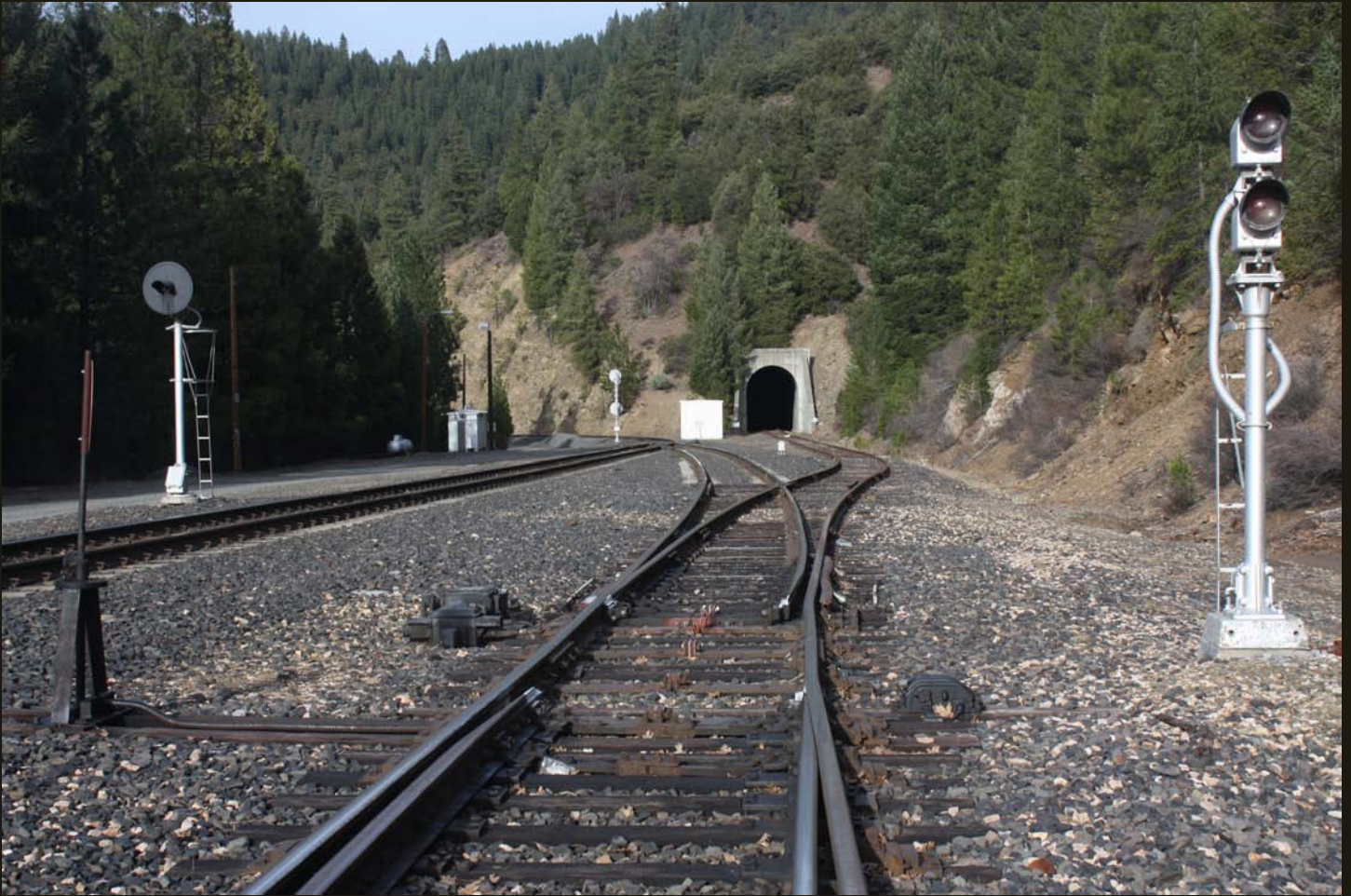
This is the second switch off of the 1909 WP mainline, which continues to the left. The line on the right with a tunnel is the eastern connection with the 1931 branch line.
