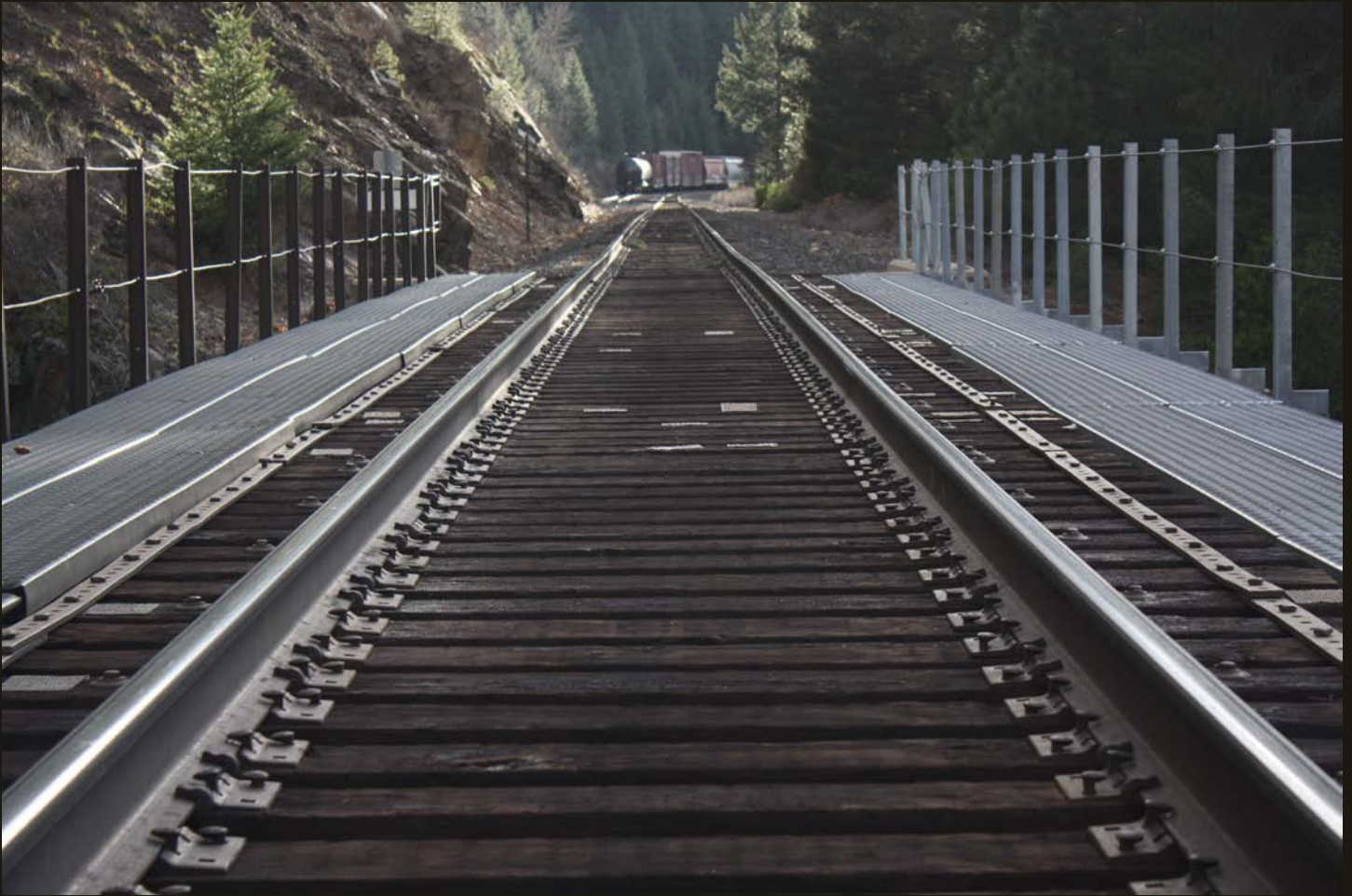
The third switch on the Keddie Wye is the northern switch where the two 1931 connections to the WP mainline merge. This southward view of the 1931 Inside Gateway line is a short distance north of the third switch, which I did not walk to.
