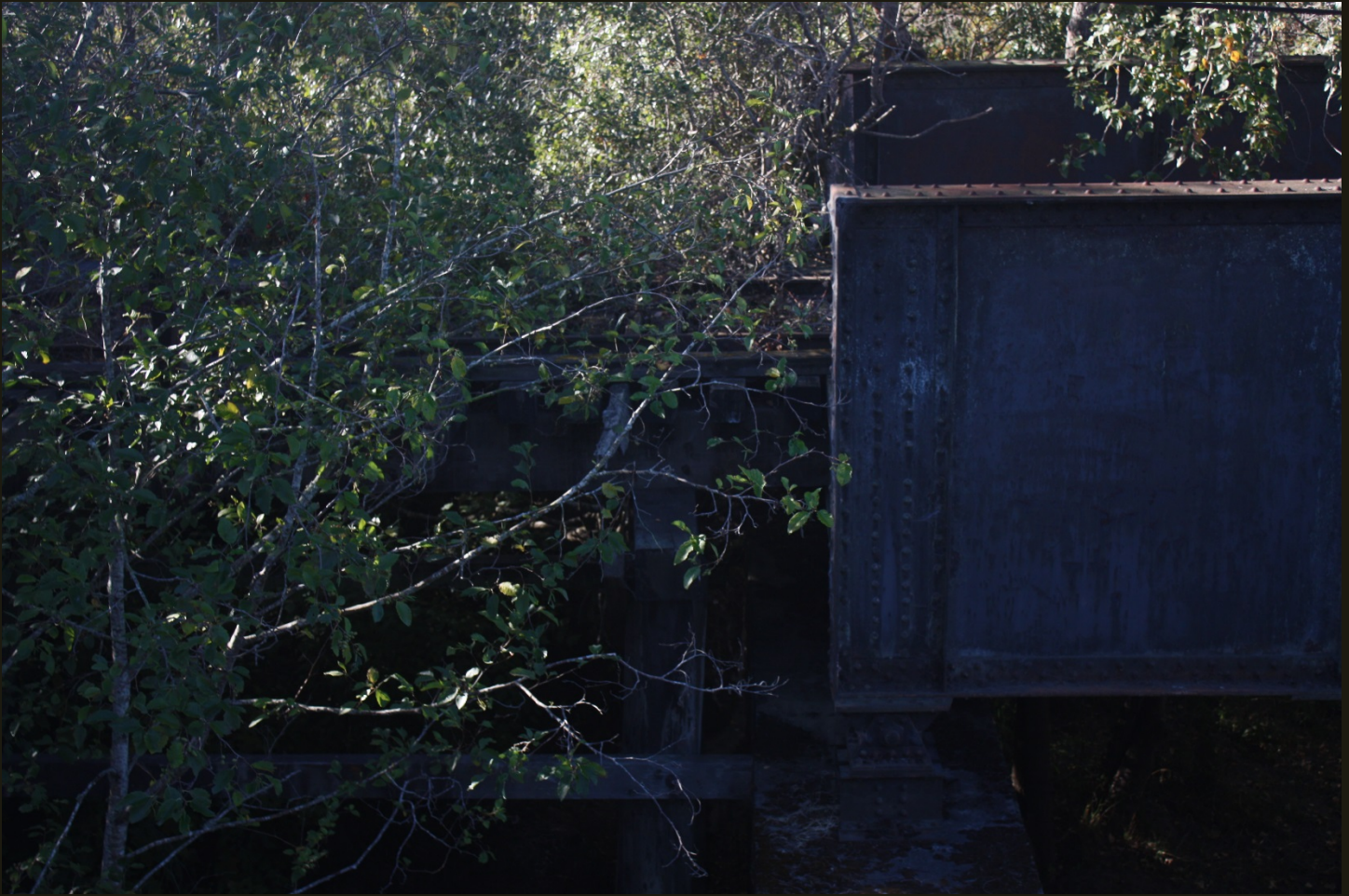
Southward view at Carlotta, California, where an overgrown bridge carries the ER&E (1884) over Yager Creek. This location is 4 miles east of Alton and 2 miles east of the reported end-of-track at Burnell's Station/Hydesville (Hydesville is the town that developed along California Highway 36 next to Burnell's Station). The only literature I could find about the line east of Burnell's Station is that, following completion of the line to Burnell's Station in 1884, subsequent construction was limited to small extensions and spurs, and that topo maps show NWP tracks extending 7 miles east of Burnell's Station, including this location at Carlotta.
