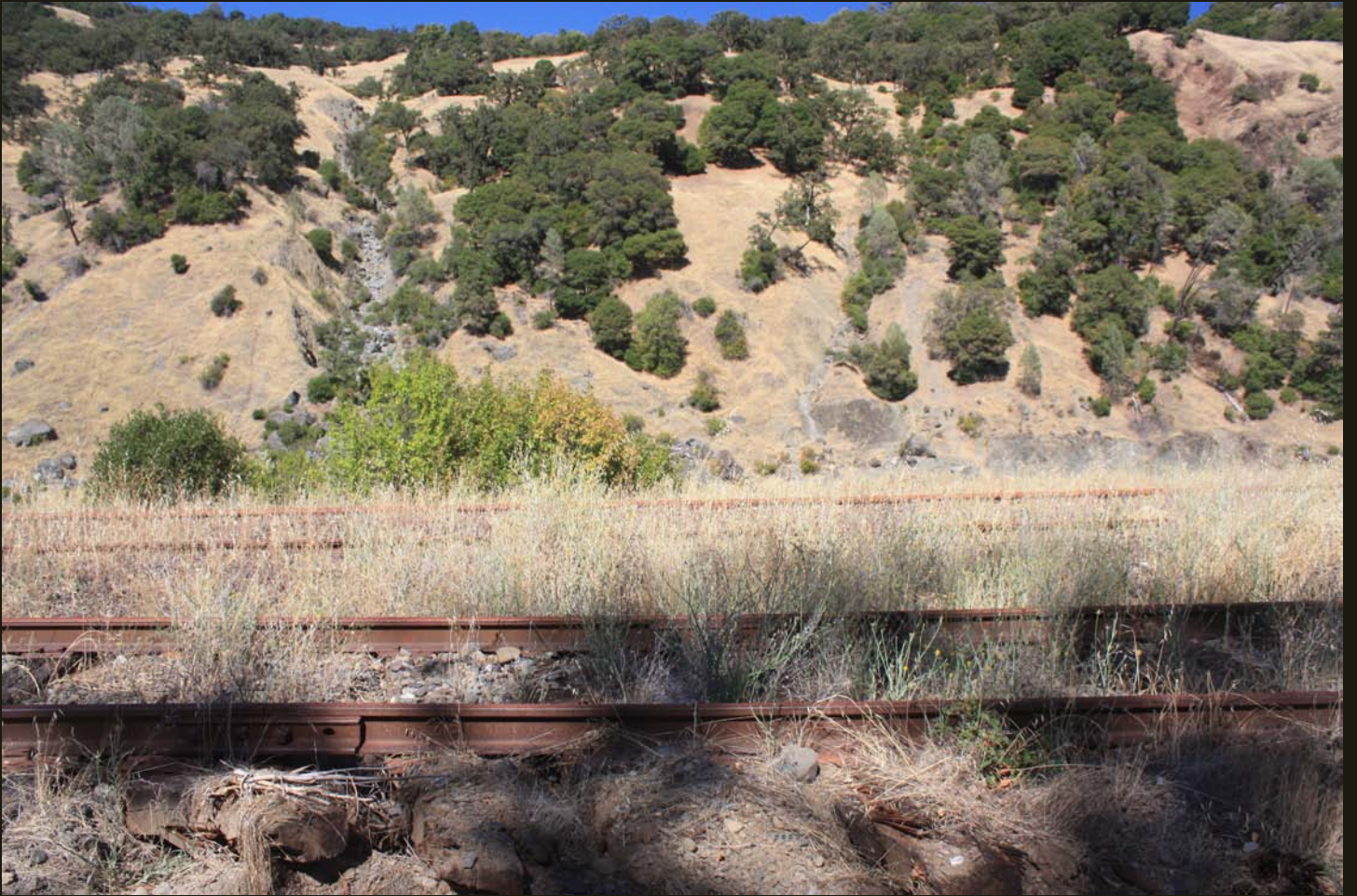
Siding and main line at Dos Rios.
