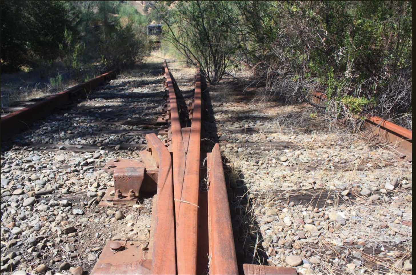
The railroad crane and sidings at Dos Rios.
