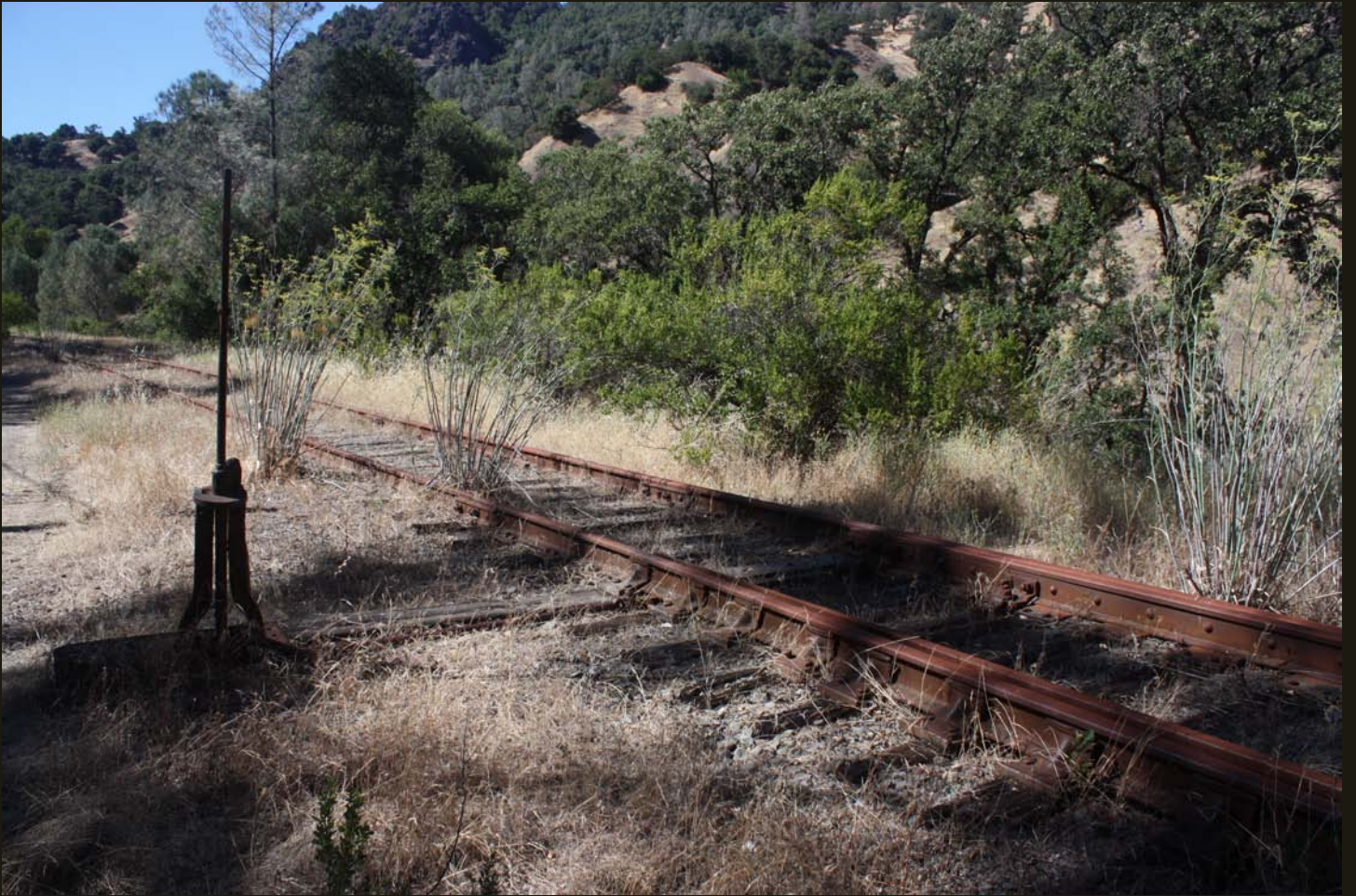
Switch for a siding at Dos Rios.
