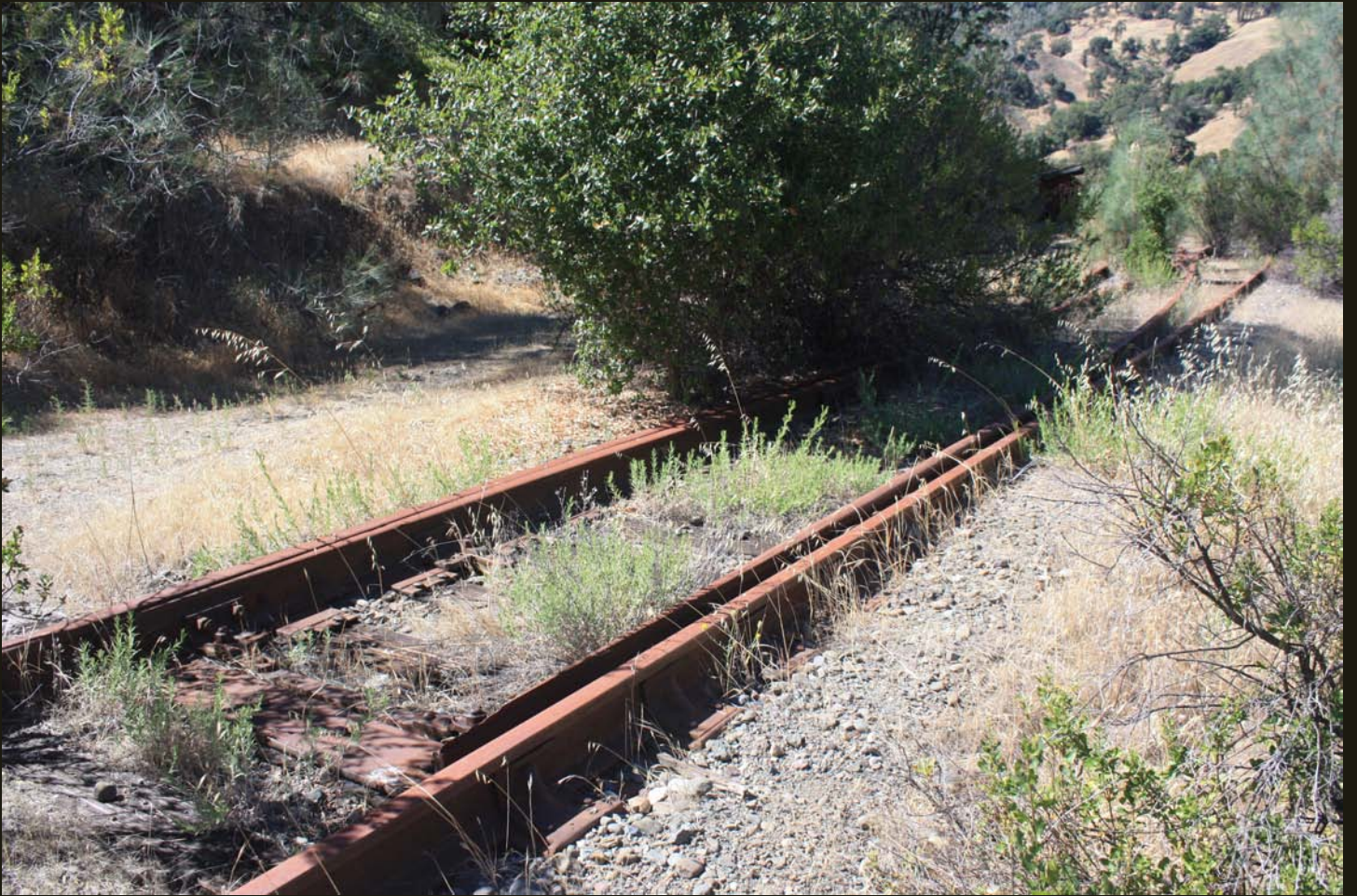
A switch for sidings at Dos Rios.
