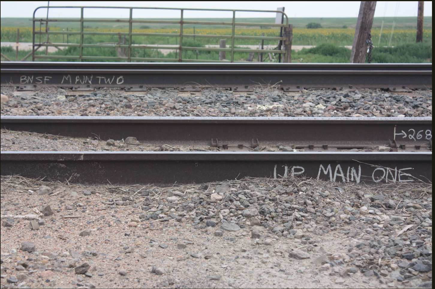
Eastward view of the double track D&RGW-C&S (1911) Southern Joint Line. Somebody conveniently marked the lines for us – the near (western) line is UP (D&RGW successor) and the further line is BNSF (C&S successor). These are well-used welded rails.
