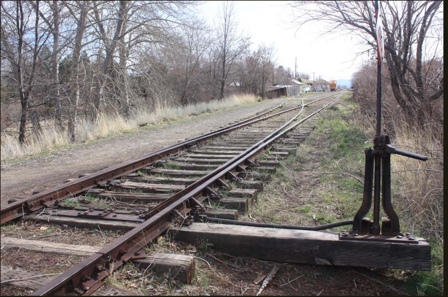
The switch for the Susanville Depot siding; the depot is the pink building in the distance. This eastward view shows most of the rails still present and the Bizz Johnson trail to the left.
