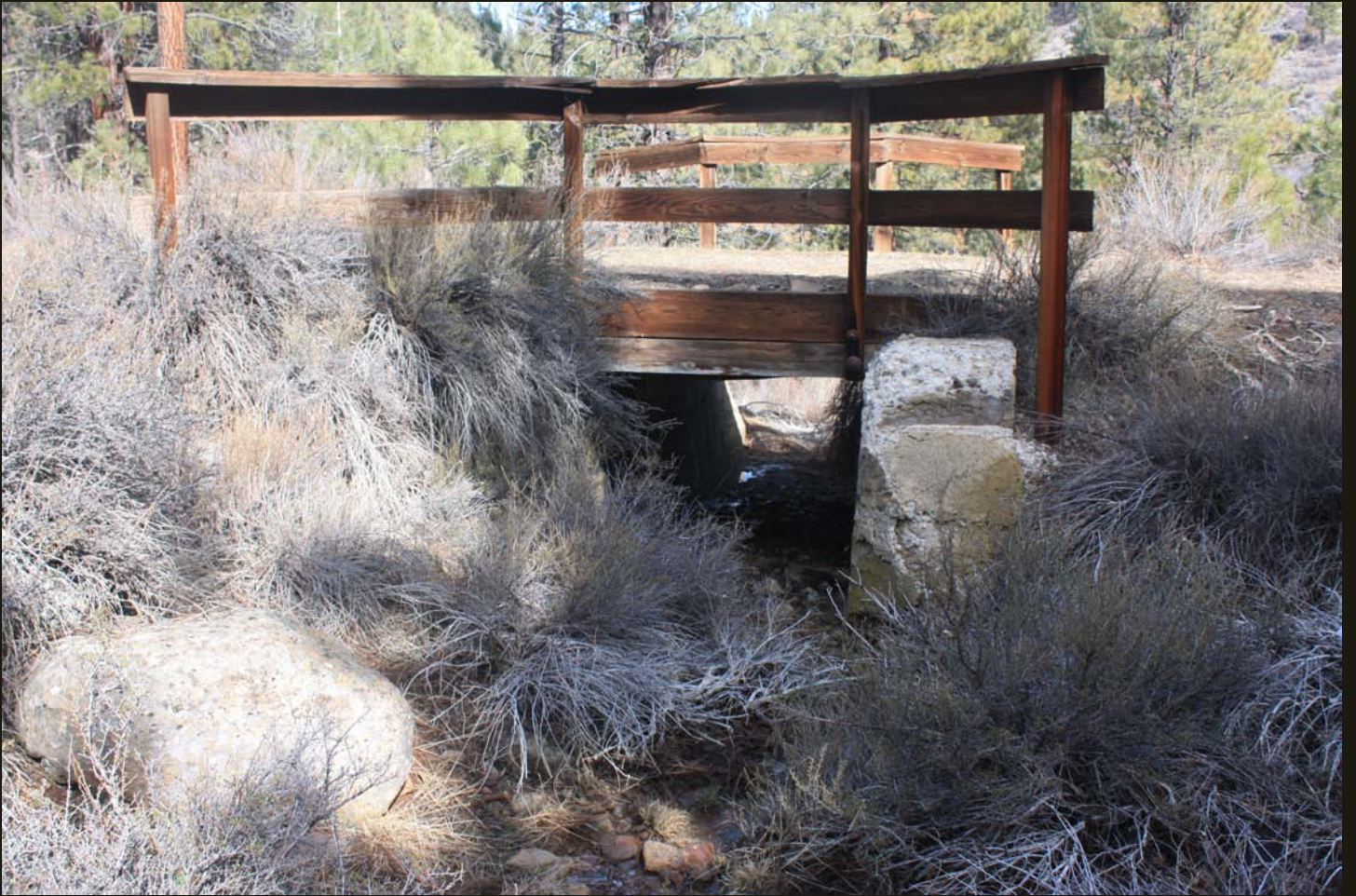
Concrete culvert for F&L.
