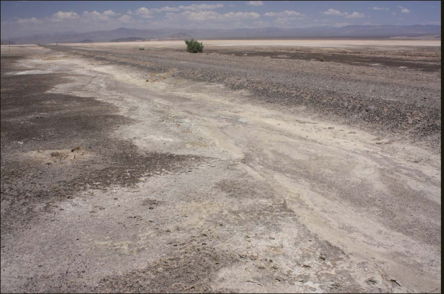
Northward view of the T&T grade just north of Zzyzx. Note the flat Soda Lake, which was a lush perennial lake during the Pleistocene ice ages. Note also that the grade is plenty wide for an automobile; after abandonment, this part of the grade was flattened and widened for auto use.
