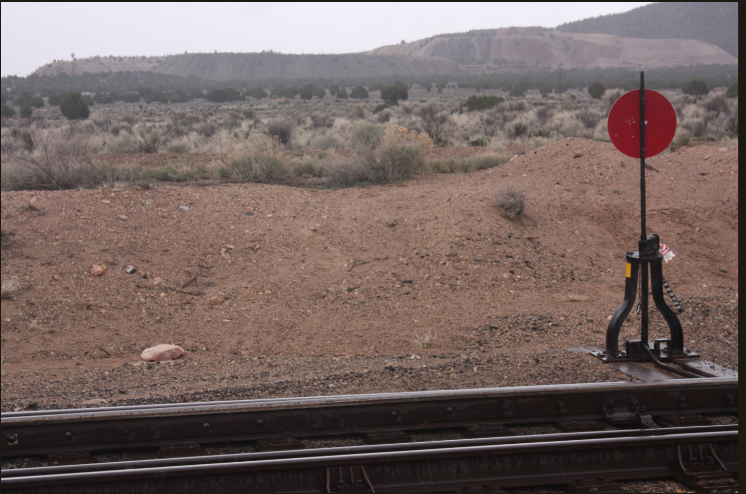
Southward view of the switch for the wye, same location as previous. Mine tailings from the Desert Mound Mine are in the distance.
