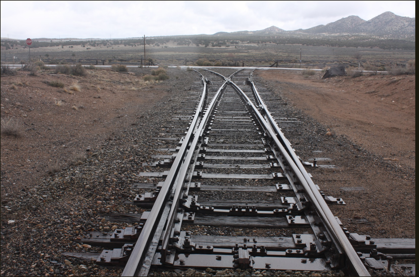
Northeastward view of the wye for the LA&SL Desert Mound Spur (1924). The LA&SL Cedar City Branch (1923) runs across the image in the distance.
