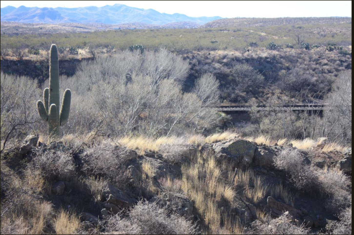
Southward view of the single-track SP Sunset Route (1881) near Pantano, Arizona. The stately saguaro was probably a youth when it oversaw the SP construction crews in 1880. The 9,000+ foot Santa Rita Mountains are in the distance.
