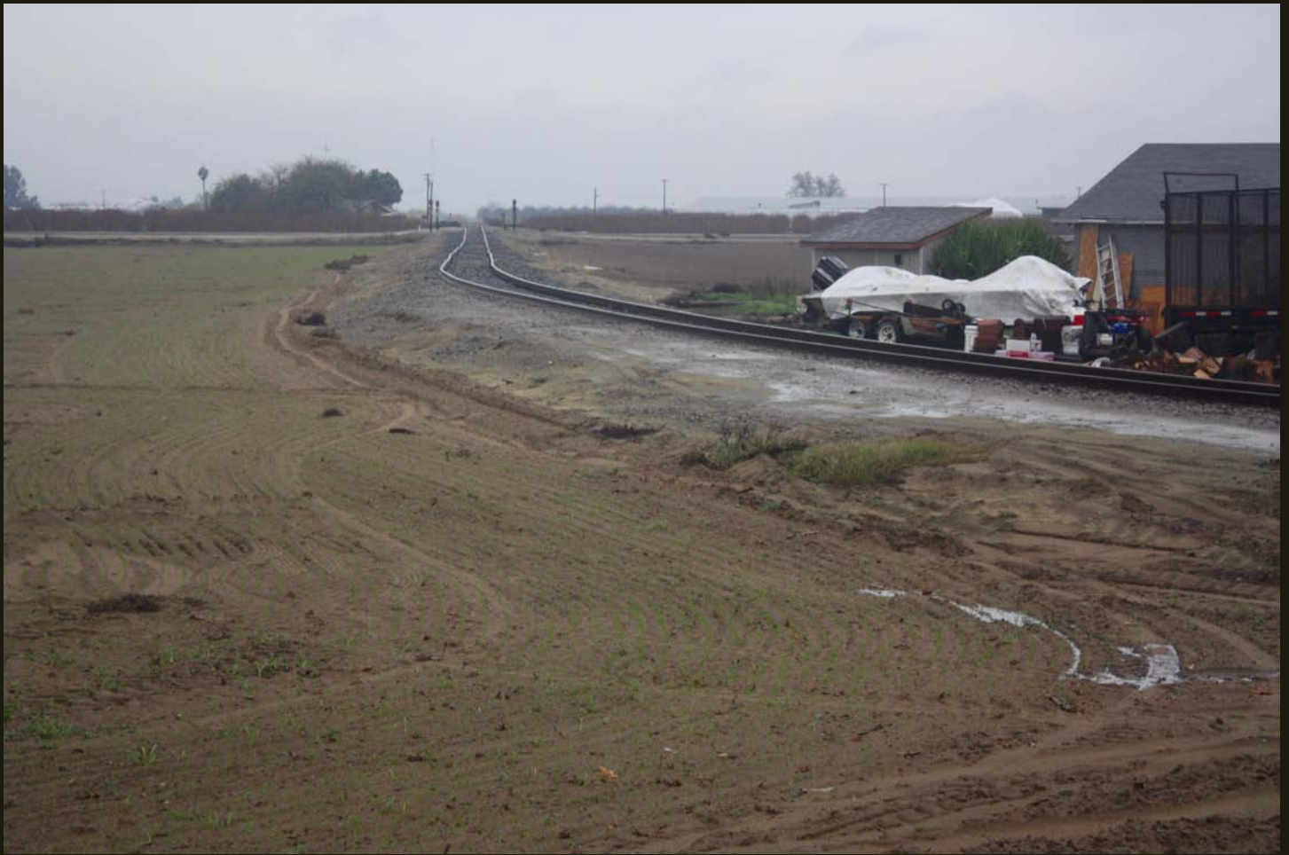
Northwestward view of the TS (1917) Hilmar Branch 2 miles south of Hatch at Chemurgic. The line to Hilmar once extended straight to the viewer but, as can be seen here, all traces of the line to Hilmar are gone; I could find no evidence of the line south of here, either on the ground or in satellite images, all traces of the line having been re-graded for agriculture and residential development around Hilmar. The curve to the right (west) is the spur to the Chemurgic facility.
