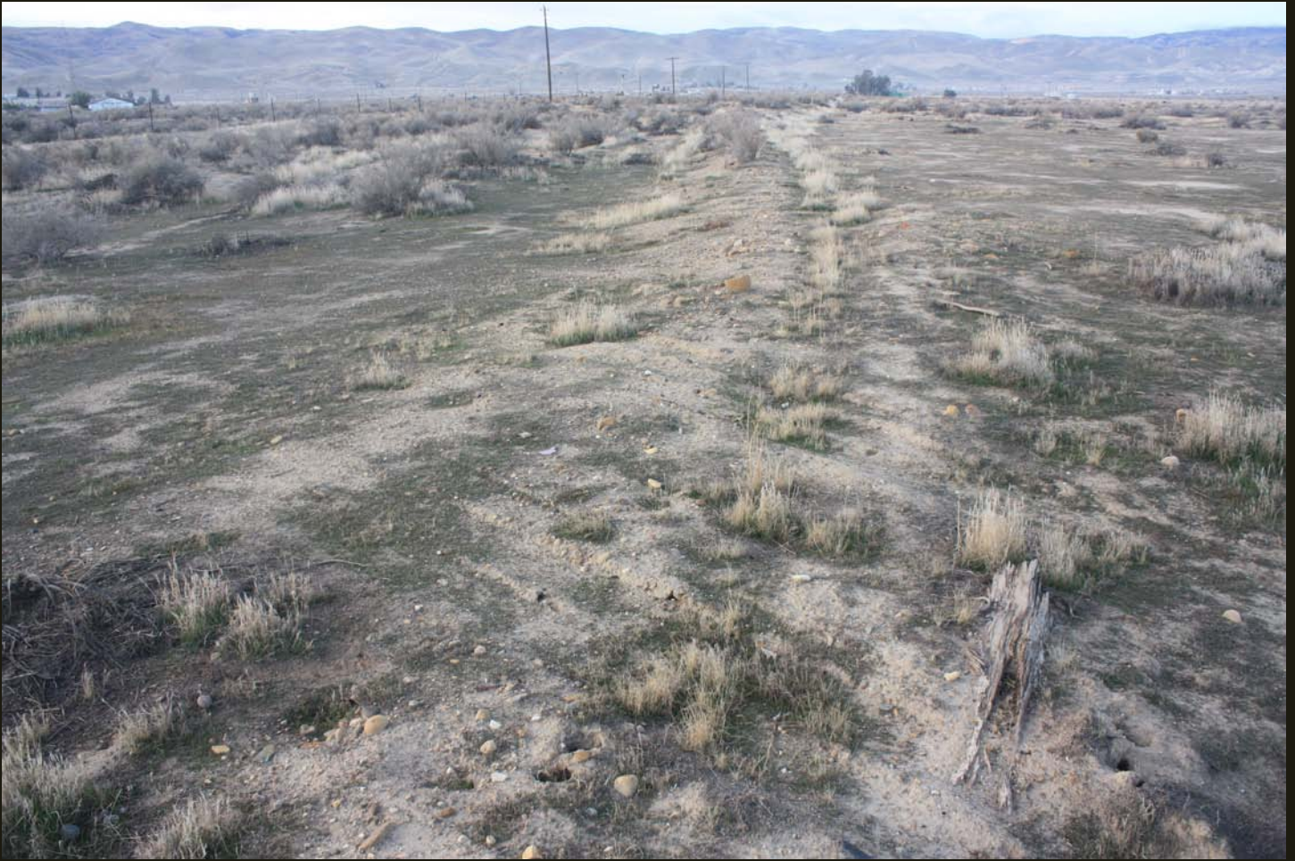
Southwestward view at the same location as previous, showing the original SW grade to Hazelton, built in 1901. Note the rounded cobbles used in the ballast; this ballast is not from the fine-grained native soils at this location and is different from the ballast used later to build the Taft Branch.
