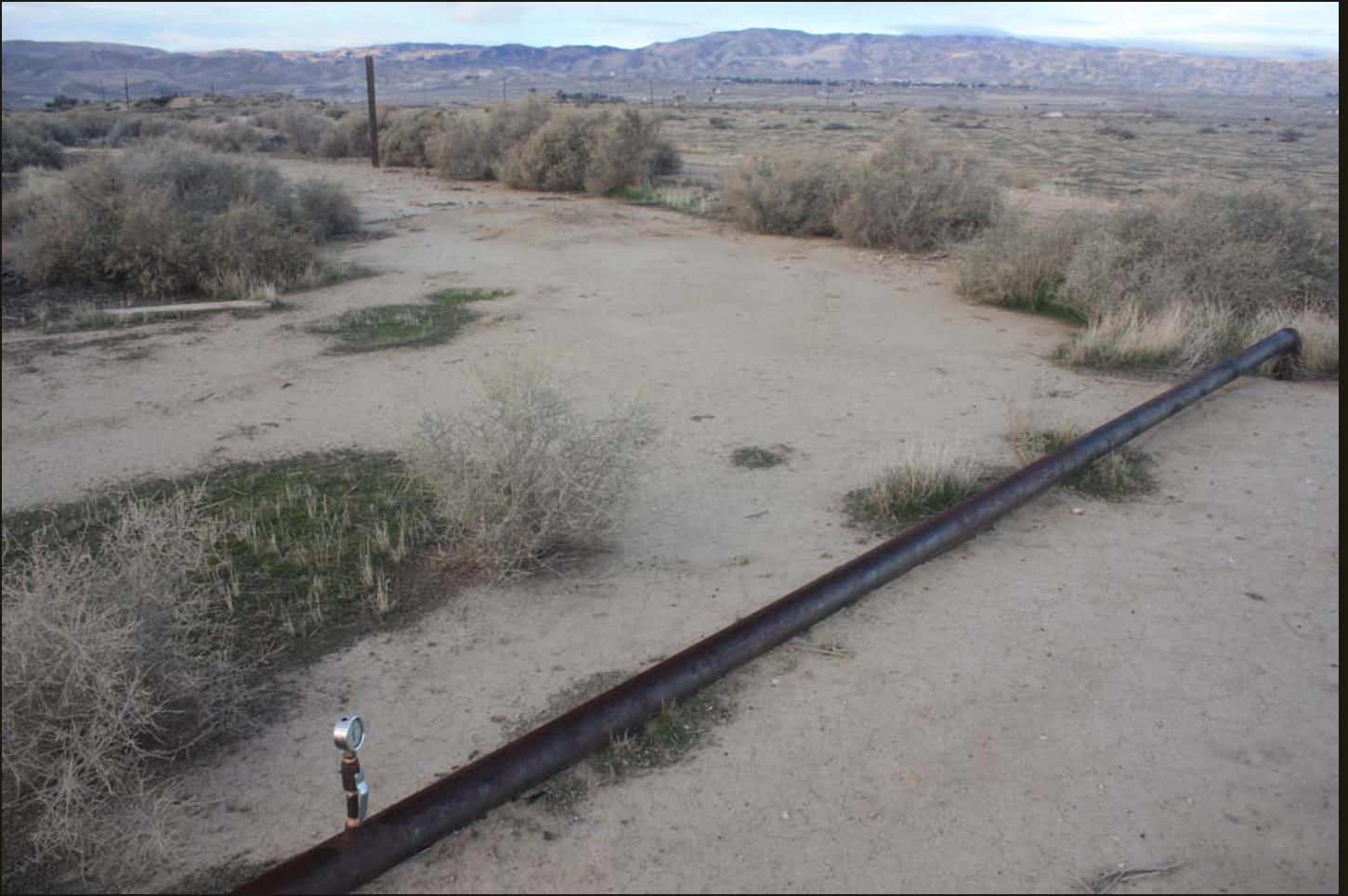
Same location as previous, showing in oilfield-related pipeline and gauge across the SW grade. Note that the pipe goes underground on the right-hand side of the picture. This may have been to go under the still-active Taft wye after abandonment of the SW original grade in the foreground.
