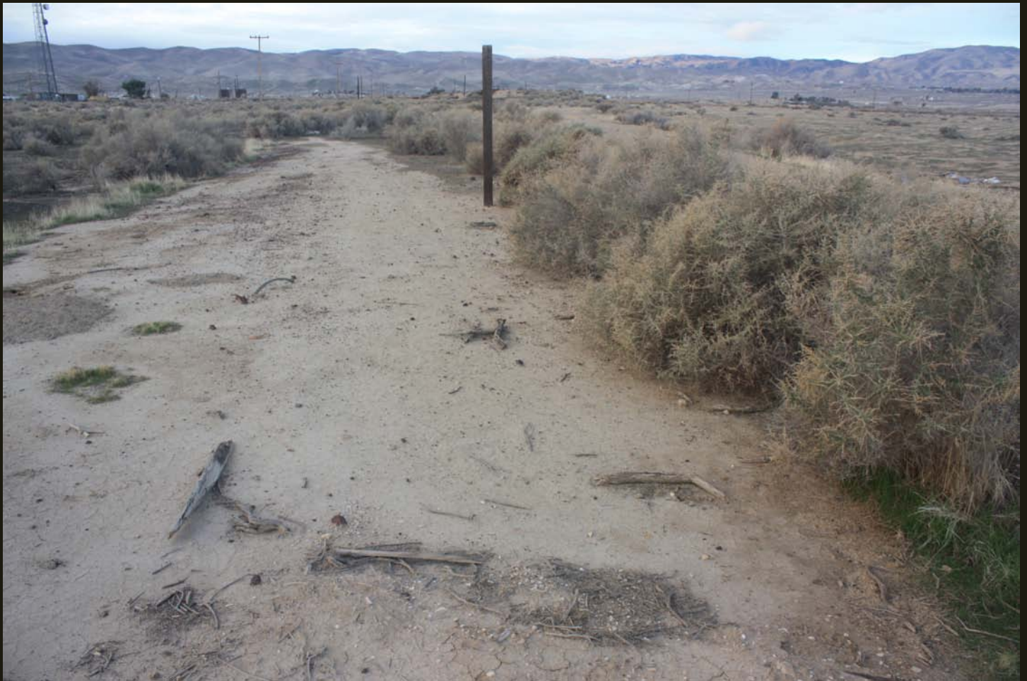
Southwestward view of the original SW grade at Pentland, California, approaching the wye for the Taft Branch. The higher-ground loading facility is behind the post. The grade in the foreground, with splinters of old ties, is the original alignment toward Hazelton; the parallel approach to the Taft wye is to the right (northeast) on the other side of the row of brush. The hills in the distance are the Temblor Range, which bounds the Central Valley to the southwest.
