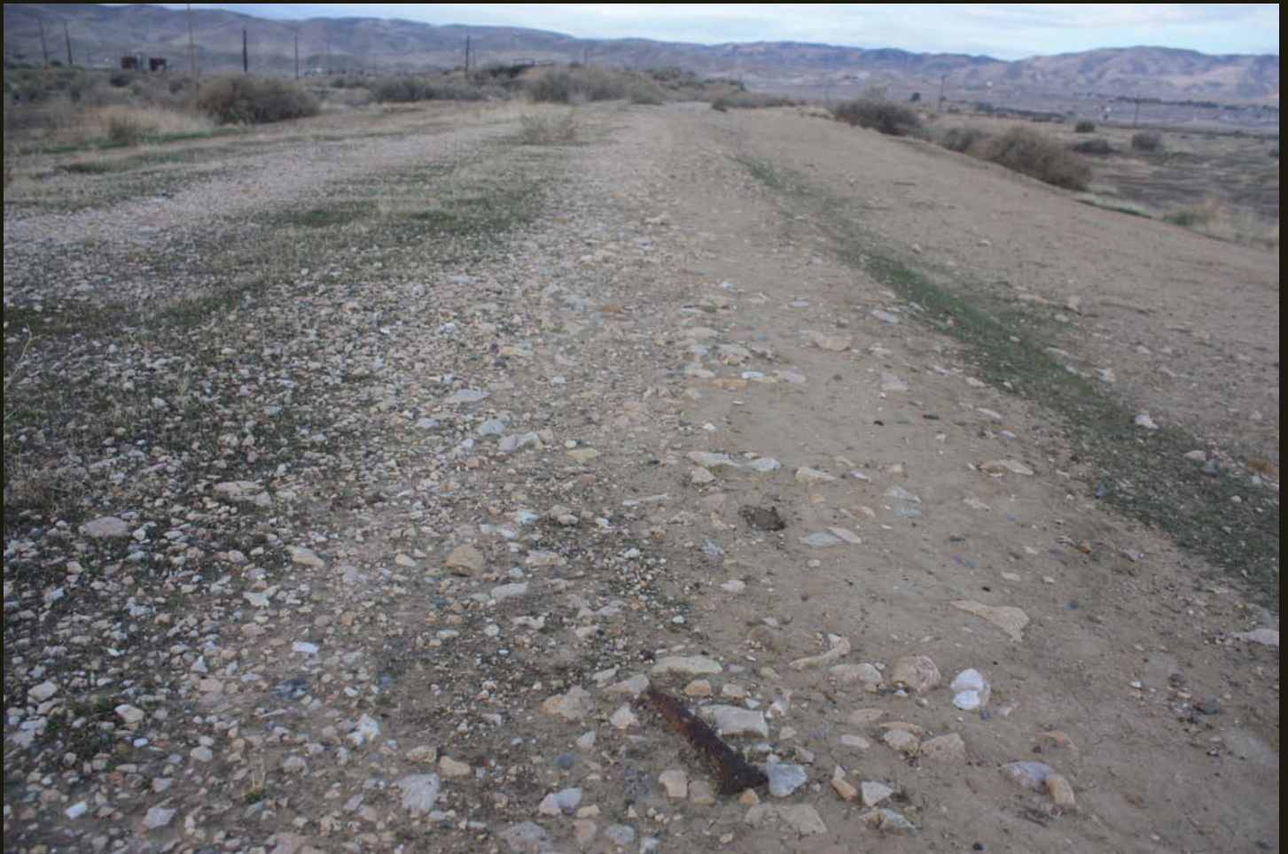
Southwestward view of the original SW grade at Pentland, California, approaching the curve to the right at the beginning of the wye for the Taft Branch. Note the higher ground where the grade curves -- the same loading facility as before -- and the old SW spike left behind in the ballast when the line was salvaged. Note also the flat area with ballast to the left; this is the original alignment toward Hazelton and is parallel to the approach to the Taft wye, which was likely a siding off of the original SW alignment.
