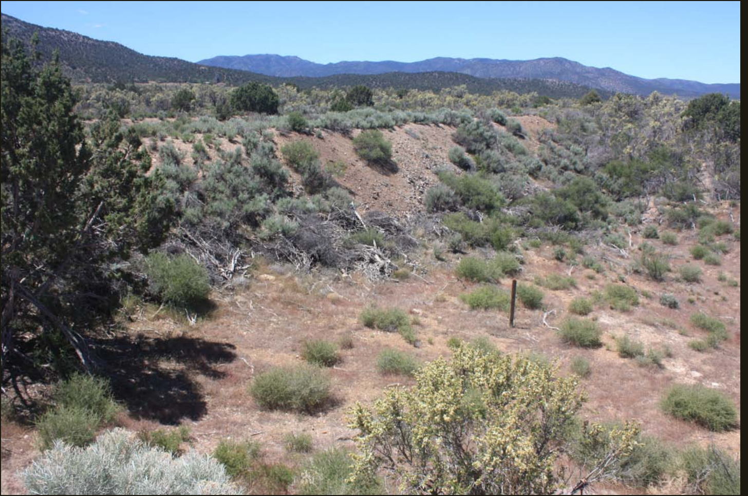
Southwestward view of a significant fill grade for the PC (1912), 200 feet west of previous location.
