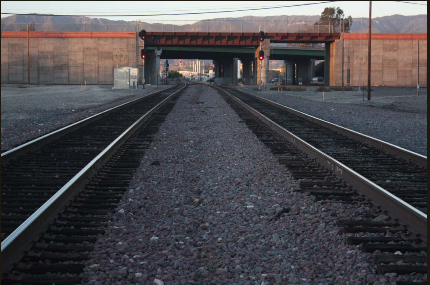
The Colton Crossing flyover project was completed in August 2013 and carries the UP (former SP) grade over the BNSF (former CS) double track. The new Colton Crossing speeds rail traffic for the more than 110 trains that pass here each day each day.
