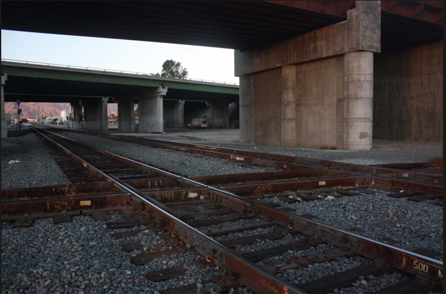
Northward view at same location as previous. The UP (former SP) single track is crossed by the BNSF (former CS) double track. The far overpass is the I-10 Freeway and the near overpass is a new UP grade separation, replacing the old crossing.
