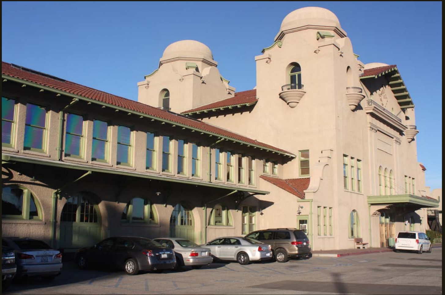
The Santa Fe (AT&SF) Station in San Bernardino is now an Amtrak station and houses some government offices.
