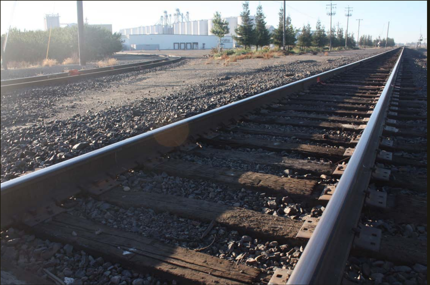
Southward view of the Northern Railway (now California Northern) a mile north of Arbuckle, with a spur to a processing plant for California Family Foods. Note the upgraded welded tracks.
