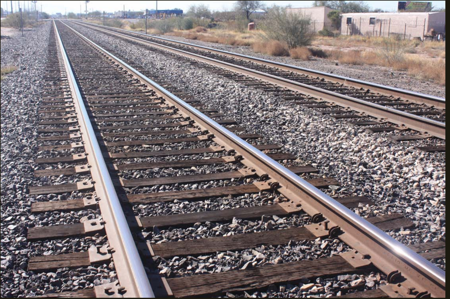
Southeastward view of the SP (1881)-EP&SW (1912) crossover track, probably built around 1952.
