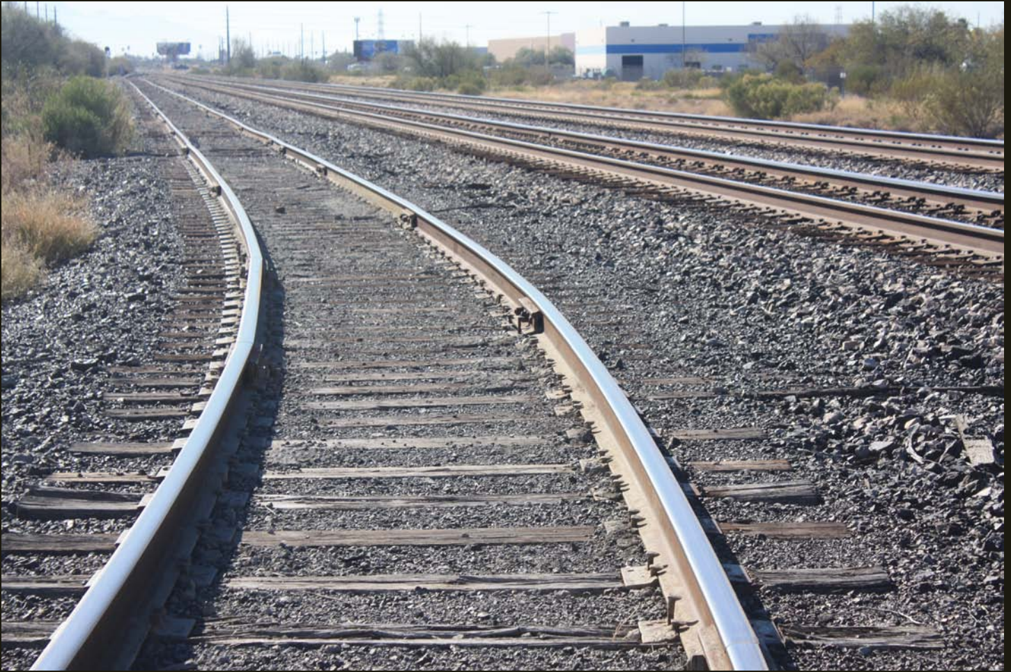
Southeastward view a quarter mile south of the previous location. The SP's 1952(?) crossover between the SP (1881) and EP&SW (1912) alignments is to the right, and an industrial spur is in the foreground and turns east.
