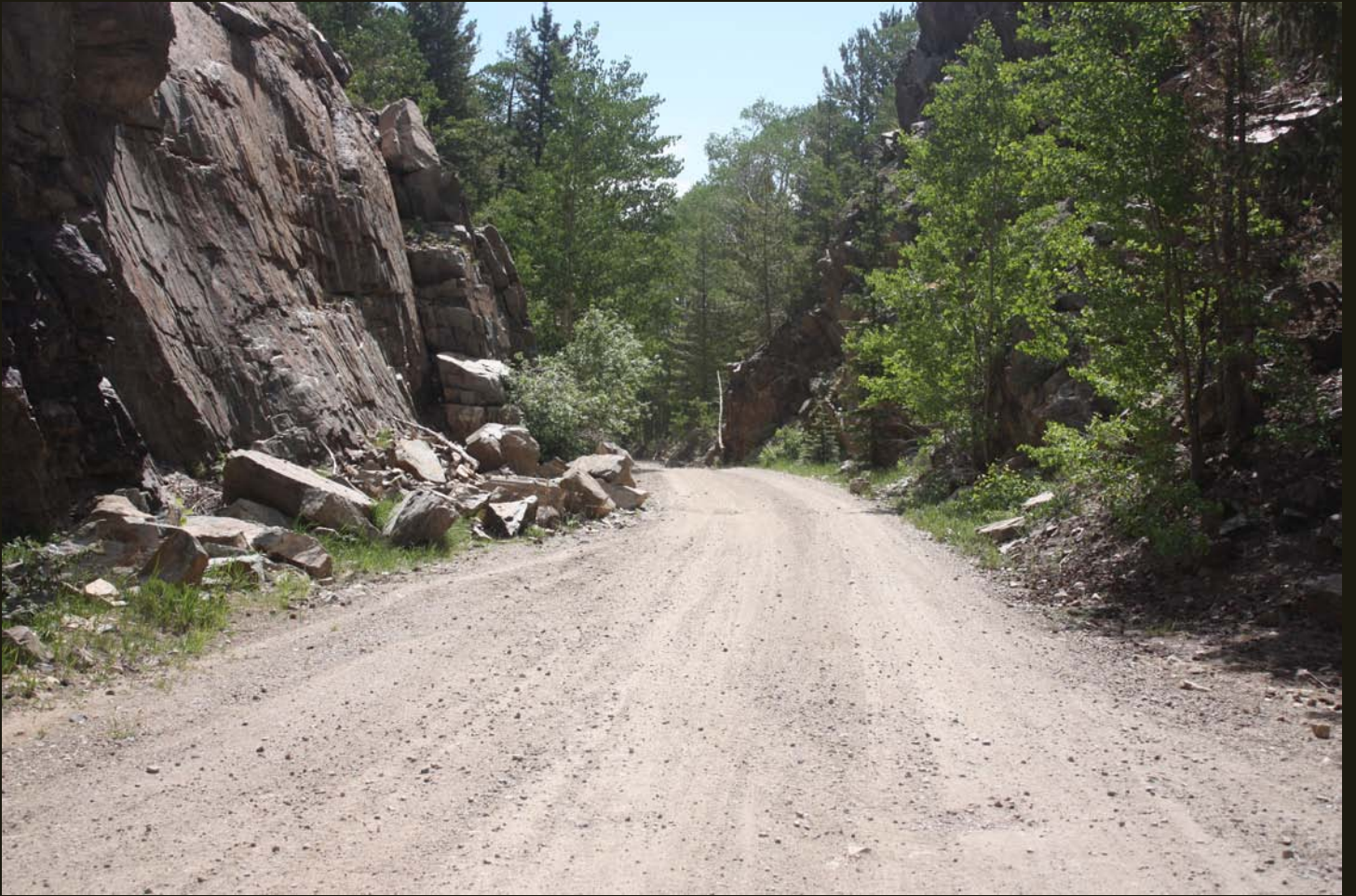
A major cut through rock, 3 miles up-grade from the previous photo.
