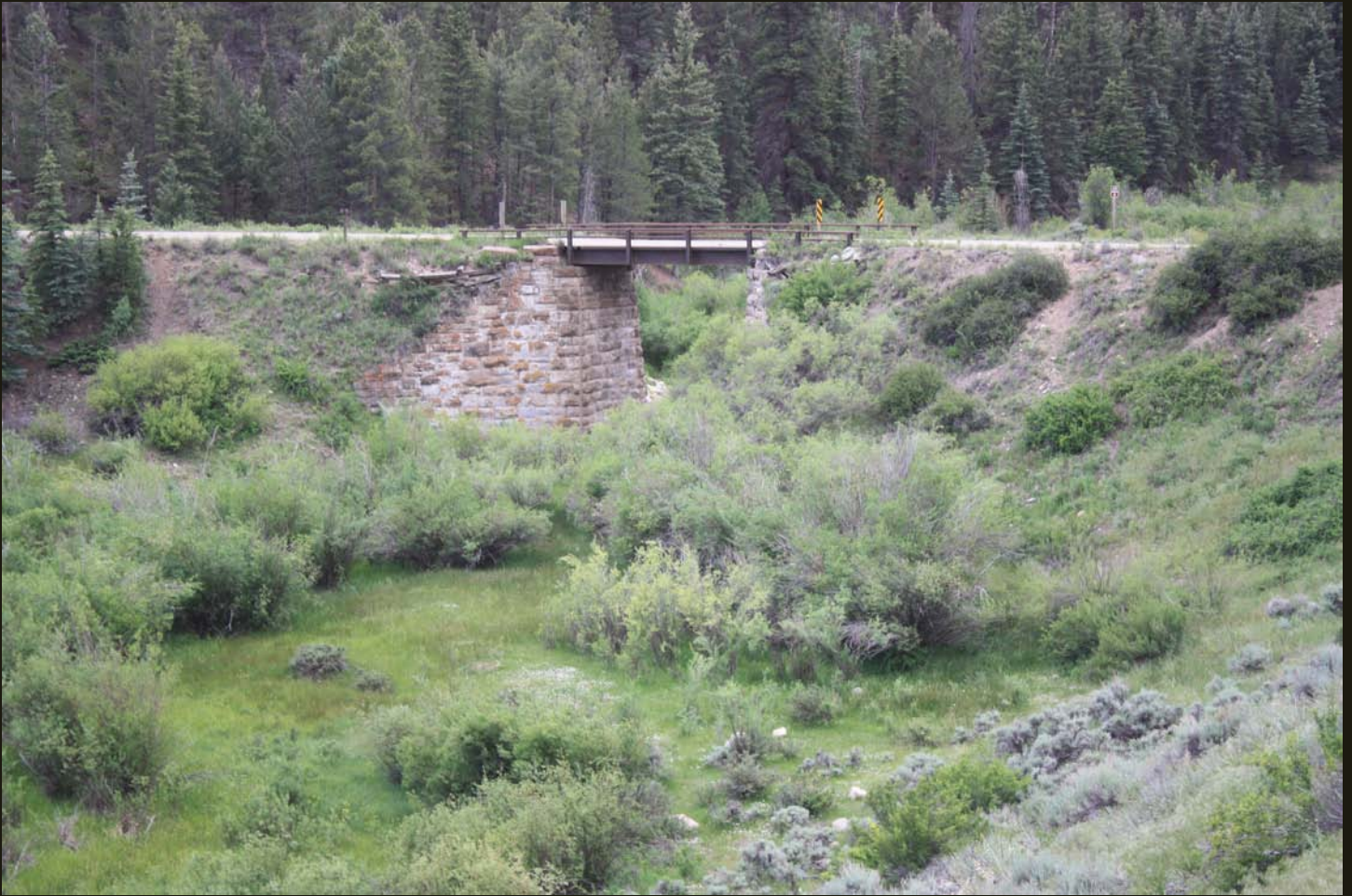
Closer view of the wonderful masonry bridge across Pocha Creek.
