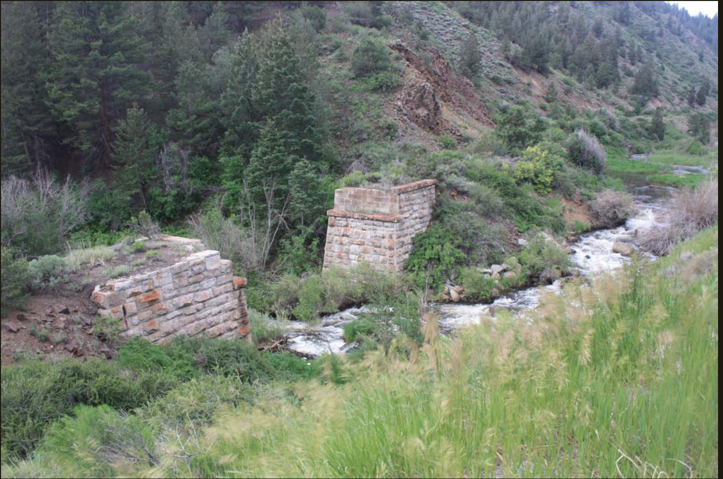
Three miles up the grade from the previous photo, masonry abutments supported a narrow gauge bridge across Poncha Creek. The junction with the D&RG's Chili Line is between this location and the previous photograph but was obliterated by later grading.
