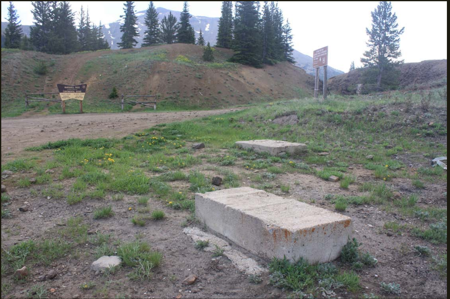
Marshall Pass, Colorado, had a small settlement with a railroad station and "the U.S.'s smallest post office" according to Time Magazine. The population was 11 in 1948 when there were six buildings. These footings at the west end of the summit cut were part of the settlement.
