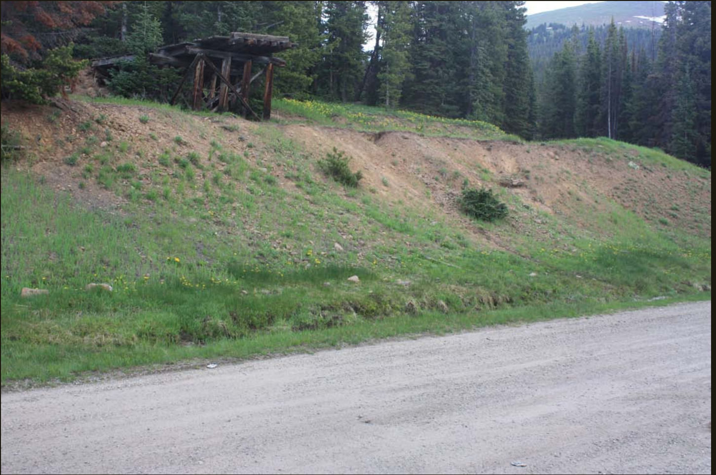
An old loading structure of some sort, a quarter mile east of Marshall Pass. Forest Road 200 on the D&RG grade is in the foreground.
