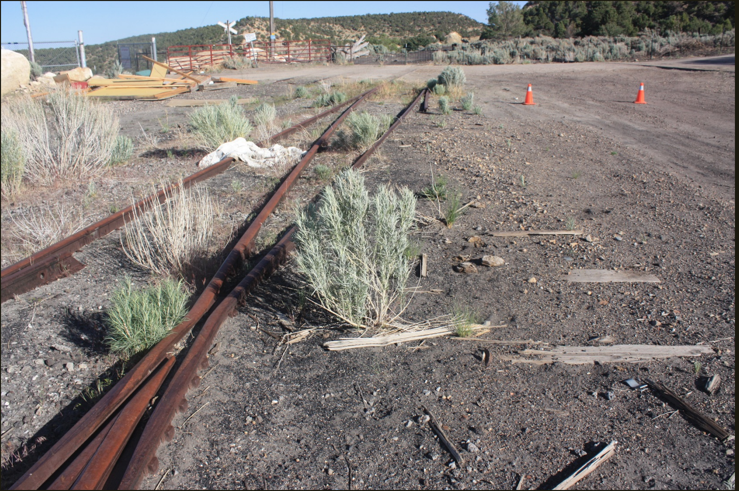
Southeastward view of the Utah Railway (1917) at Hiawatha, 100 feet north of the previous location. The same crossing of Utah "Highway" 122 is just beyond the traffic cones. There are three tracks that cross the road in this view, from left to right: cut siding, the mainline (which extends to the foreground), and the lower spur (above the cone in the upper right corner of the photo). The crossing of the upper spur is just out of sight on the right. The mainline in the foreground has a switch and some ties still in place for an otherwise removed siding.
