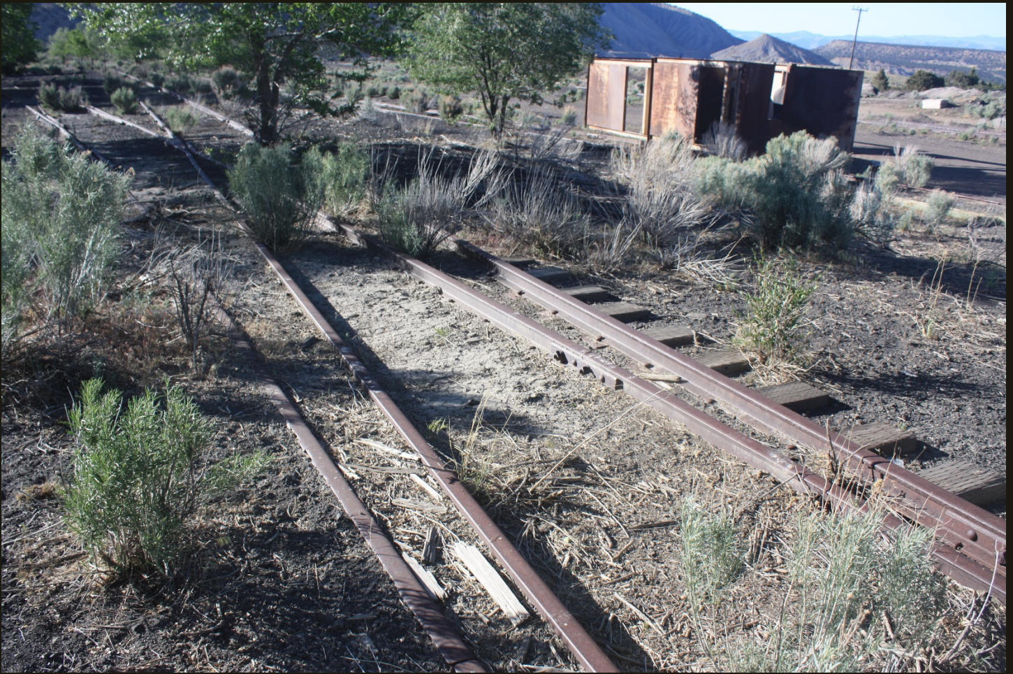
Northward view of the higher of the two spurs of the Utah Railway (1917) at Hiawatha, 40 feet west of the previous location and the lower spur. The lower spur is just visible in front of the discarded steel frame (referenced in the previous photo). In the foreground, the upper spur splits off a siding so now three tracks are heading to the Hiawatha town and mine.
