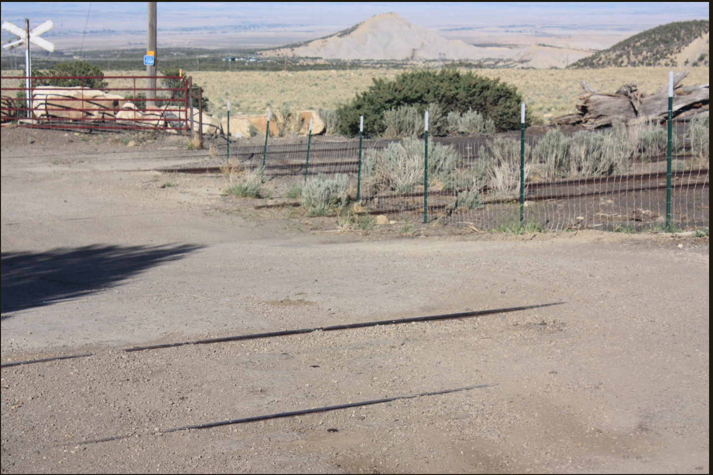
Eastward view of the Utah Railway (1917) 100 feet west of the previous location, where the tracks cross Utah "Highway" 122. There are four tracks that cross the road, from nearest to farthest: the upper spur (hidden by sagebrush in the previous photos), the lower spur, the mainline, and the cut siding (in foreground of previous photo).
