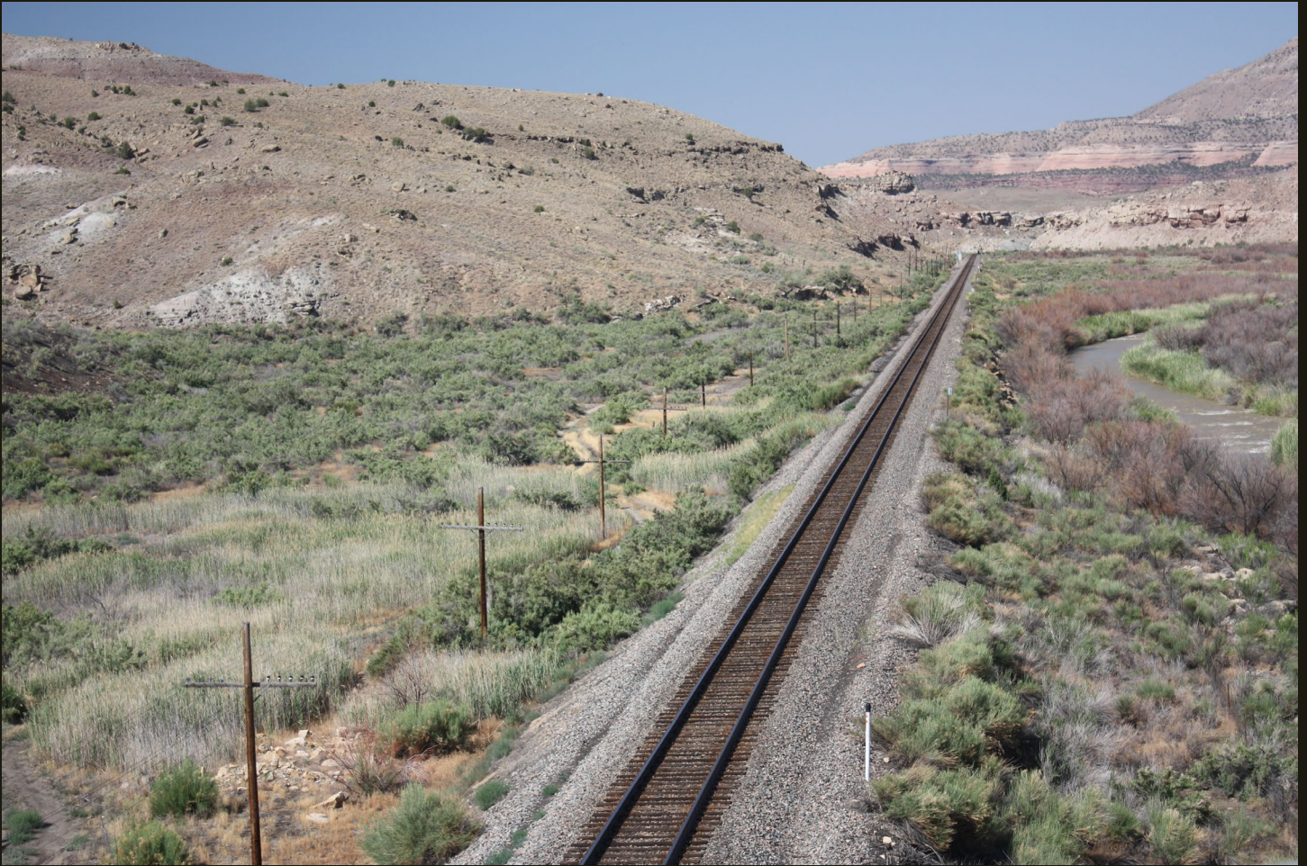
Southwestward view of the D&RGW (1890) from the I-70 overpass 1 mile west of the previous location, where the line follows Salt Creek to its confluence with the Colorado River 2 miles down the line.
