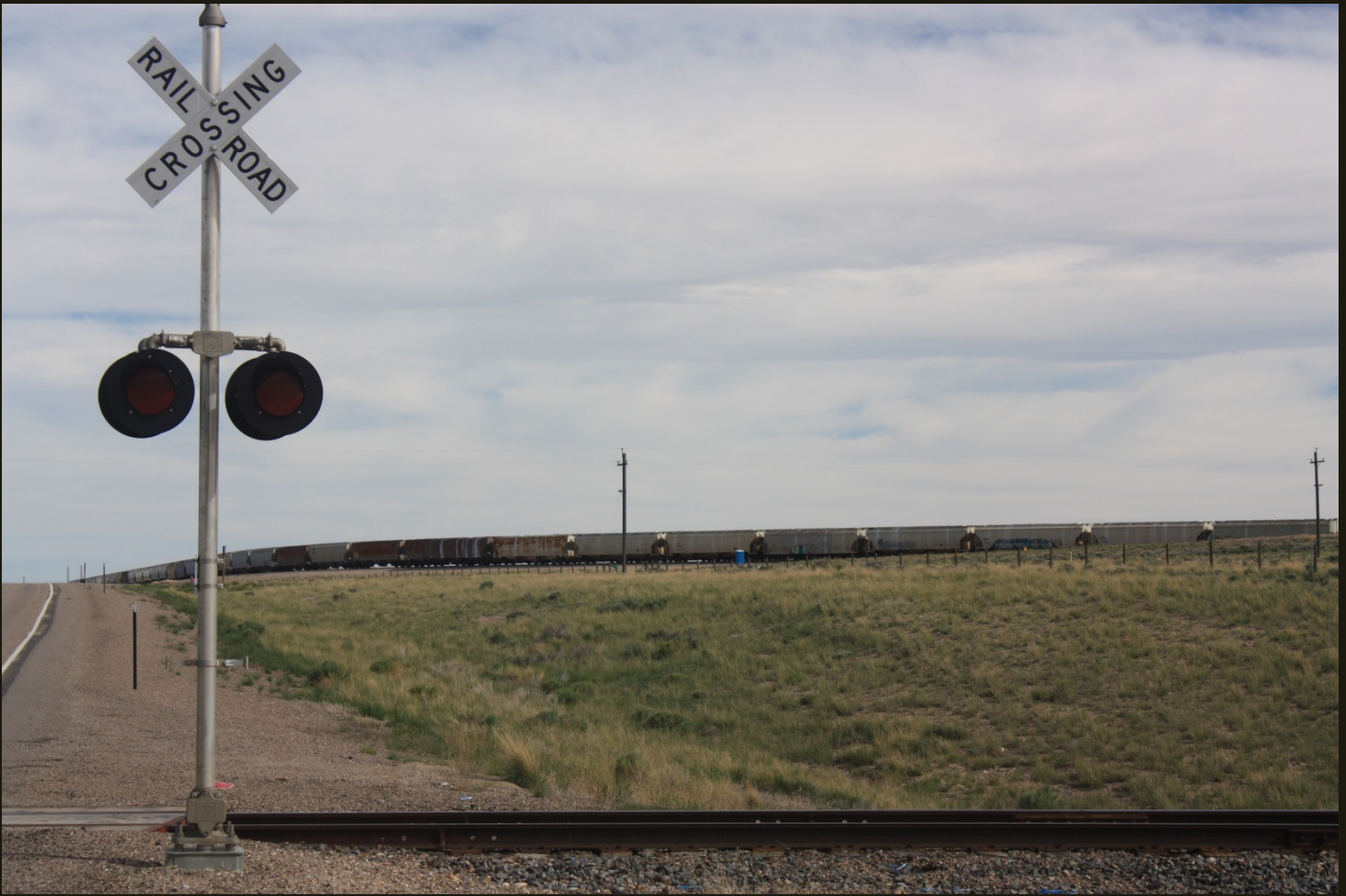
Southward view of the UP Stauffer Branch (c1962), in the foreground, same location as previous. The paved road on the far left is Wyoming Highway 372. The ore cars are on a car storage spur, which switches to the UP Stauffer Branch (c1962) 4,000 feet southwest (to the right) of this location. From that switch, the spur runs northeast, makes a 90-degree turn (seen in this photo) to a southeast alignment, and then ends after a total length of 2.5 rail miles.
