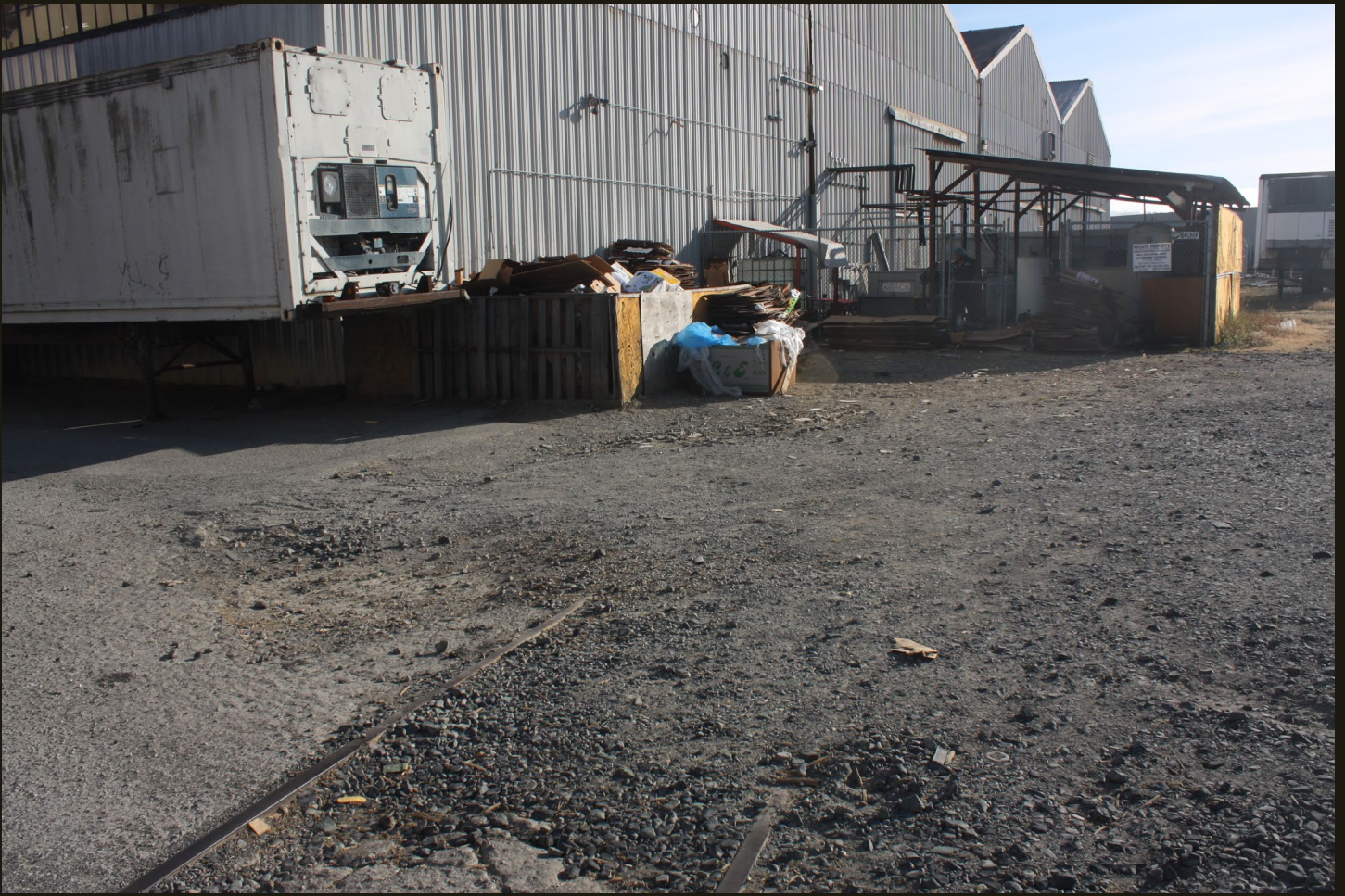
Remnants of track that only hint at the network of spurs that once served industries in South San Francisco.
