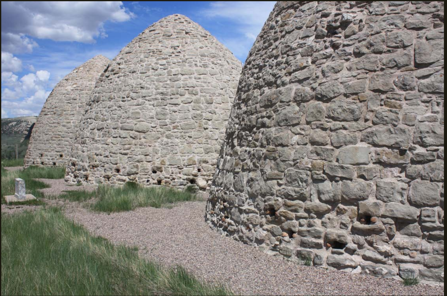
In 1877, Moses Byrne constructed five charcoal kilns in Piedmont, of which three survive and are listed on the National Register of Historic Places. Quaking aspen and pine logs were hauled by ox teams to the kilns where they were burned into charcoal. The UP used the charcoal as fuel for the passenger cars.
