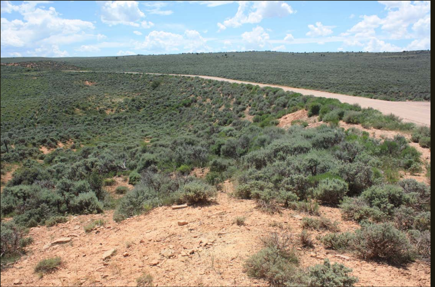
A substantial fill grade on the abandoned 1868 UP route over Aspen summit, where the grade is used by modern Piedmont Road.
